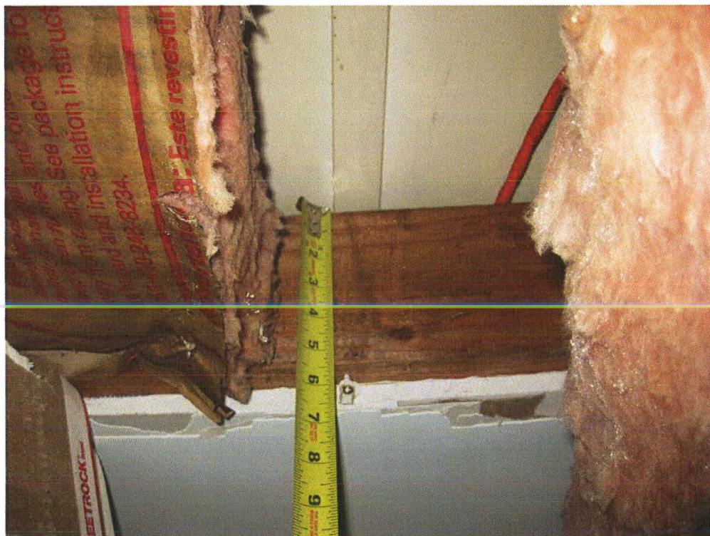
Photo #14 – Ceiling joists at kitchen
