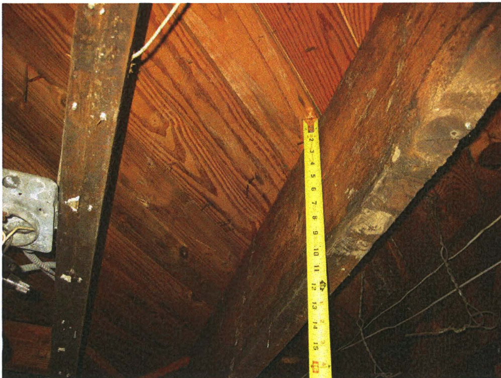
Photo #16 – Second floor framing above mechanical space
