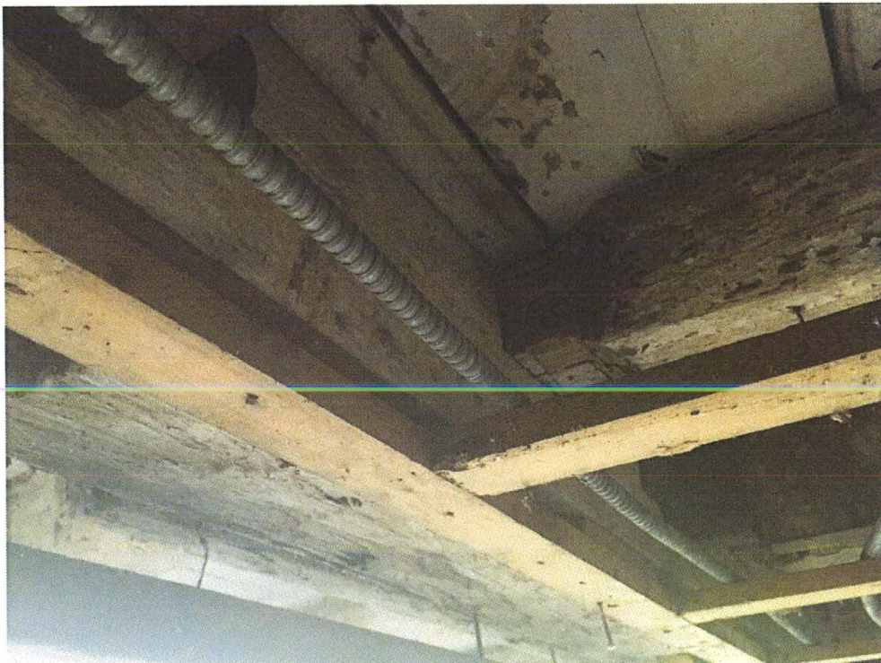
Photo #6 – Bearing at joists on ledger mounted to perimeter girder
