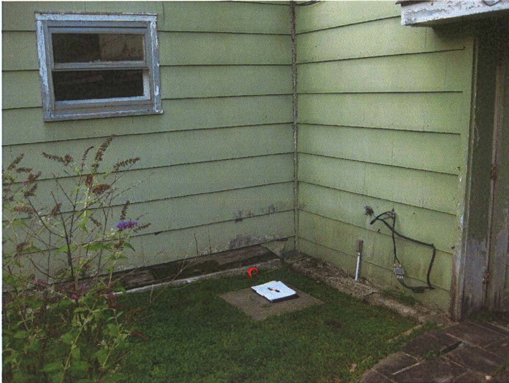
Photo #15 – Support of first floor and foundations at kitchen
