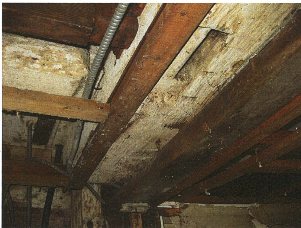
Photo #4 – Second floor framing at original building with mortise at bottom of girder
