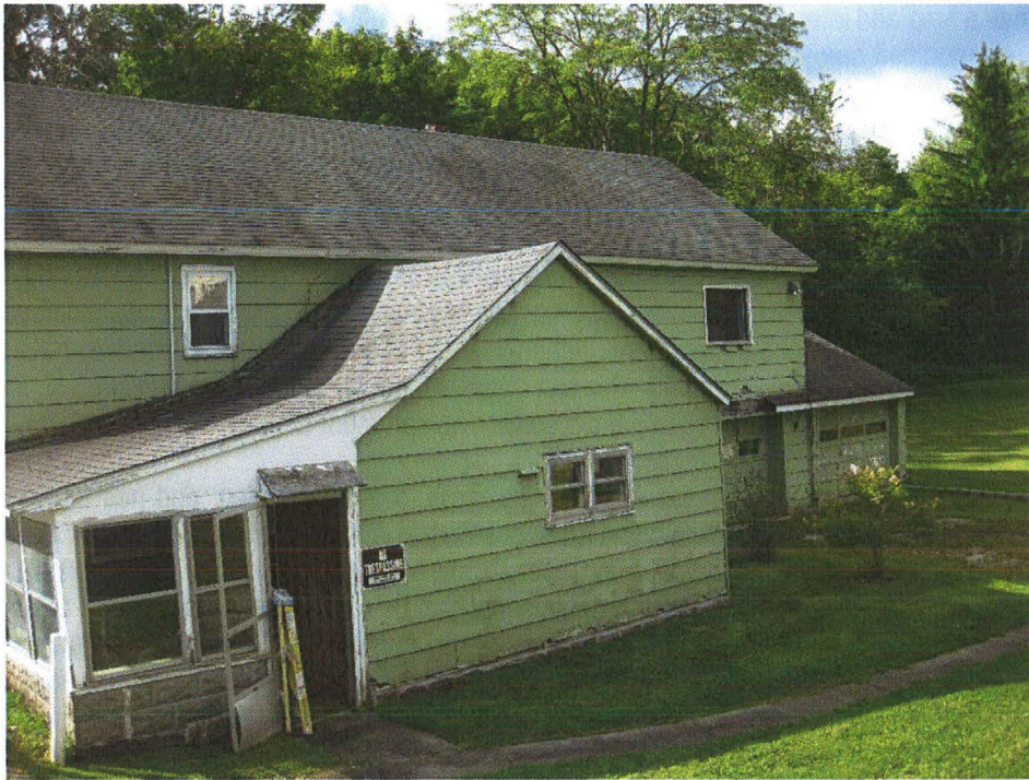
Photo #1 – Roof forms at north side
