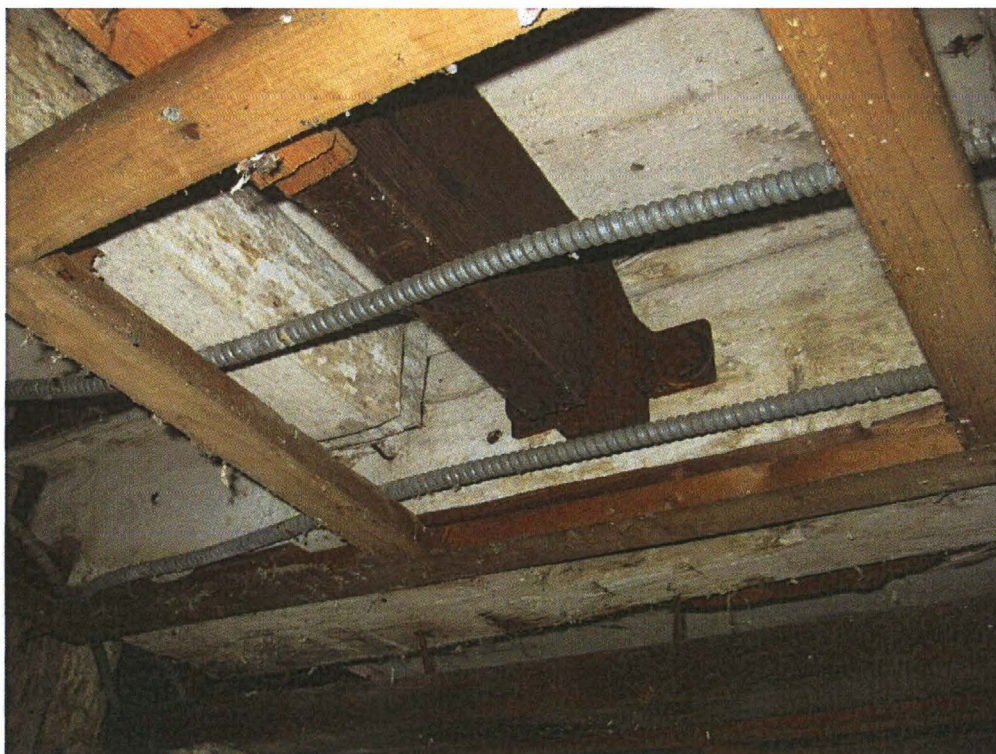
Photo #8 – Sister joists at second floor
