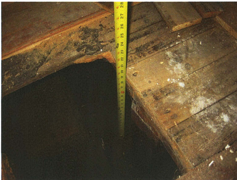
Photo #11 – Supported first floor and mud slab
