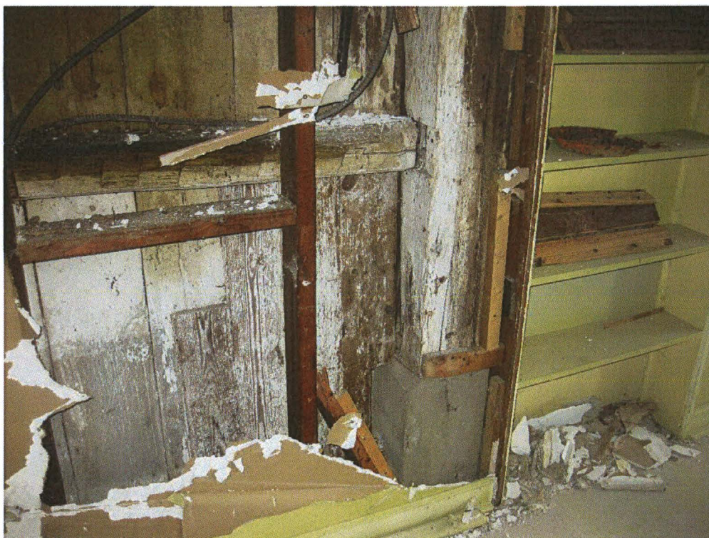
Photo #12 – Concrete pier at base of post
