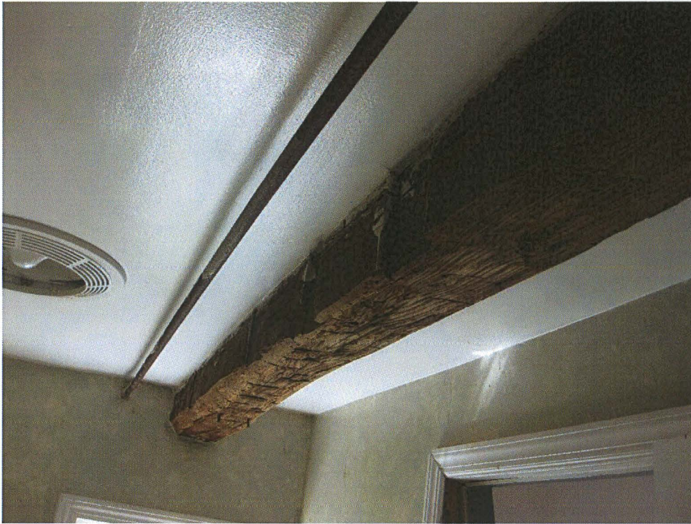
Photo #19 – Reclaimed ceiling girder and tie rod at second floor
