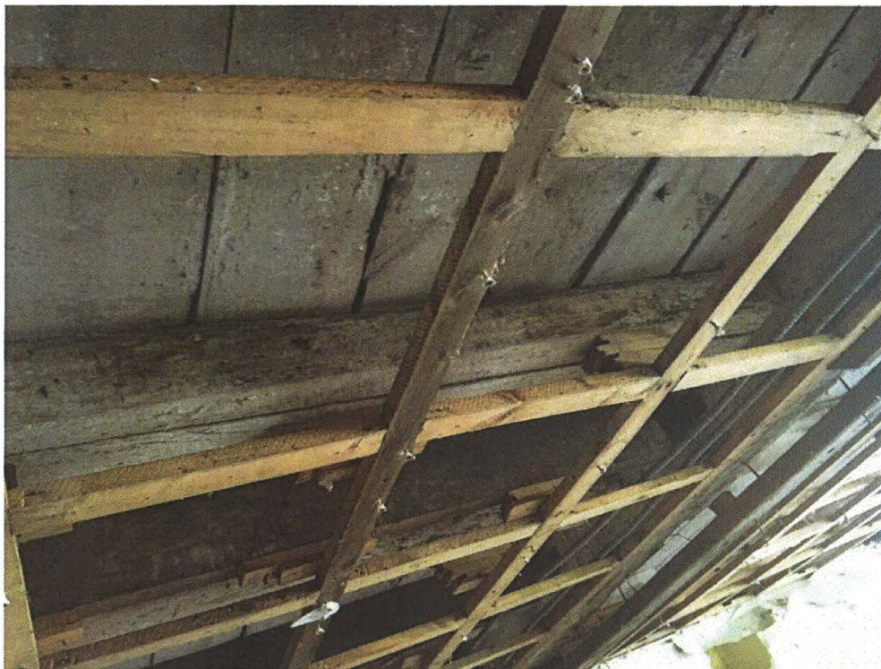
Photo #3 – Second floor framing at original building
