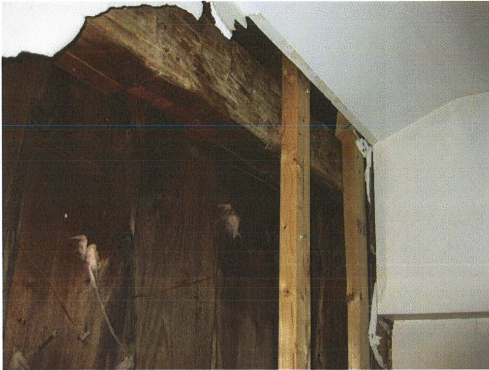
Photo #9 – Original wall framing
