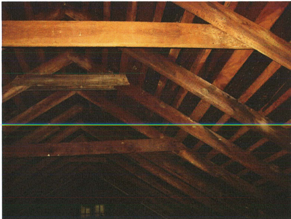
Photo #10 – Roof framing at main gable
