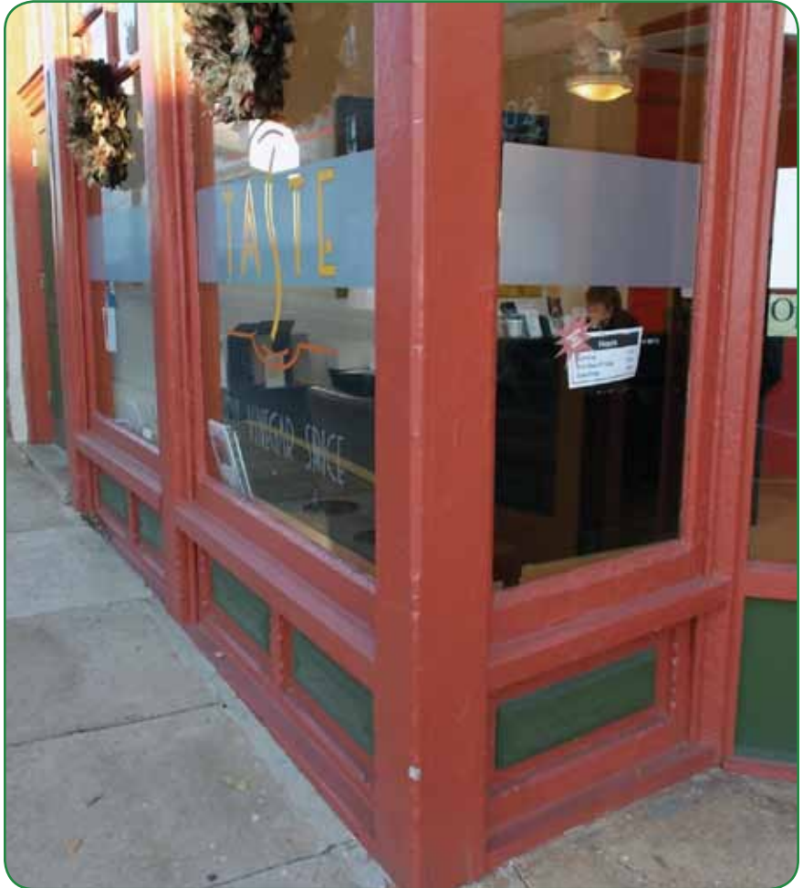
EXAMPLE OF APPROPRIATE TREATMENT: WELL-MAINTAINED FRAMING MEMBERS AND BULKHEADS
