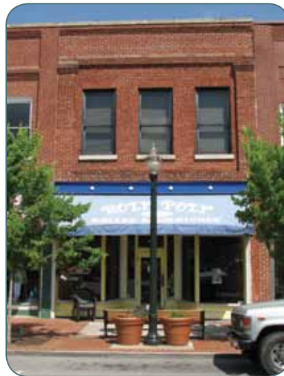
A local example of a one-part commercial block at 104 Washington Street.
