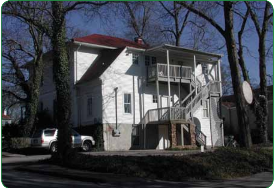
COMPATIBLE AND APPROPRIATELY LOCATED FIRE ESCAPE ON REAR ELEVATION
