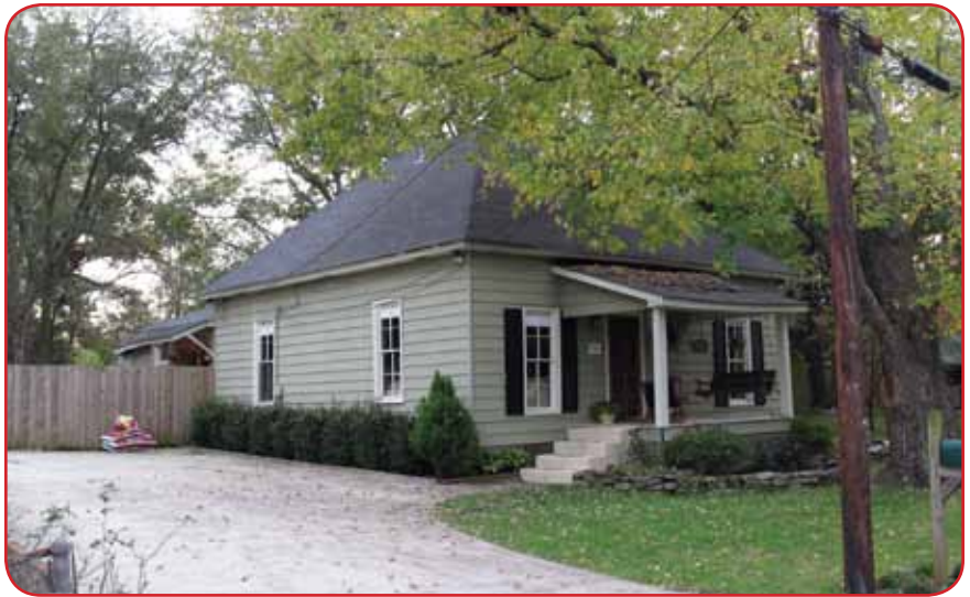
INAPPROPRIATELY LARGE CONCRETE DRIVEWAY
