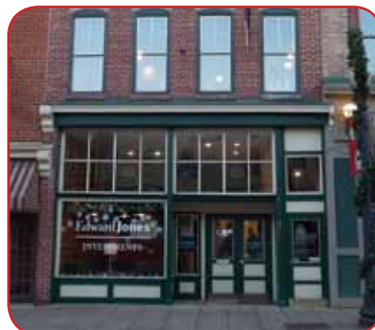
EXAMPLE OF INAPPROPRIATE TREATMENT: ALTERED AND ENLARGED TRANSOMS
