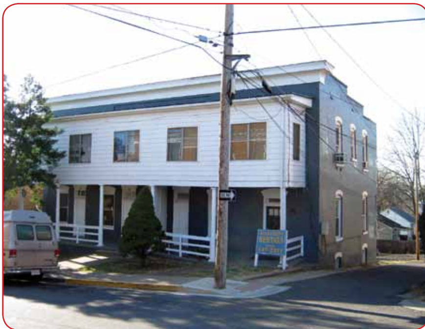
EXAMPLE OF INAPPROPRIATE TREATMENT: ADDITION WITH INCOMPATIBLE MATERIALS
