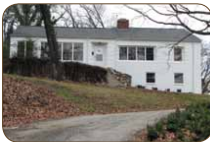
1185 Green Street Circle is a local example with elements of the Art Moderne style.
