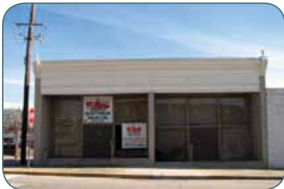
A local example of a one-part commercial block at 851 Main Street, SW.
