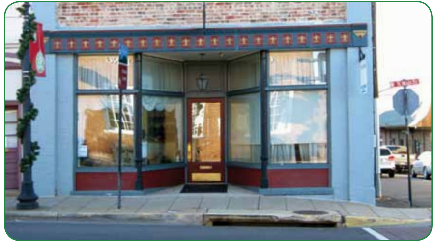
EXAMPLE OF INAPPROPRIATE TREATMENT: ENCLOSED TRANSOM WINDOWS
