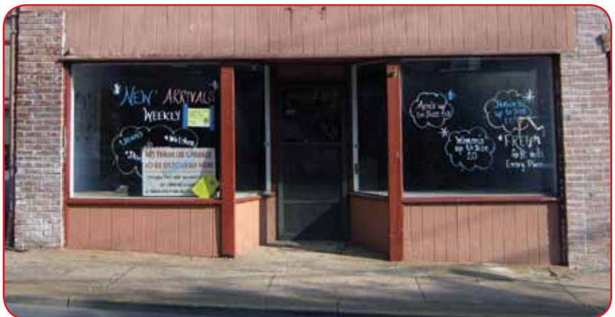
EXAMPLE OF INAPPROPRIATE TREATMENT: ALTERATION TO FRAMING MEMBERS AND BULKHEADS
