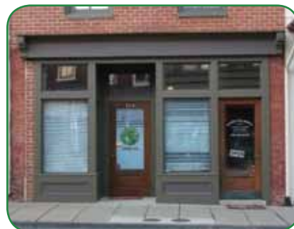
EXAMPLE OF WELL-MAINTAINED HISTORIC DOORS
