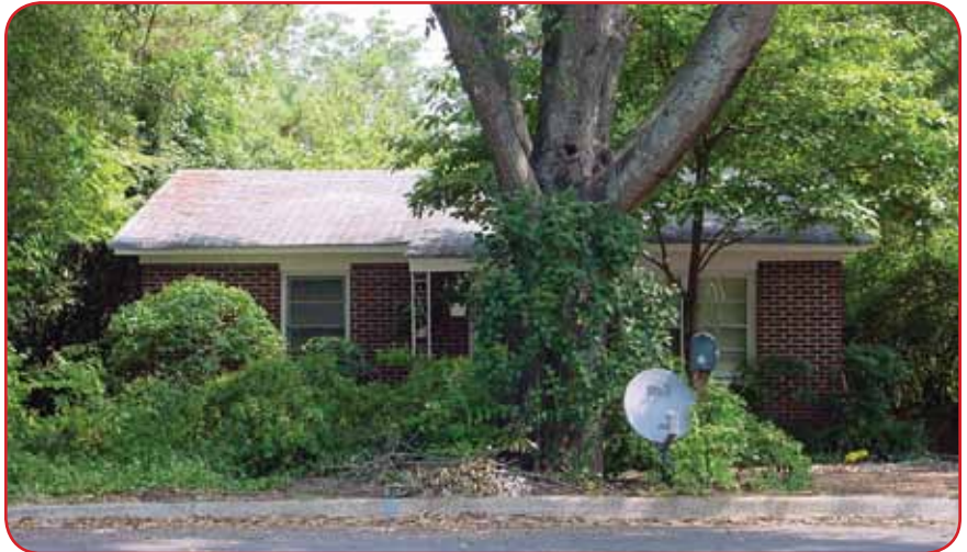
INAPPROPRIATE TREATMENT: SATELLITE DISH NOT SCREENED FROM PUBLIC RIGHT-OF-WAY
