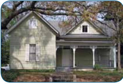
A local example of Folk Victorian architecture located at 500 Ridgewood Avenue.
