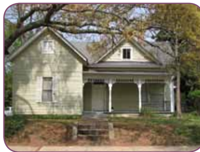
Folk Victorian style residential building located at 500 Ridgewood Avenue is an example of a gabled ell cottage.
