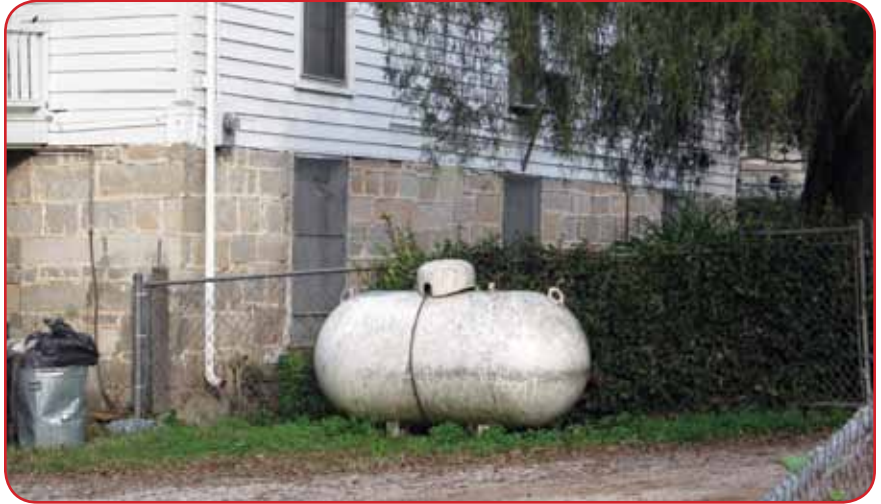
INAPPROPRIATE TREATMENT: UNSCREENED UTILITY
