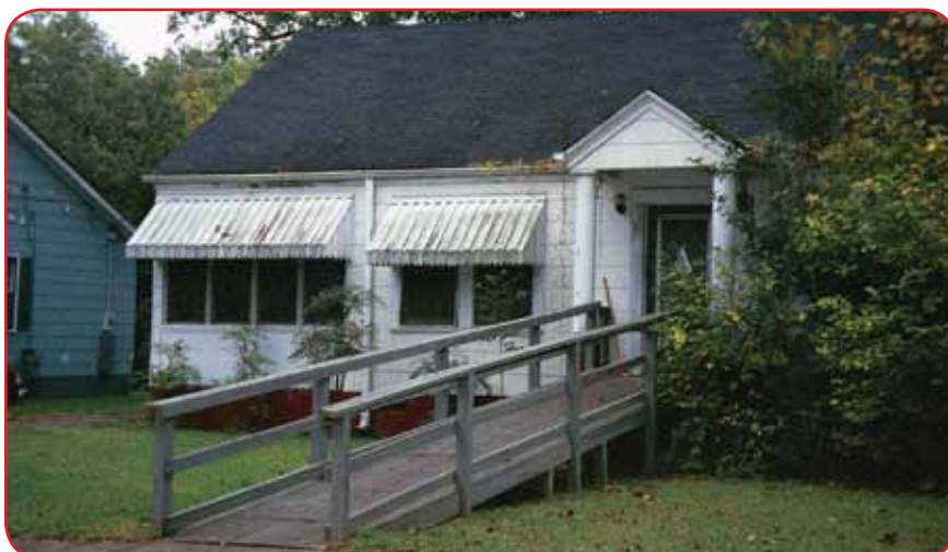
INAPPROPRIATELY LOCATED ACCESSIBILITY RAMP ON PRIMARY FACADE
