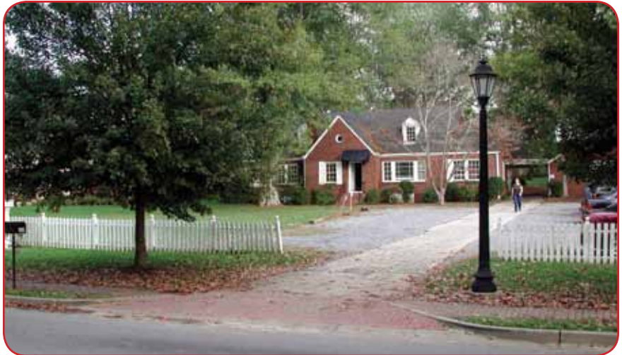
INAPPROPRIATE VEHICLE PARKING AREA IN FRONT OF PRIMARY BUILDING
