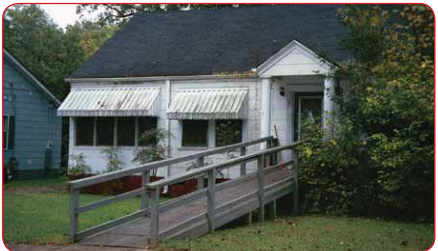
INAPPROPRIATELY LOCATED ACCESSIBILITY RAMP ON PRIMARY FACADE
