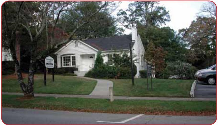
INAPPROPRIATE VEHICLE PARKING AREA LOCATED FOREWARD OF PRIMARY FACADE AND NOT SCREENED
