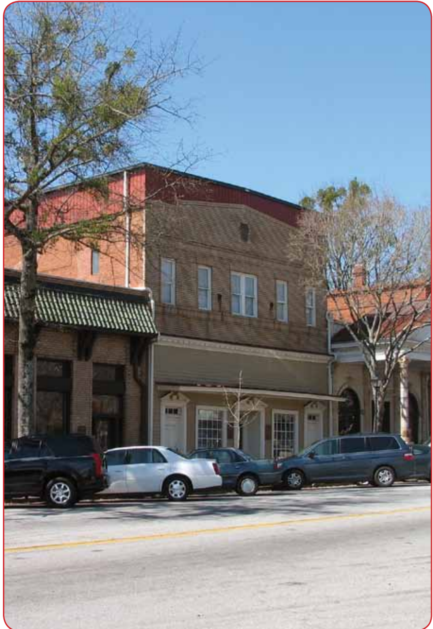
EXAMPLE OF INAPPROPRIATE TREATMENT: ROOFTOP ADDITION VISIBLE FROM PUBLIC RIGHT-OF-WAY
