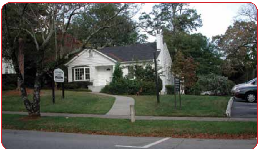
INAPPROPRIATE VEHICLE PARKING AREA LOCATED FORWARD OF PRIMARY FACADE AND NOT SCREENED
