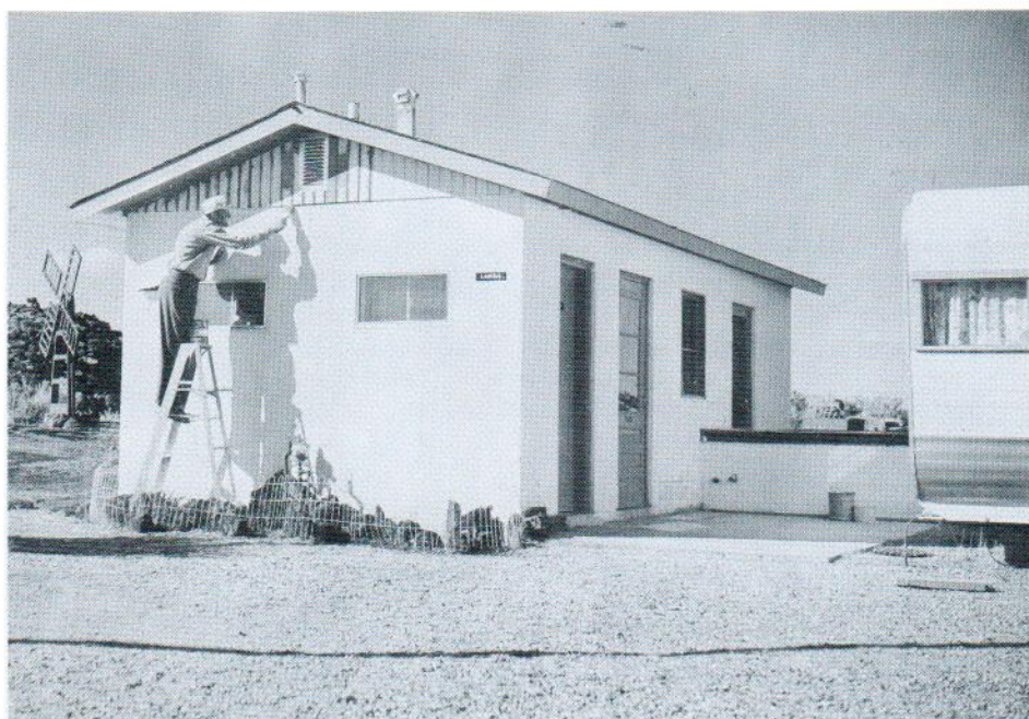
A utility building houses the Onan electric generating set. Exhaust from the unit is piped out the rear of the building. Aluminum louvers directly behind the unit permit ventilation. Pressure tanks for the water system are located in the central portion of the building and the front end houses public restrooms.
