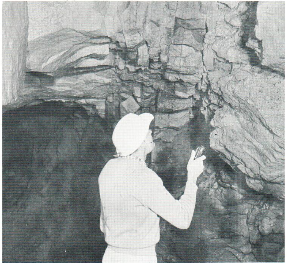
Papadakis, shown inspecting a six foot-wide dike, blasted for two years to complete the tunnel to the cave.
