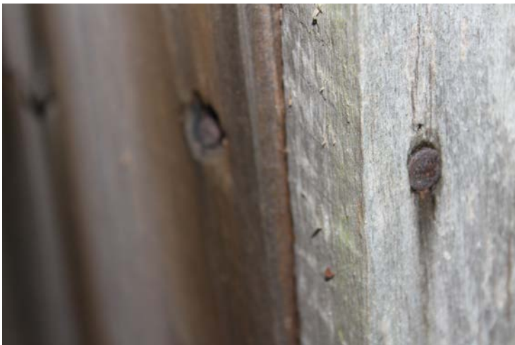
Fig. 21: Type B Cut Nail, 1820-1900 (Photograph by Stephanie Shaw).
