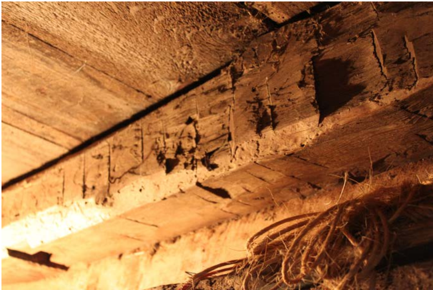
Fig. 20: Hand hewn marks on Post and Beam barn (Photograph by Stephanie Shaw).
