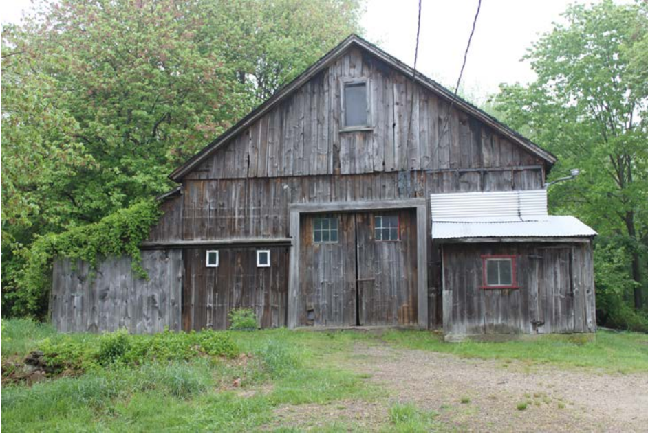
Fig. 15: Gable front barn in Gloucester, Rhode Island (Photograph by Stephanie Shaw).
