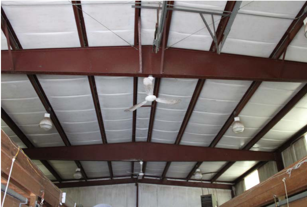
Fig. 22: Metal Framed Barn Interior in Glocester, RI (Photograph by Stephanie Shaw).
