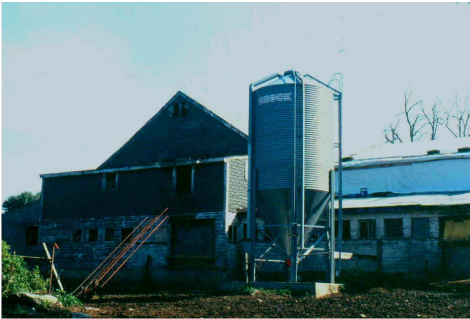
Fig. 18: Metal Silo at the Barton Farm, used for dispensing commercial feed (RIHPHC 2010: Photograph on File).
