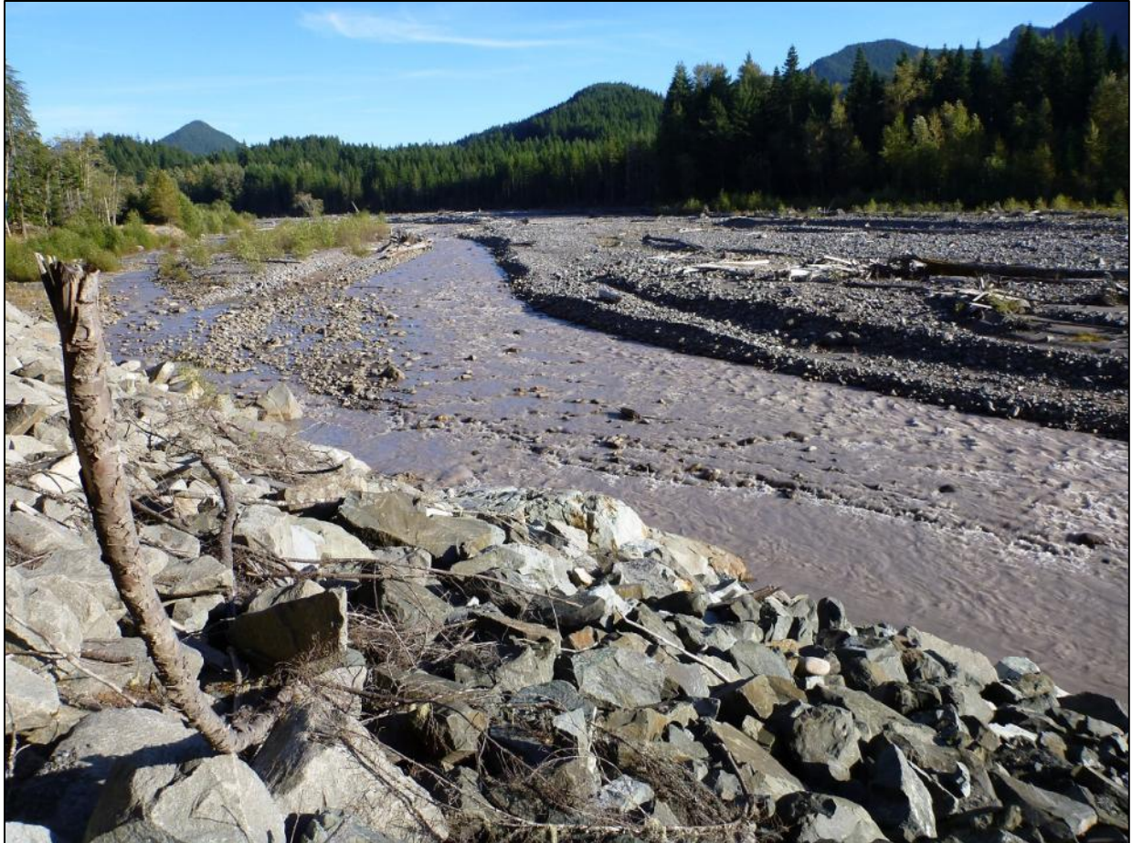
Figure 13. Photograph of the Nisqually River at Park boundary sample reach illustrating the broad floodplain and braided channel characteristics. Note: Bank armoring/rip-rap in the foreground.
