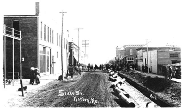
State Street, c. 1919. Installation of Sewer Lines. Norton Historical Society
