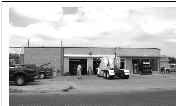
210 North First Avenue
