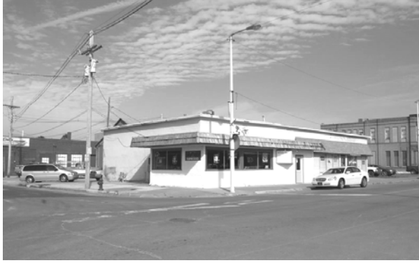
Detached Modern Movement Style c. 1960 Building 109 W. Washington. (Note parking lots at rear and sides of building.)
