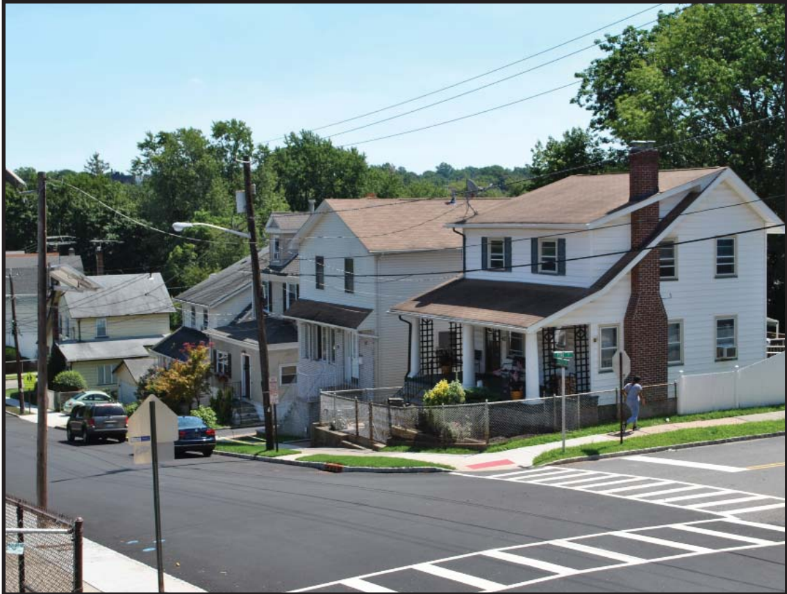
Photograph 2.5. Educational Park Section, view looking east on Hazel Avenue from Pine Street (photographer Eryn Boyce, August 2016; HRI Neg.#16043/D1:0101]).
