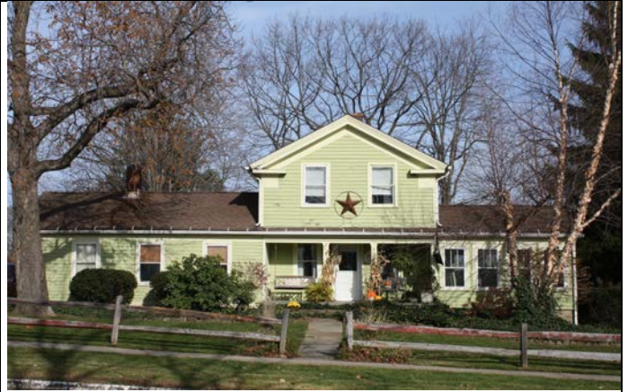
Greek Revival. Cramton House. 13918 Kirtland St. GEA0025104
