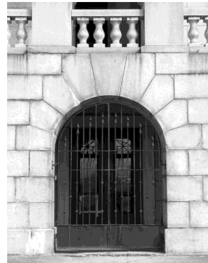
Ground Floor Entry
