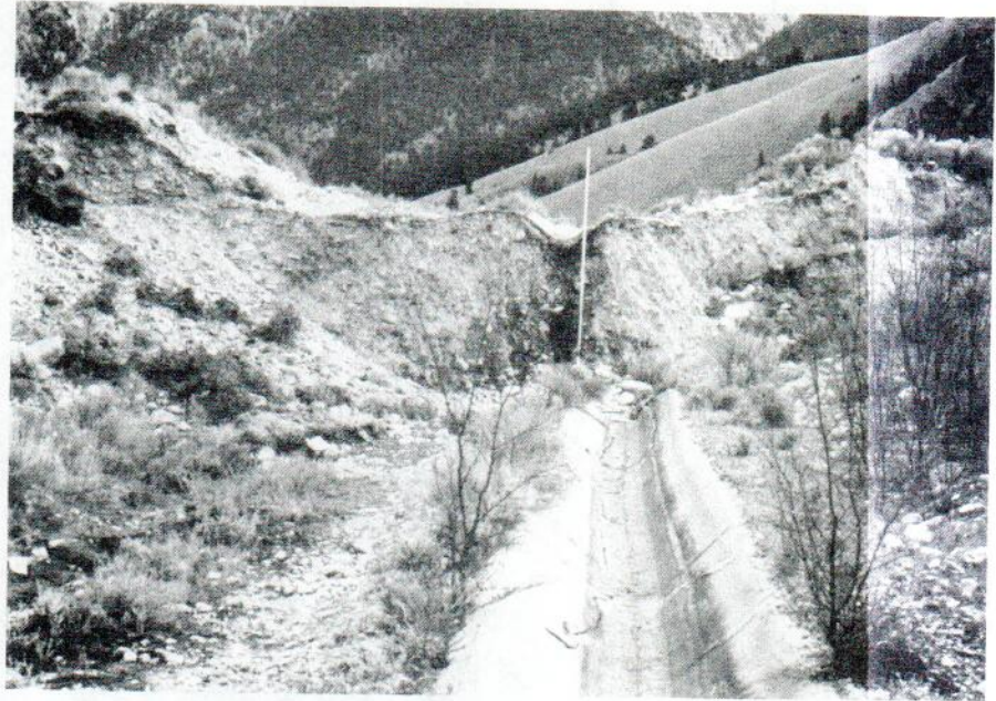
FIG. 6. Faulted concrete irrigation ditch at Rock Creek showing component of sinistral slip (see Plate 1). Vertical displacement of the ditch is 2.90 m, and sinistral slip is 0.43 m. Stadia rod is 4 m long. Photograph by A. J. Crone, 30 October 1983.
