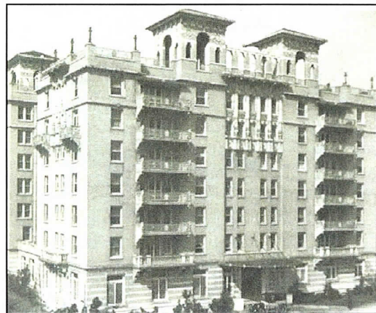
Meridian Mansions (now the Envoy) was originally capped by a roof terrace with pavilions, railings and decorative light fixtures. Replication of such missing elements is encouraged.
