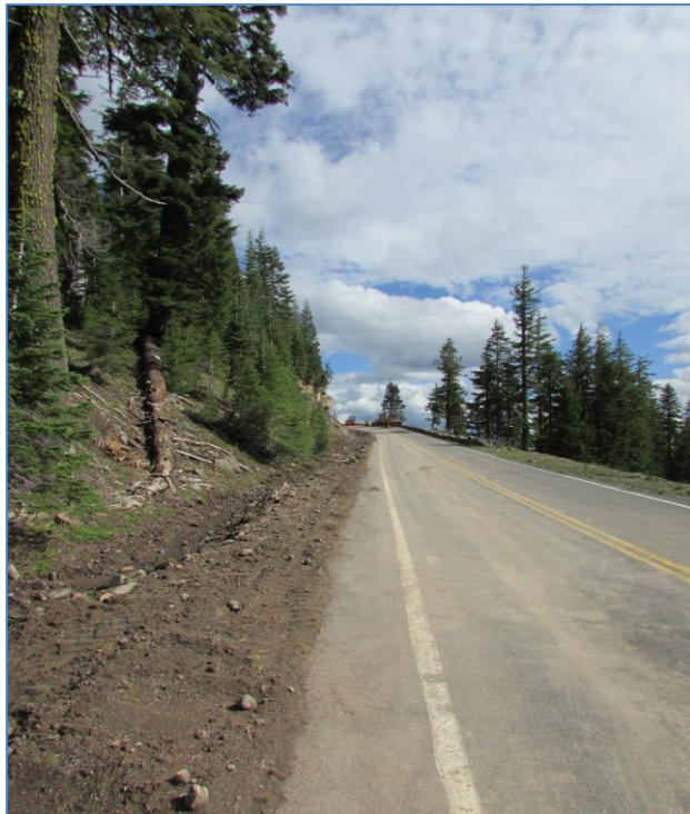
Figure 7. Roadside maintenance in a rockfall-prone area along East Rim Drive exposes mineral soil, facilitating invasive plant introduction and spread. Photo by Jen Beck.
