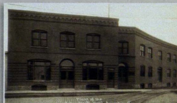
The John W. Tuthill Lumber Company has undergone a complete restoration and today houses a local interior design store.
