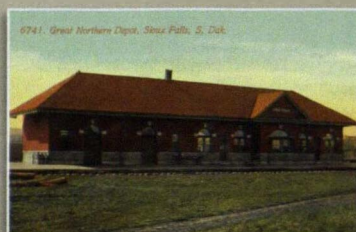
Located at 505 East 8th Street, the Great Northern Depot is an example of the Richardsonian Romanesque style architecture using native quartzite stone.
