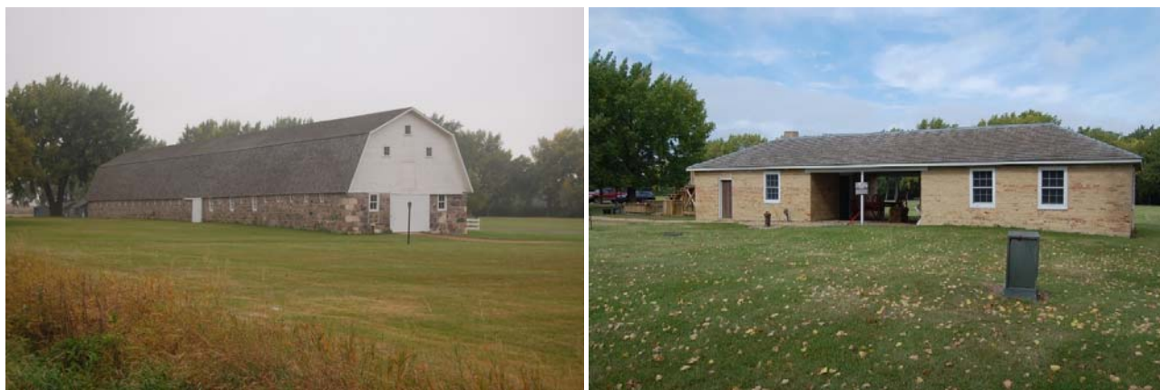
Figure 11. Stable and Carpenter's/Blacksmith's Shop
