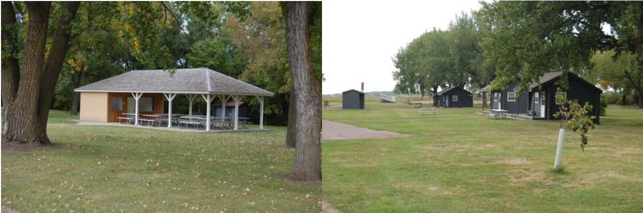
Figure 13. Picnic Shelter and Camping Cabins
