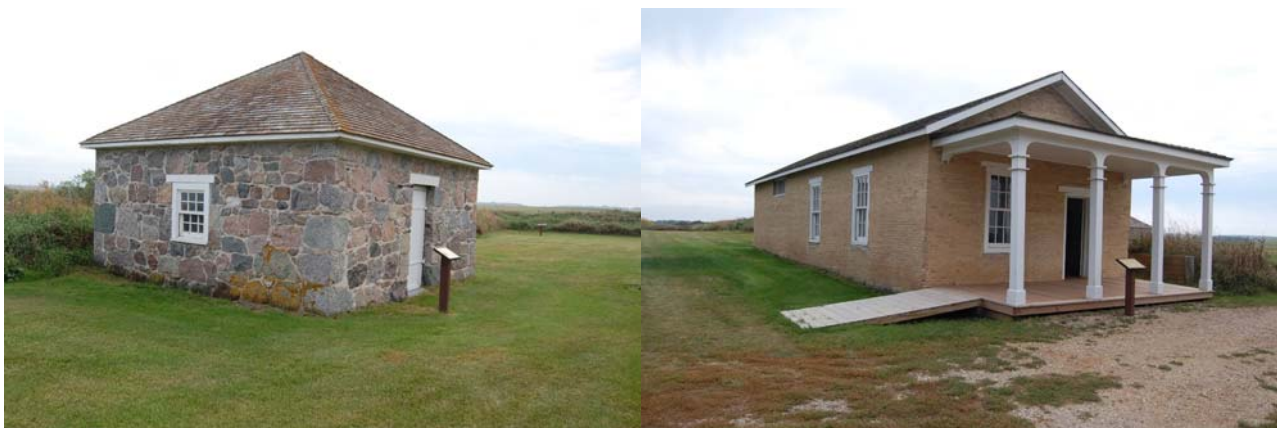
Figure 5. Oil House and Guard House
