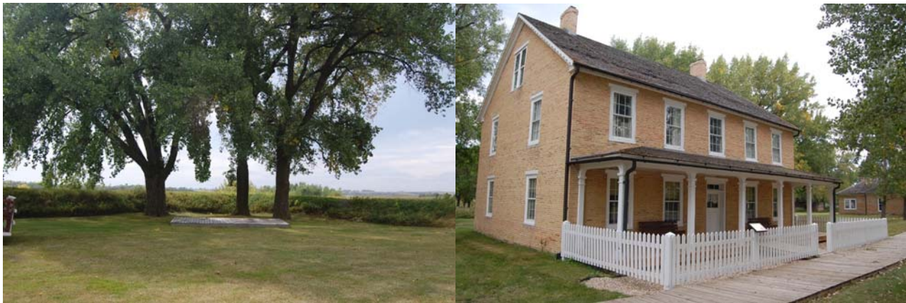
Figure 8. Original Magazine Site and Commanding Officer's Residence
