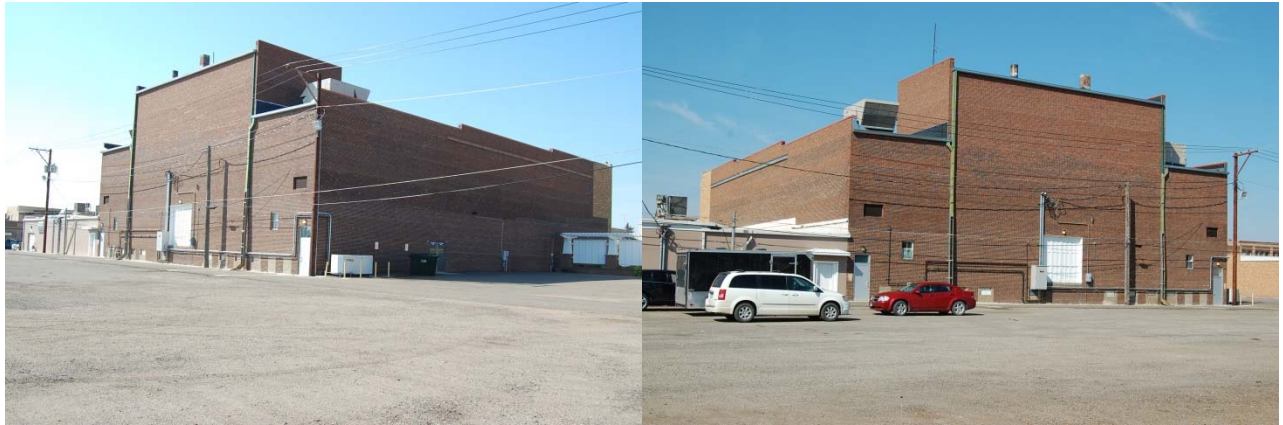
Figure 4. Mobridge Auditorium, Facing Southwest and Northwest
