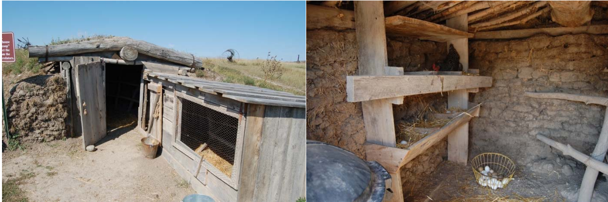
Figure 10. Reconstructed Chicken Coop, Facing Northwest (left) and Interior (right)
