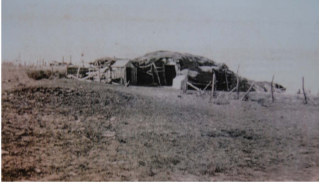
Figure 14. The 1913 photograph is believed to show the “straw barn,” west of the existing barn, no longer extant
