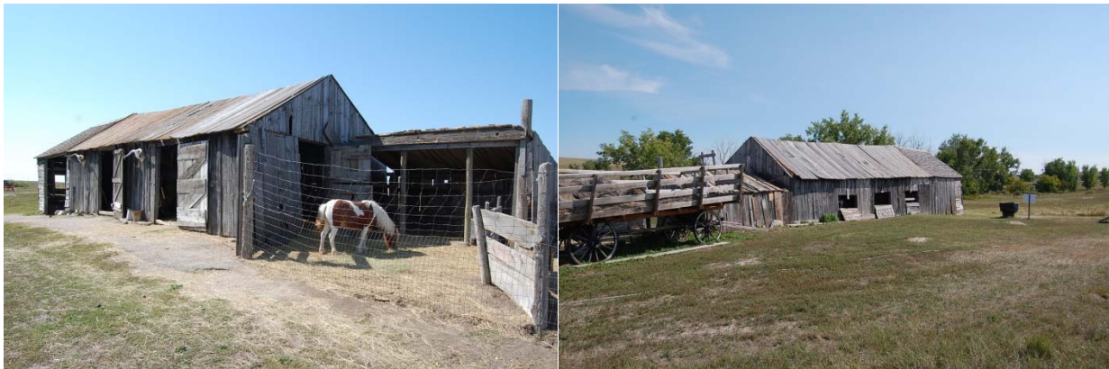
Figure 11. Barn, Facing Southwest (left) and Southeast (right)
