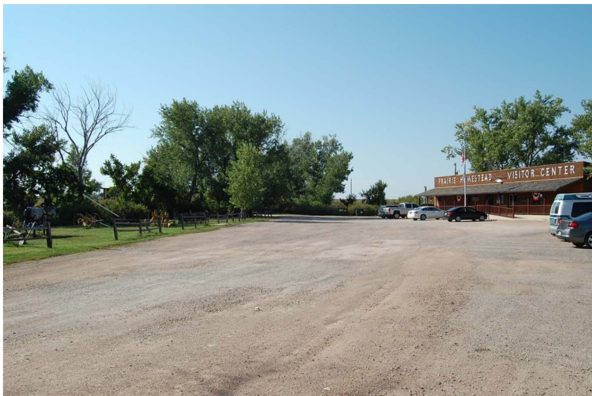
Figure 1. Current visitor center, gravel parking area at entrance from Highway 240 (left of view), facing Southwest
