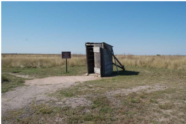
Figure 9. Reconstructed Privy, Facing Southwest
