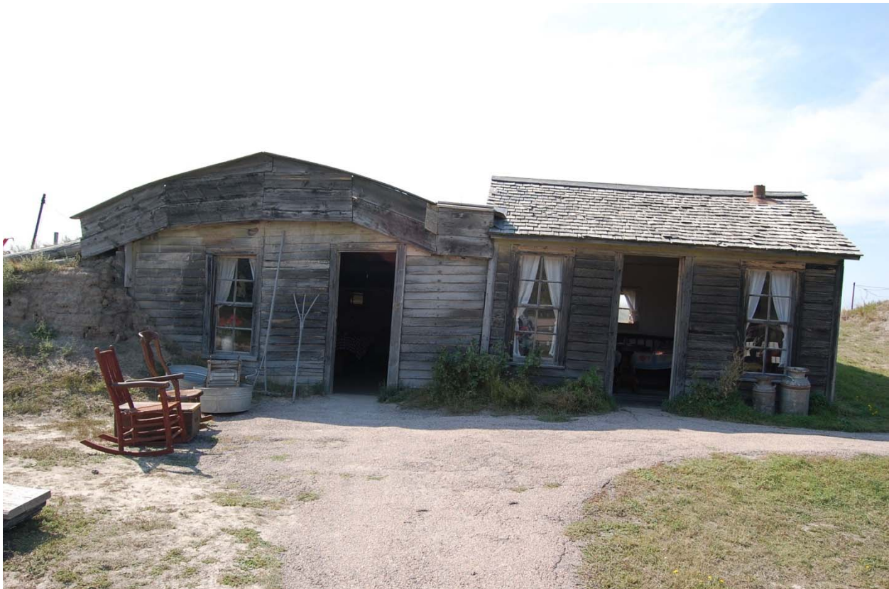
Figure 3. Façade of Dugout (left) and Claim Shack (right), Facing West
