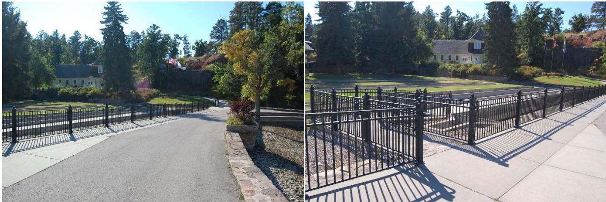
Figure 18. Examples of Modern Sidewalks and Railings
