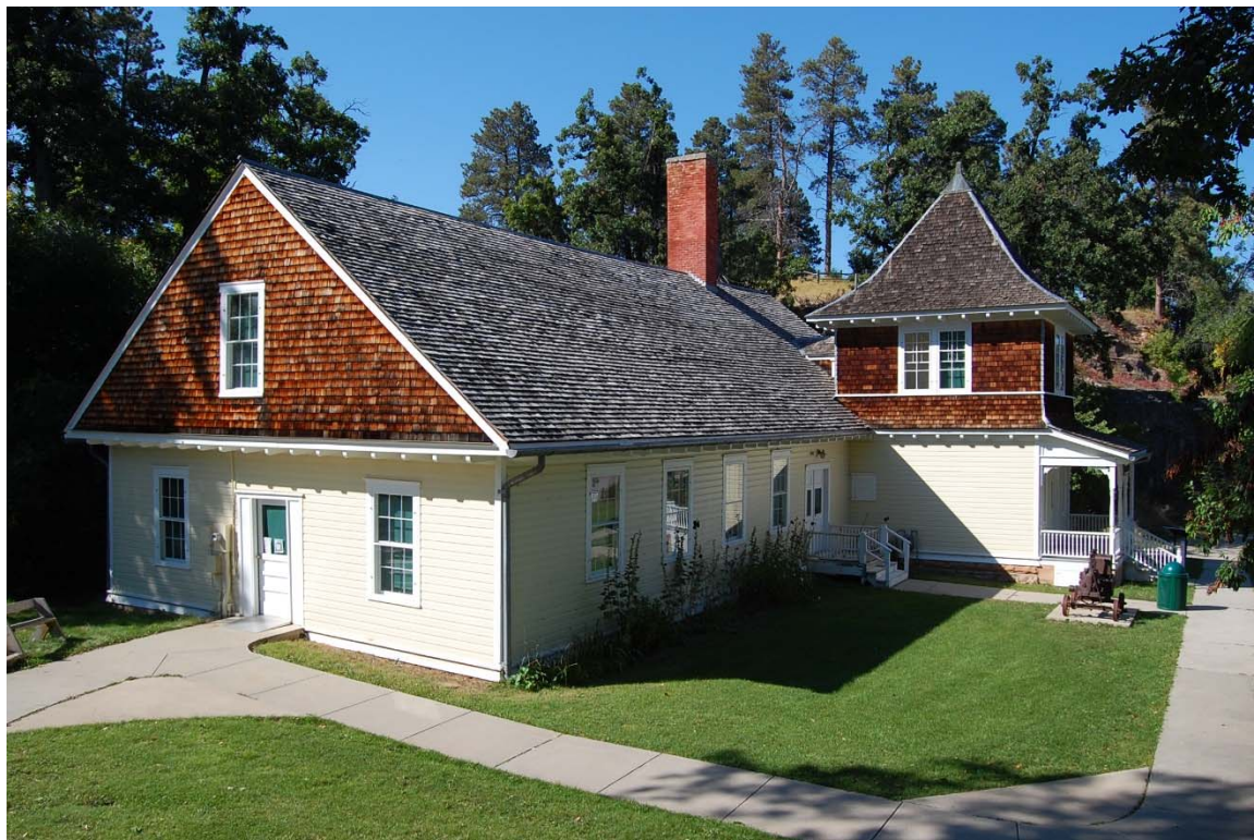
Figure 3. Hatchery Building, Facing NW
