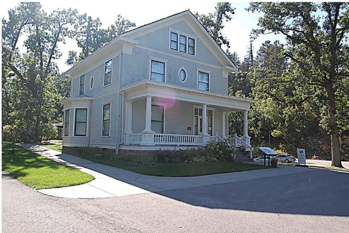
Figure 4. Superintendent's Residence, Facing SW
