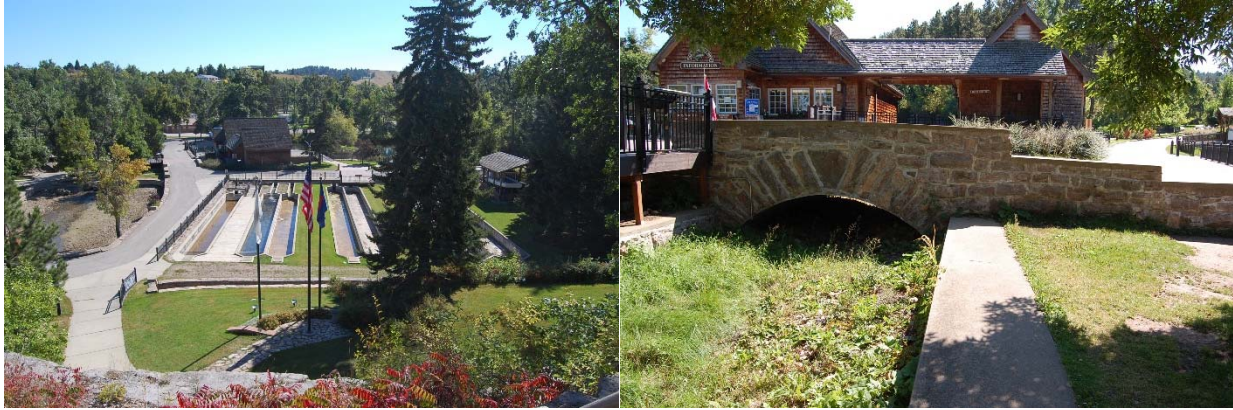
Figure 10. Raceways, Facing E; Masonry Bridge, Facing S
