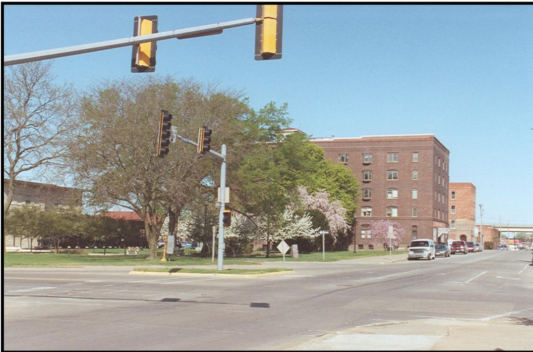
Figure 75 200 block W Main with 302 W Main in background, looking west
