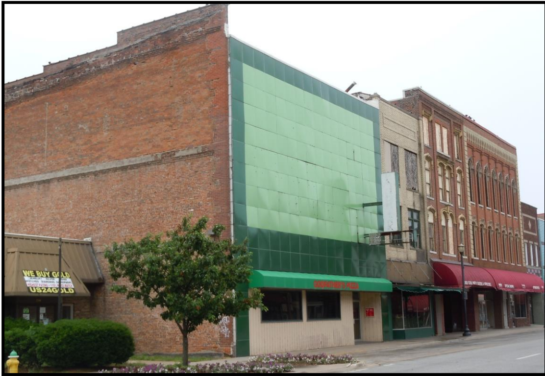
Figure 87 200 block E Main, site of the Union Block
