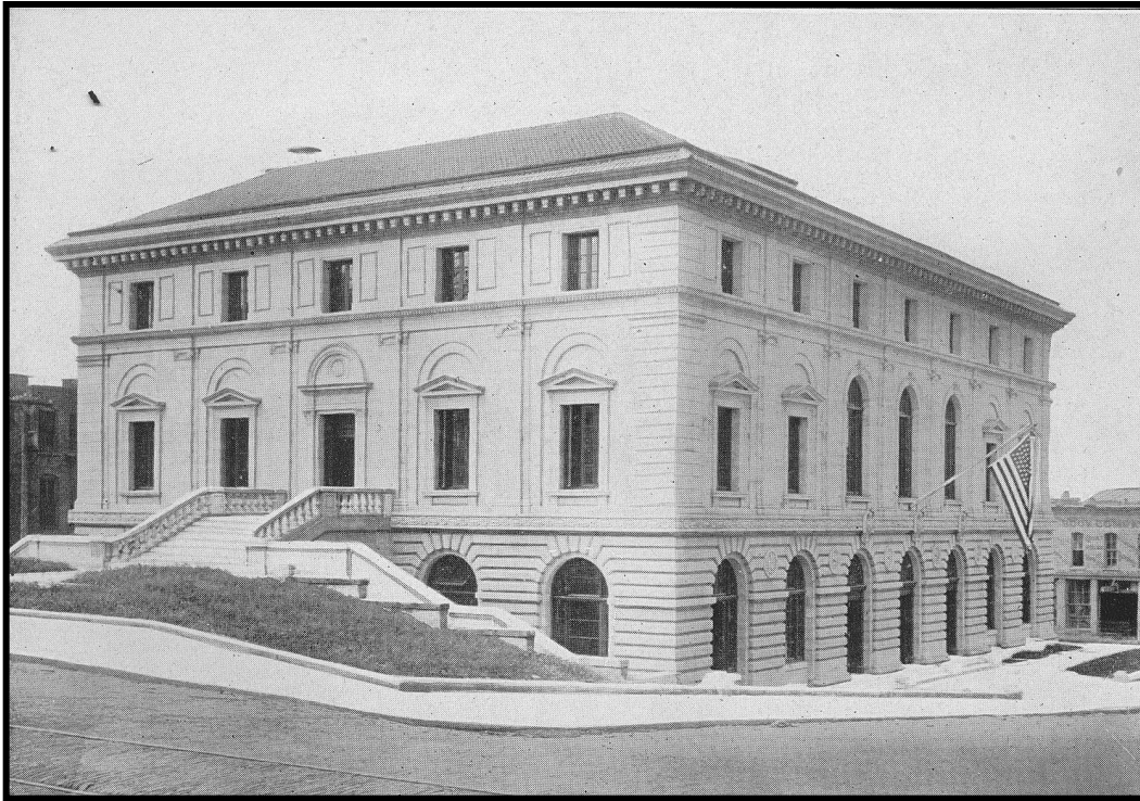
Figure 33 US Post Office/Federal Building (NRHP), 1910-12 Third Street on east side Central Park
