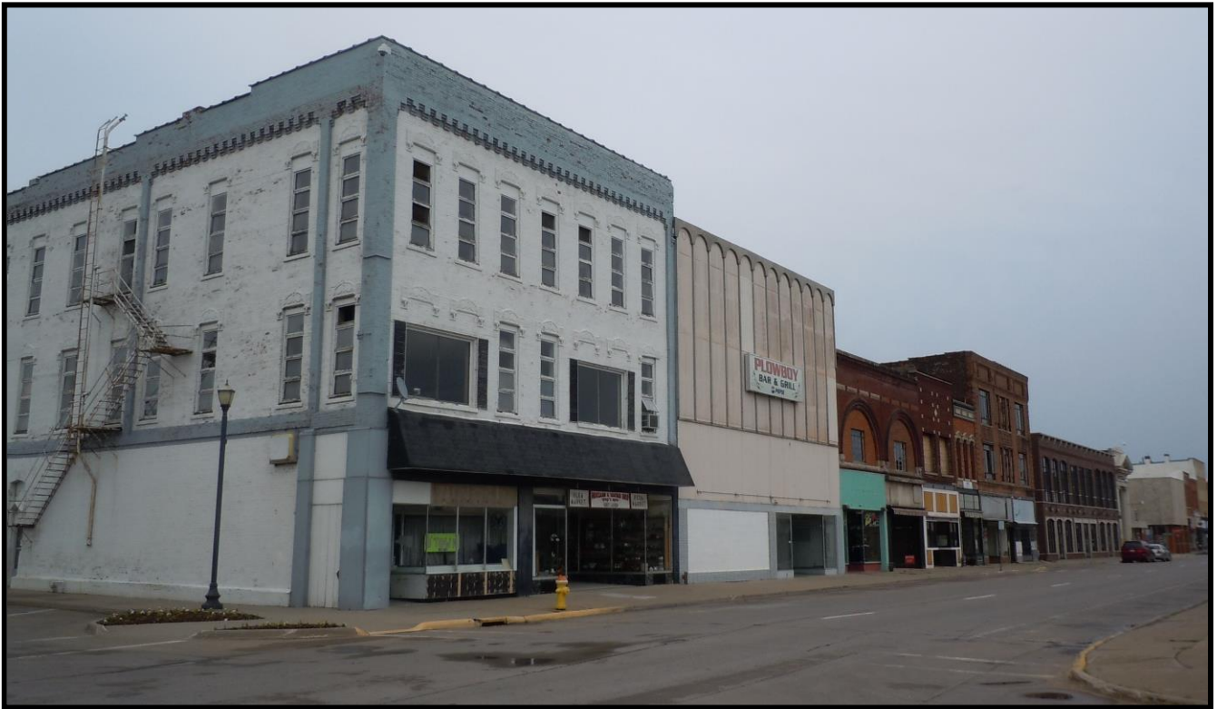
Figure 79 100 clock E Main, north side from Court
