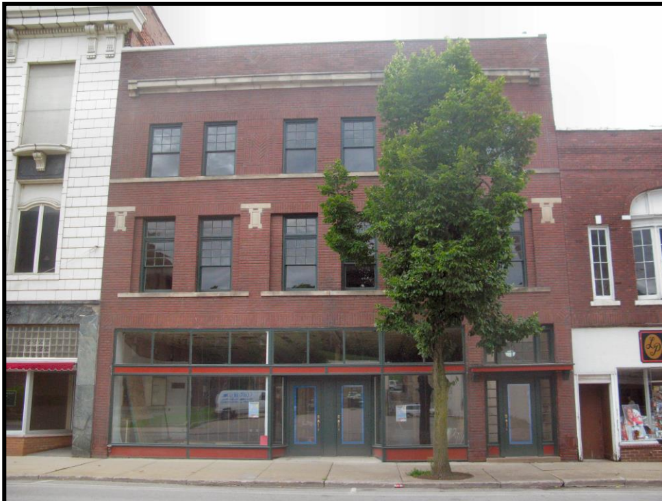
Figure 40 Utt Building and Garner Building (NRHP), 2012
