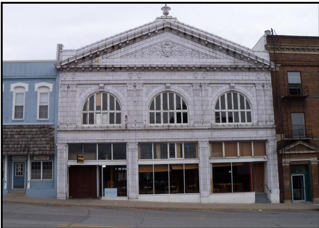
Figure 49 Benson Block (NRHP), 1924 108-112 N Market
