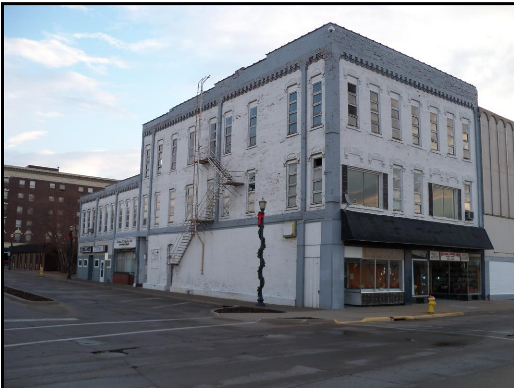
Figure 106 100 block S Court, east side facing new construction
