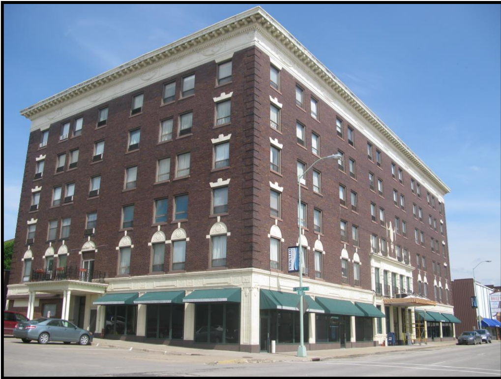
Figure 93 100 block E Second, north side from Court
