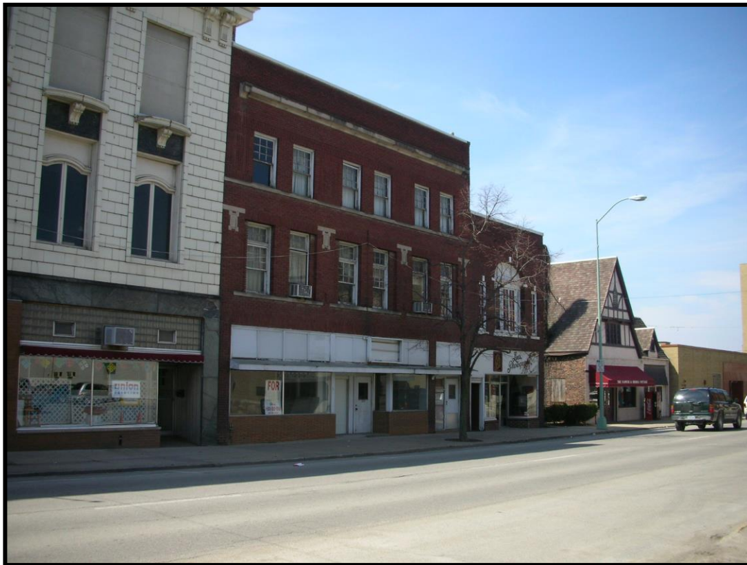
Figure 102 200 block E Main, south side, middle
