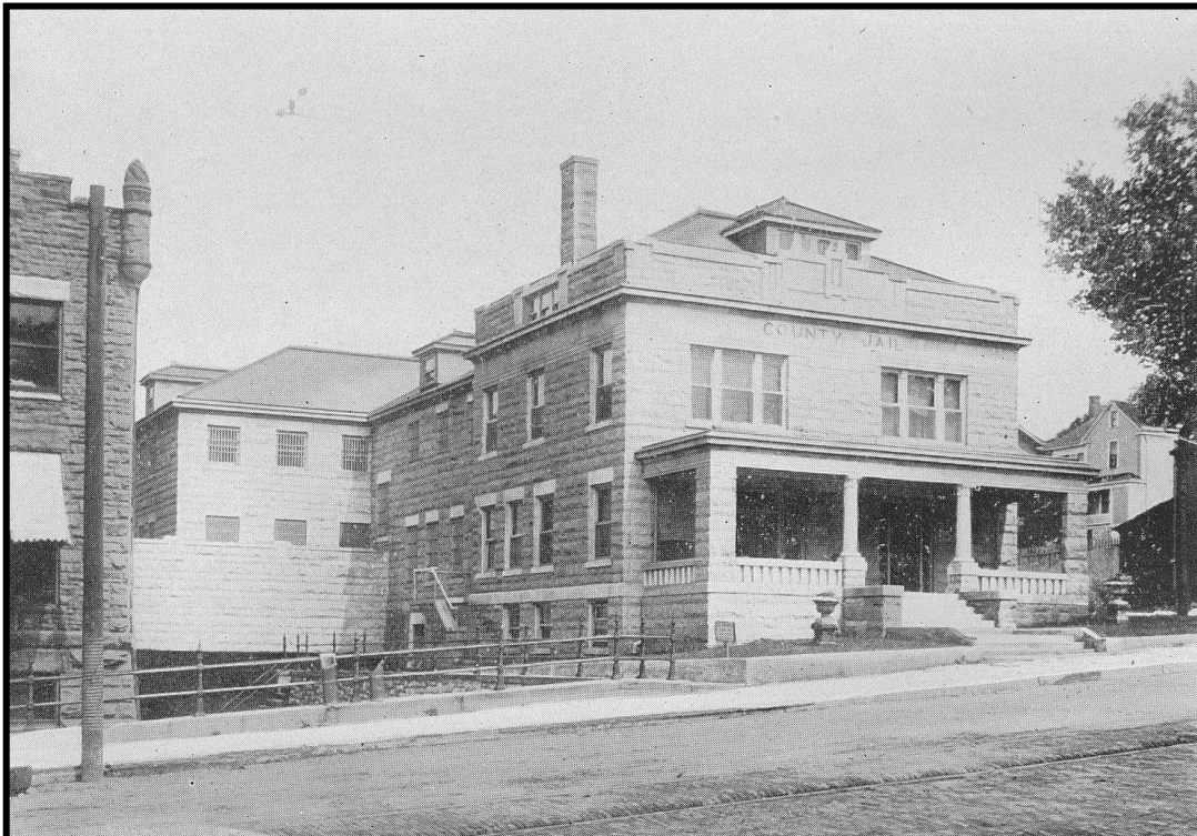
Figure 34 Wapello County Jail, 1910 N Court just north of Fourth Street
