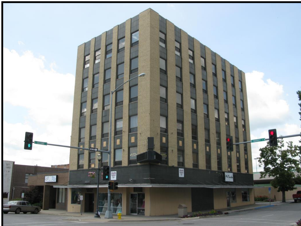
Figure 96 100 block E Second, south side from Market
