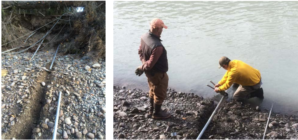
Figure 3. Installation of a new permanent well/sensor array at Nabesna River. The well pipe is pounded through the bank at an angle (left hand photo), then a perforated well tip containing a pressure transducer is attached to the end of the pipe and buried in the sediment in the river (right hand photo). A cable carrying power and communication runs from the transducer up through the pipe to the datalogger at the transmitter station.
