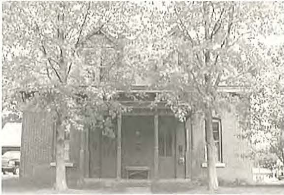
Henry Bauch House 1037 South 16 th Street
