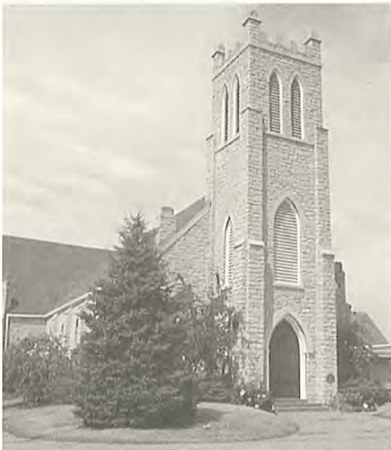
St. John's Episcopal Church 701 Hampshire Street
