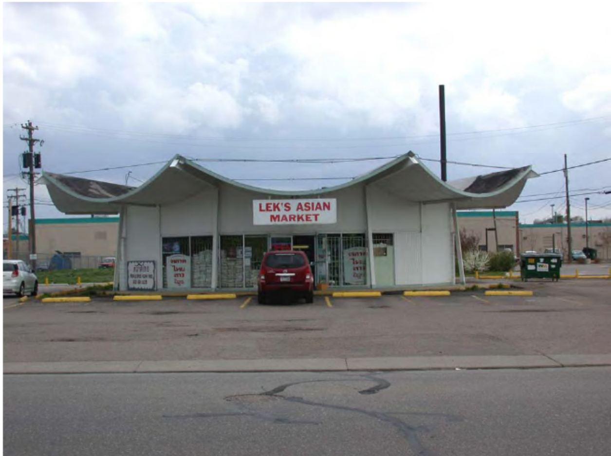
Hoehn Architects PC (April 2010)
