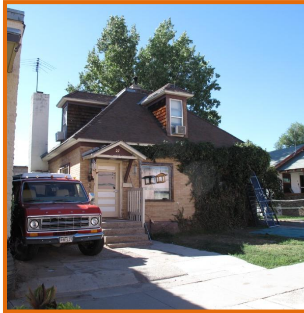
Photograph 2: The oldest building in the survey is the home at 27 North Beech, built about 1900.
