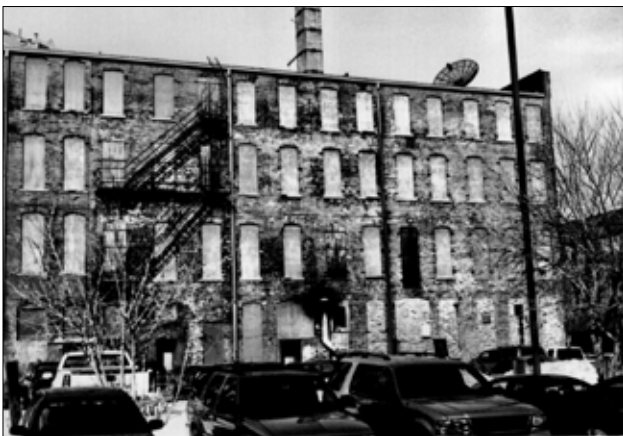
This early photo of the Seth Richards commercial block shows the side of the spaghetti factory building with fire escapes and blocked in windows.
