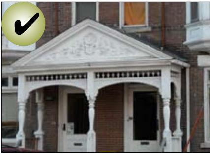
Maintain an original porch.
