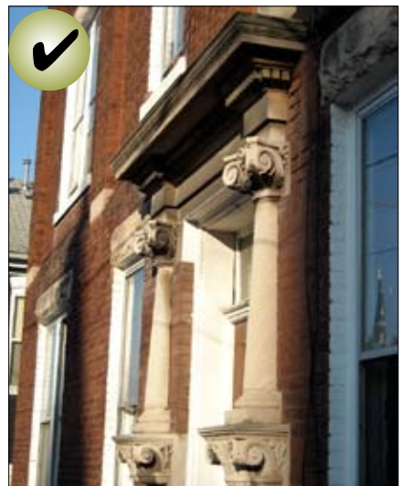
Features such as these collonettes should be preserved in order to avoid the need for replacement in the future.
