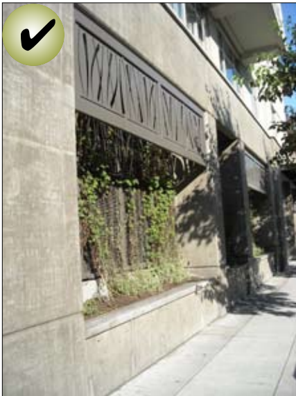
The parking structure reflects a visually attractive edge with recessed areas that contain landscaping and creative screens. Note these conceptually reflect storefront elements.
