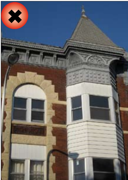
Inappropriate profile for window replacements; the proportions are inaccurate.
