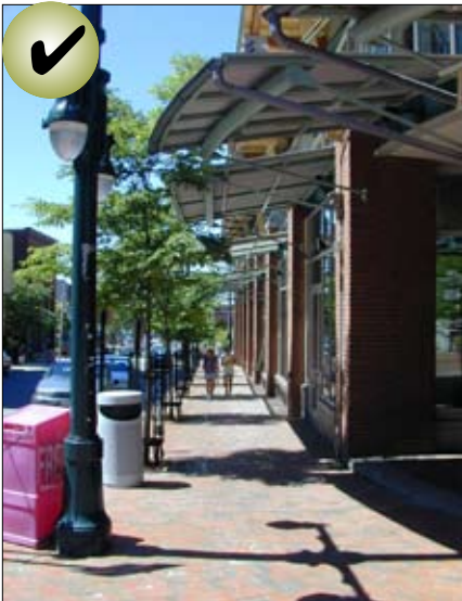
Wall mounted brackets are appropriate supporting mechanisms for fixed metal canopies.
