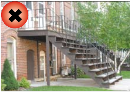
Inappropriate design on a primary facade.
