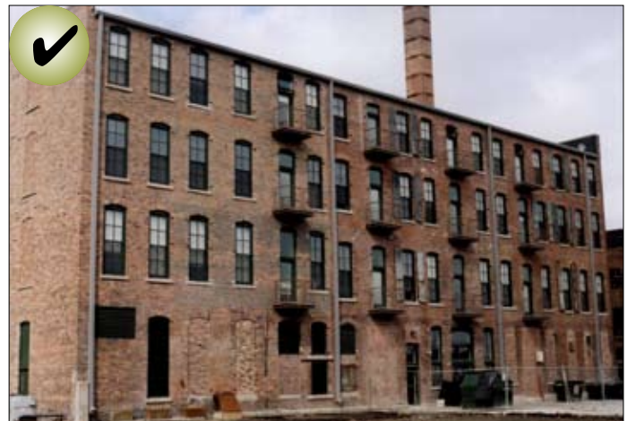
In a later rehabilitation the fire escapes were removed and a limited number of simple metal balconies were installed.
