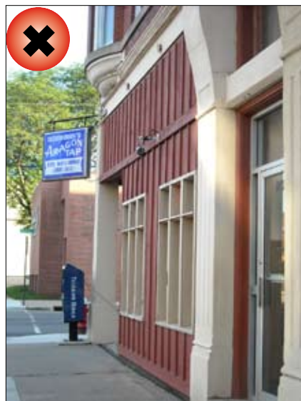
Inappropriate storefront modification.
