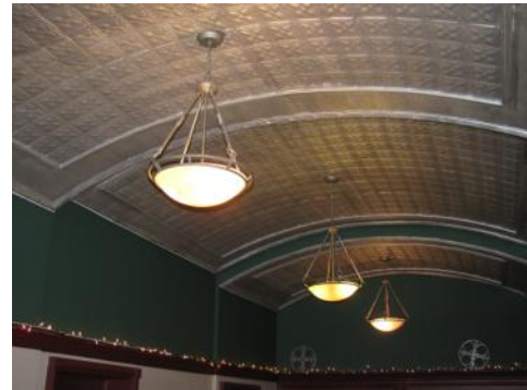
Main Lobby Decorative Pendant Lighting
