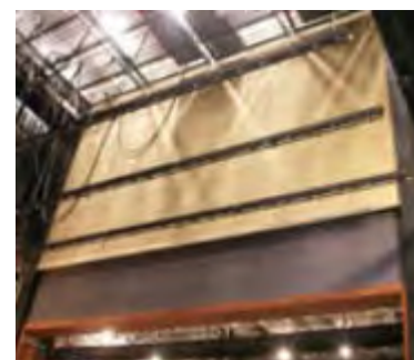
New Brail Fire Curtain System
