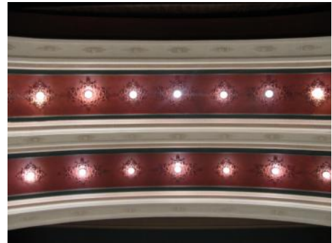
Proscenium Arch Incandescent Lighting
