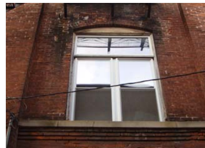
South façade window
