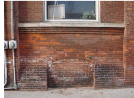
South façade base detail
