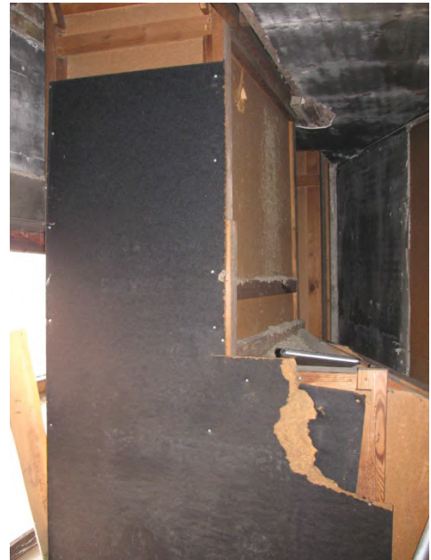
Existing supply duct riser, stage-left
