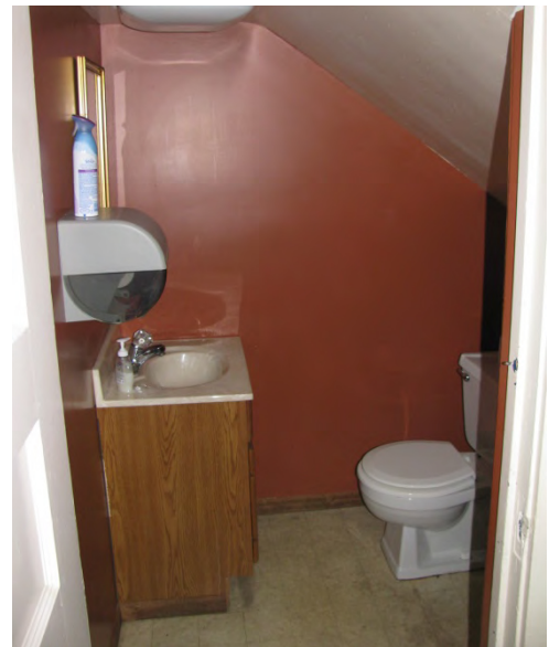
Existing typical plumbing fixtures
