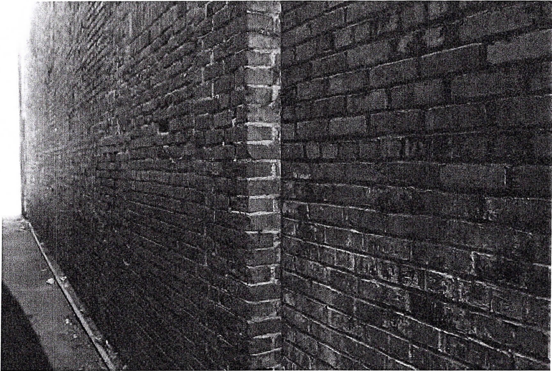
Masonry Wall in Alley Way (note differing bricks and evidence of openings bricked in)
