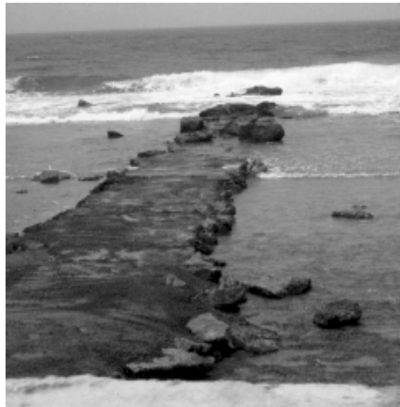
Figure 9. Seawater intake pipe at the RRE clam farm in Majuro, RMI. Note the pipe has been coated with concrete to reduce damage from wave action on the reef flat (Eileen Ellis).
