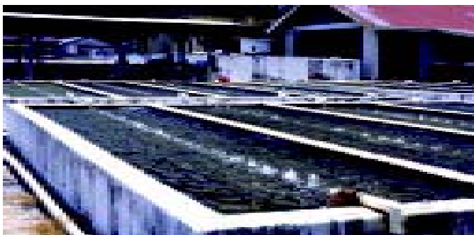
Figure 17 (Left). Concrete block raceways at the Palu Mariculture Demonstration Center, Palau. Note the low height and shared center walls (Eileen Ellis).
