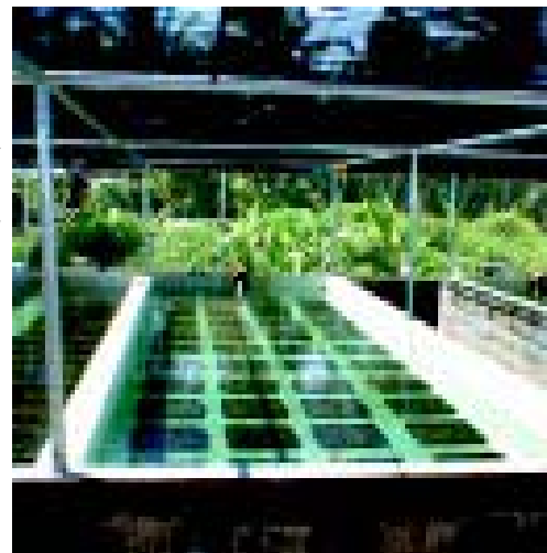
Figure 16 (Right). Concrete block raceway at RRE Clam Farm in Majuro, RMI. Note the overhead shade cloth and epoxy coated walls. (Simon Ellis).
