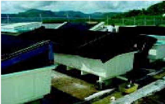
Figure 11 (Left). Fiberglass grow-out tanks at the Lenger Island giant clam hatchery, Pohnpei State, FSM. The roof over the tanks is to protect the clams from the locally heavy rainfall. (Eileen Ellis).
