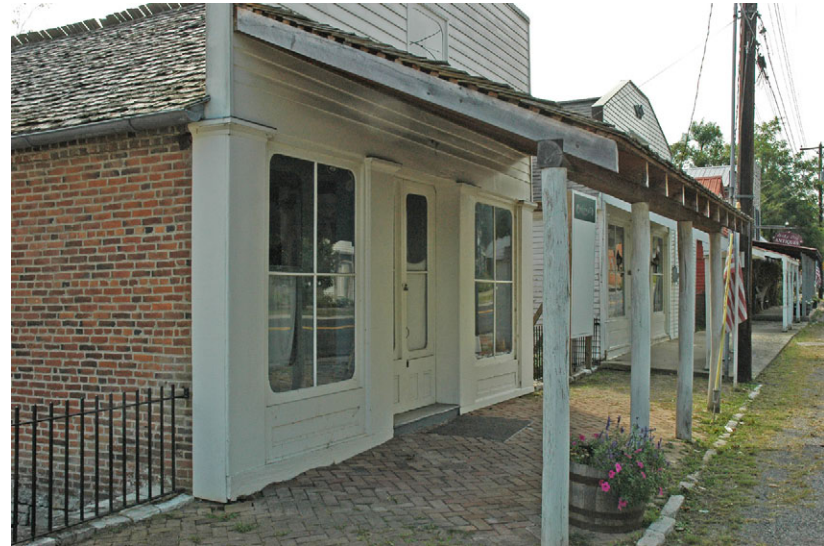
Authentic paving materials can have a patina that is compatible with historic buildings.
