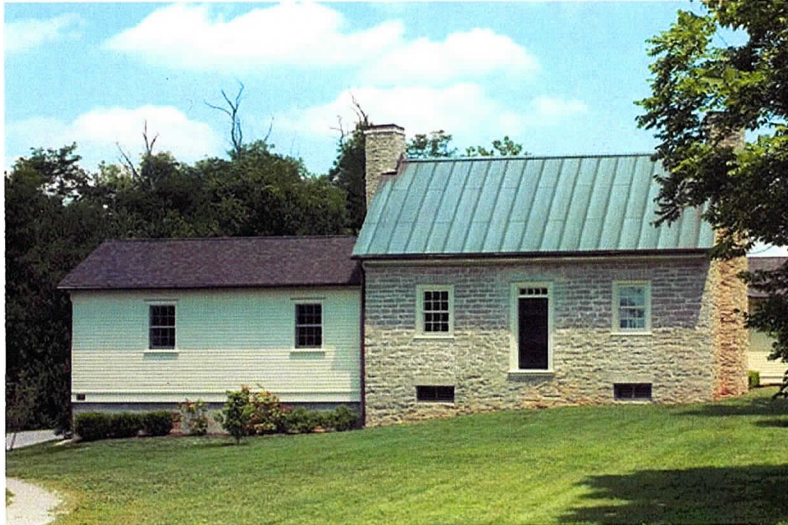
An addition set back from the older building mass yields to its original composition. Photograph: Prajna Design.
