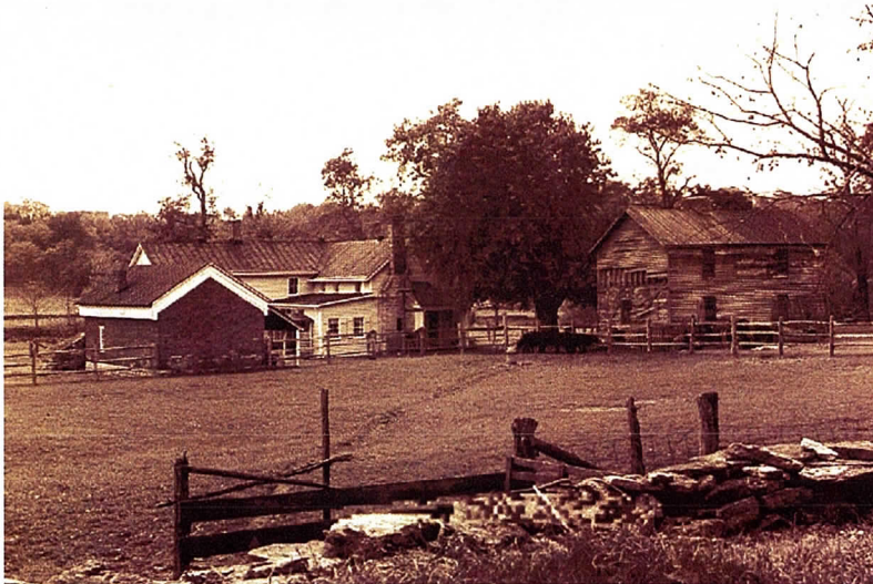
Buildings and small enclosed areas together form the arrangement of a farmstead. Photograph: Julie Riesenweber.
