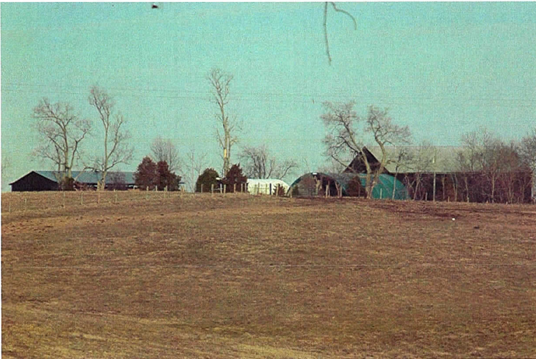
Hoop barns mingled into a cluster of original barns create some intrusion into its character.
