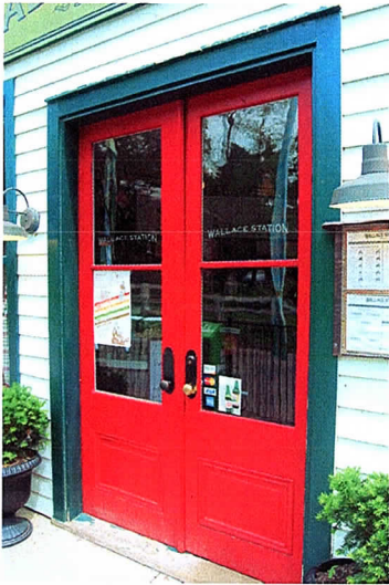
Large doors with windows extend an invitation to enter a rural store.
