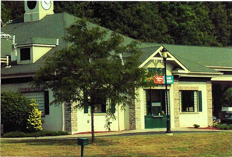
Just like historic buildings, modern buildings benefit from signs that are placed within the proportions of their building forms.
