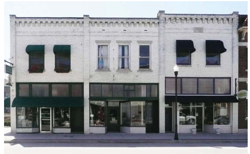
109-115 East Broadway. This grouping of buildings is an excellent example of the use of repetitive elements, including vertical brick piers, second-floor windows, brick corbel string course at the cornice line, transom sash and storefront design.
