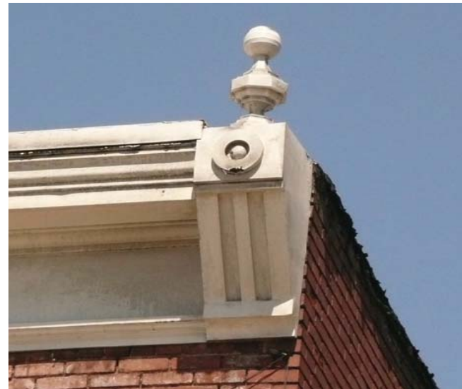
Detail of Metal Cornice
