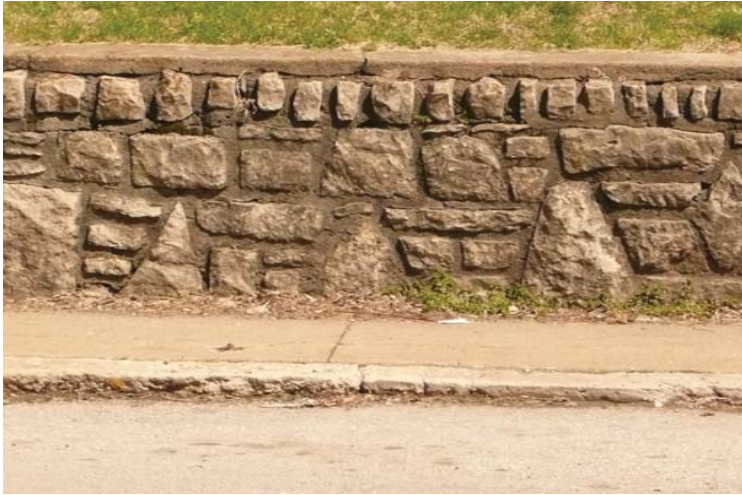
Original Stone Retaining Wall
