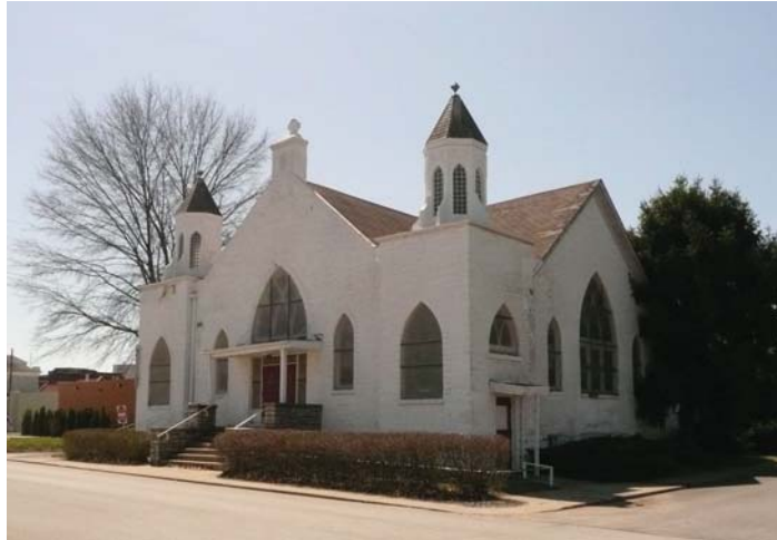
114 North Marietta, Former Methodist Church. The alteration to the shape of the tower roofs drastically changed the appearance of this Gothic Revival Style church.
