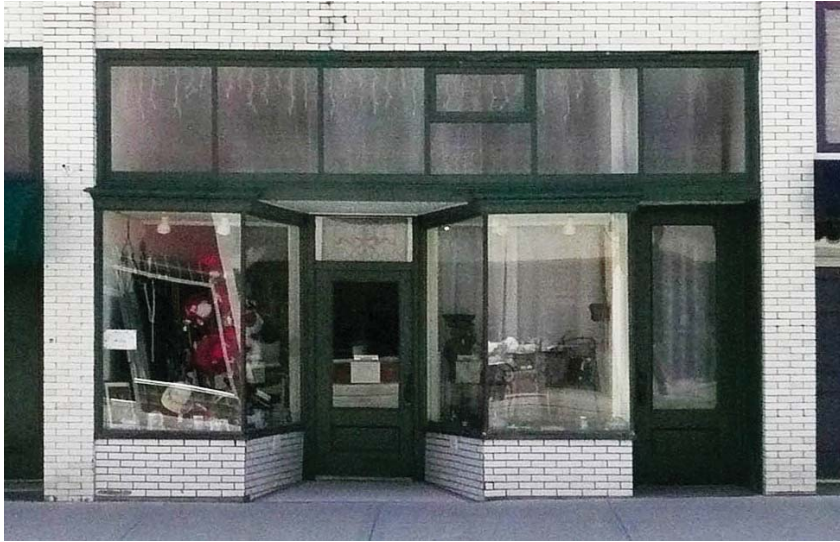
Historic Metal Storefront
