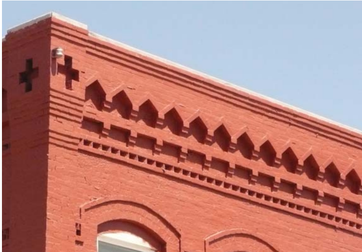
Decorative Brick Cornice
