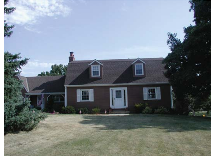
Before New Construction, Addition, Weston, Missouri, 2005
