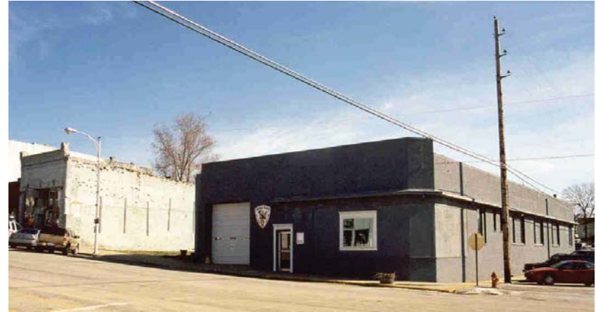
Example of Area Before New Construction, Platte City, Missouri, 2000
