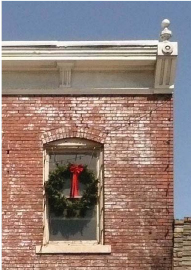
129 109-115 East Broadway, Victorian Commercial, Excelsior Springs, Missouri, 2008.
