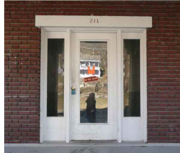
Typical Historic Wood Door with Sidelights
