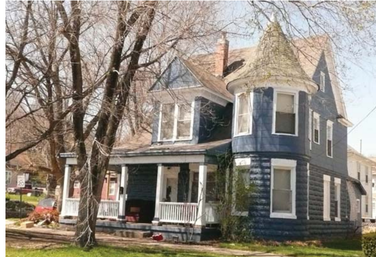
403 Concourse, Queen Anne Style Roof with Multiple Roof lines and Prominent Tower
