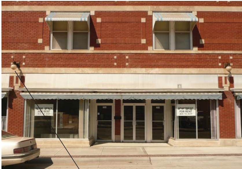
Historic Light Fixtures at the Historic Ideal Hotel. These fixtures should be retained,
