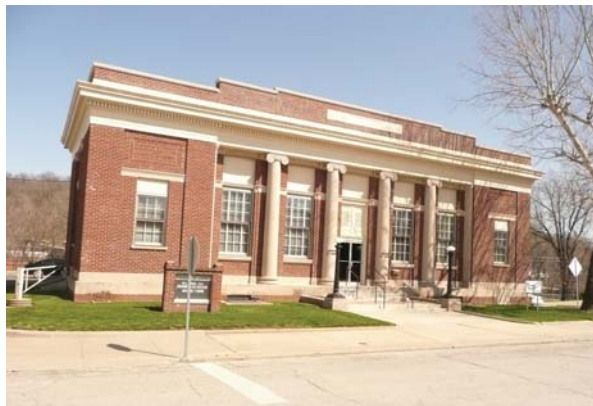
505 Elms Boulevard (Historic Post Office)
