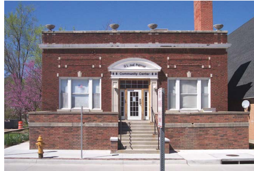
112 Thompson Avenue (Community Center)
