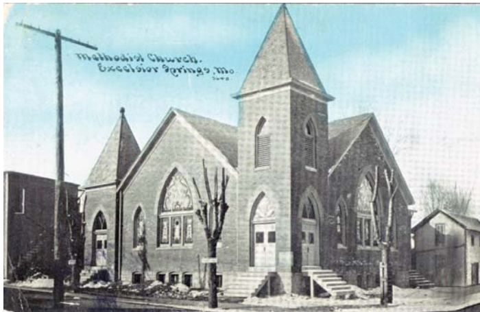
114 North Marietta, Former Methodist Church, Dennis Hartman Post Card Collection
