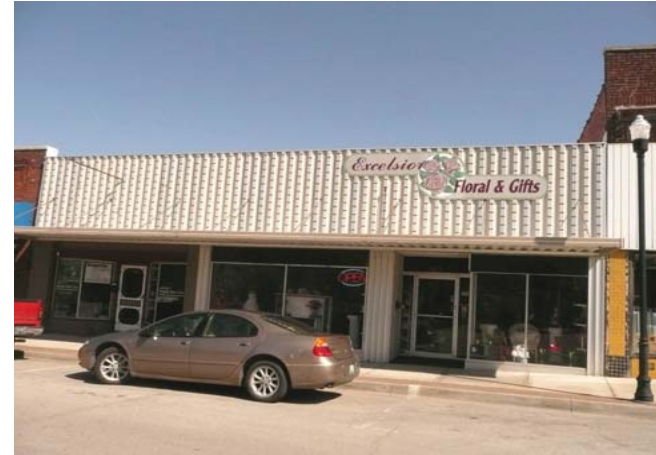
209 Thompson Avenue. According to the Historic Resources Survey, this building has been covered since the 1940s or 1950s.
