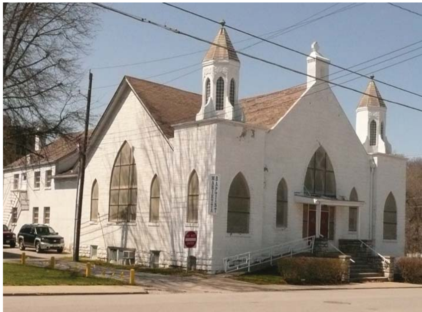
114 North Marietta, Former Methodist Church (c.1905). This church displays an eclectic alteration of a Gothic Revival Style structure, specifically as it relates to the towers and cupolas that flank the main entrance. As seen in the historic photograph to the right, these towers have been altered since the building's original construction.
