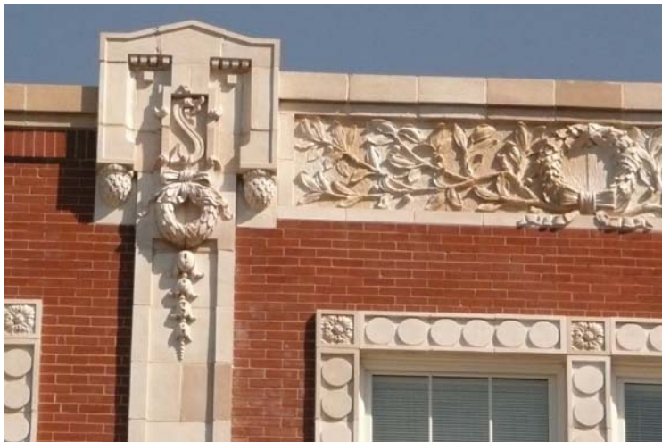
Example of buff-colored terra cotta and red brick, typical materials in the commercial district.
