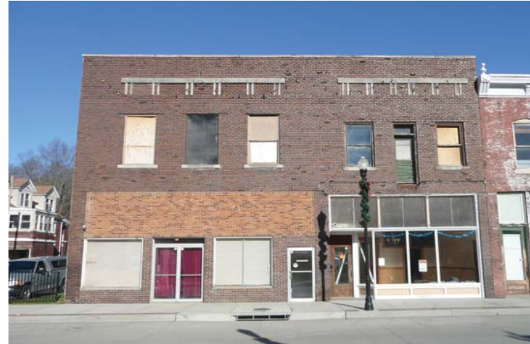
244-246 East Broadway. The owners are currently rehabilitating these buildings. The original storefronts and second-floor balcony should be reconstructed based on the historic postcard below.
