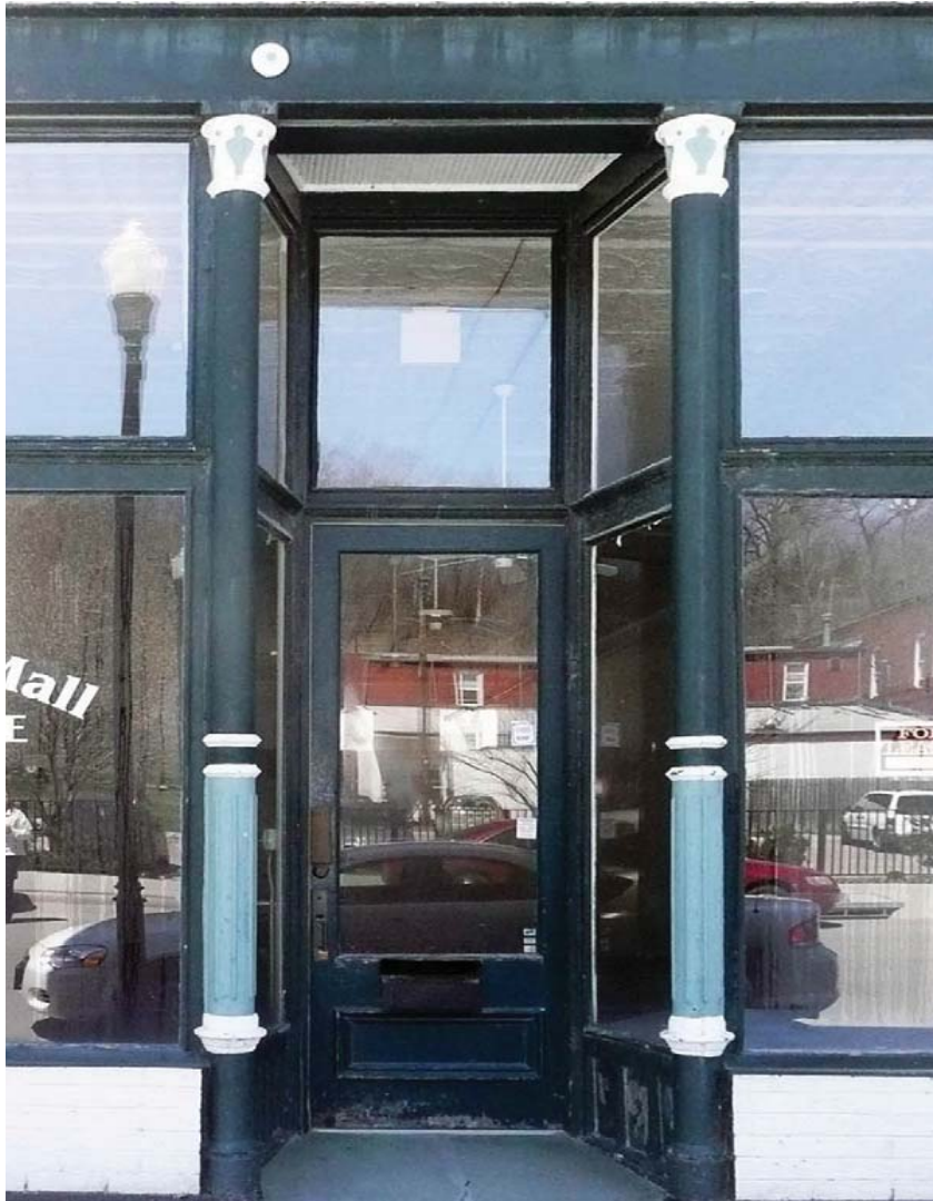
Detail of Historic Cast Iron Storefront
