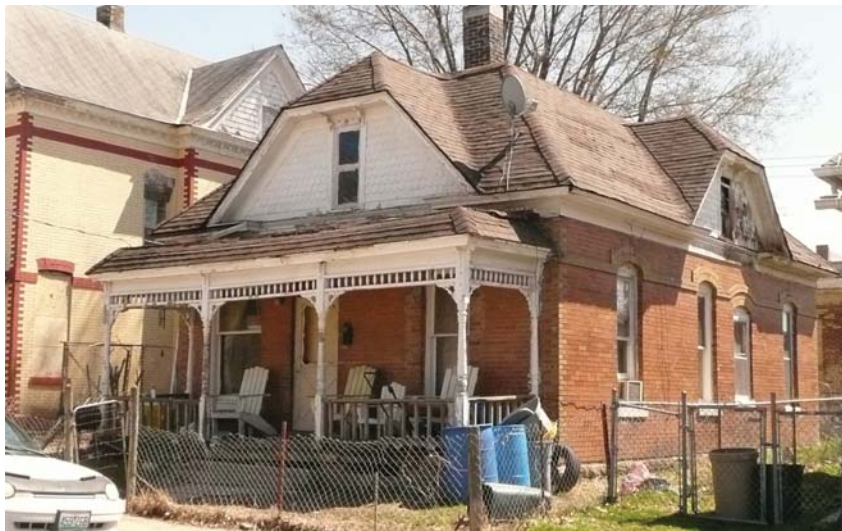
107 West Excelsior (c.1897). Example of the Folk Victorian Style. Note the spindle work porch supports, arched window heads and wood shingle cladding at the gable.
