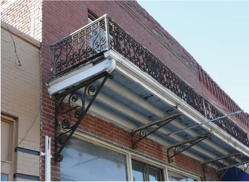
Historic Wrought-Iron Balcony on Broadway
