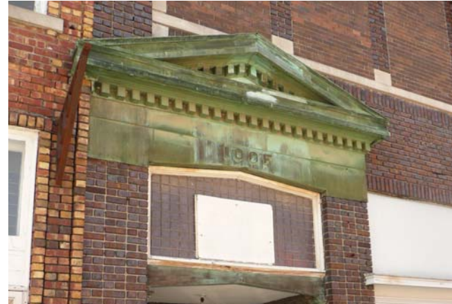
Detail of Copper Pediment at Entry Surround
