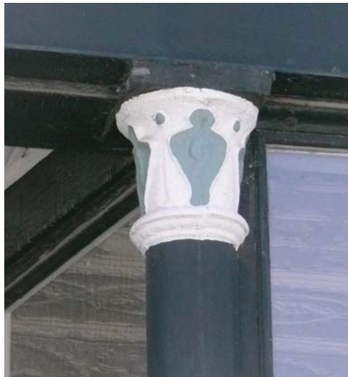
Vernacular Commercial Style, Detail of Cast Iron Column
