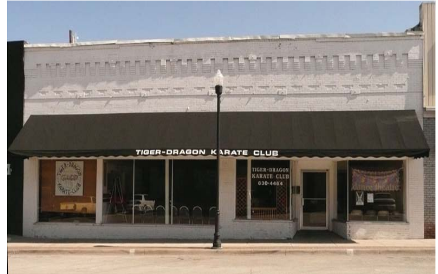
Example of Appropriate Awning, Excelsior Springs, Missouri, 2008.
