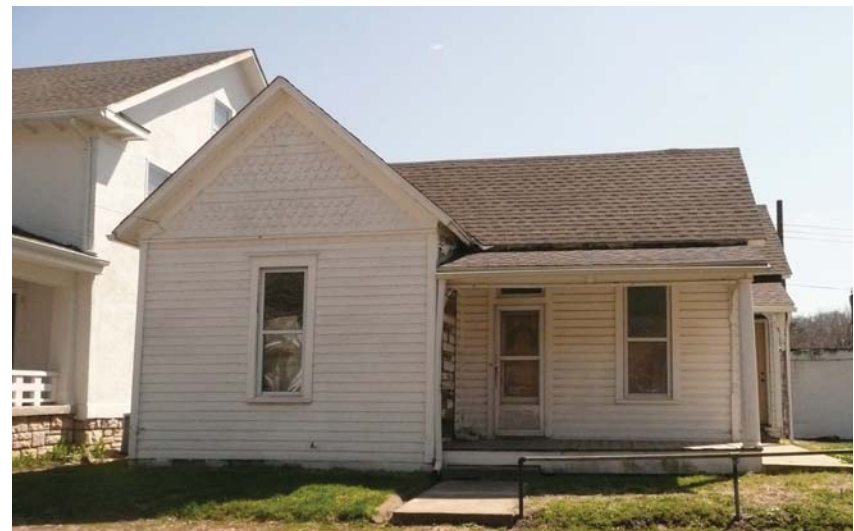
309 East Excelsior (c.1905). Example of the Folk Victorian Style. Note the scalloped wood shingles at the front gable end.
