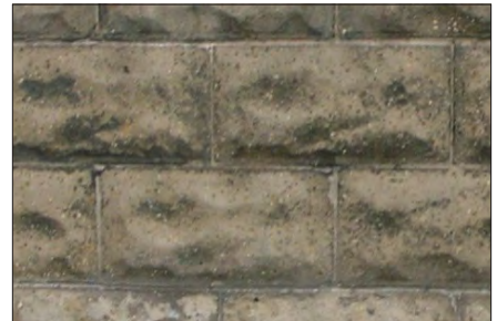
Textured Concrete Block - A structural building material made by mixing water, cement, sand and aggregate, placing it in forms and hardening it; used for foundations, walls and piers, popular in the early to mid 20th century.
