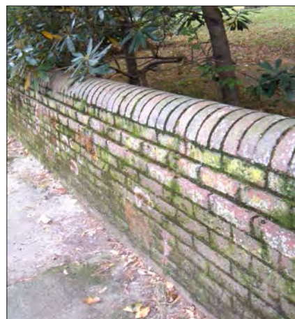
The white, powdery surface on the brick is an example of efflorescence, where water-soluble salts leached out of the brick and mortar. Since the efflorescence is concentrated in the area of repointing, the likely cause is the replacement mortar.
