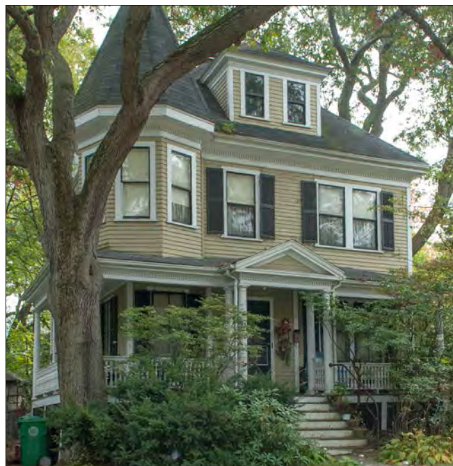
In many Victorian-era homes, such as this example in Auburndale, decorative exterior woodwork is a significant component of the building's architectural style and integrity.
