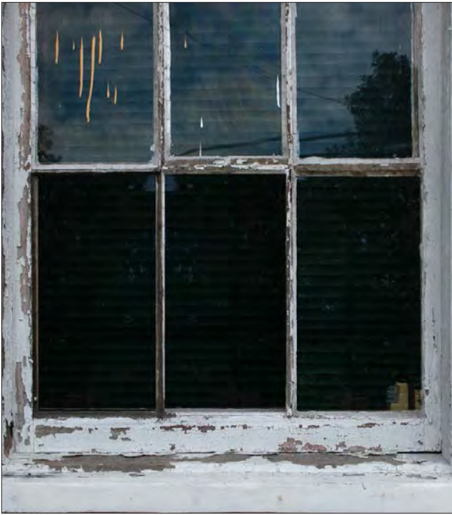
Typically, the deterioration of wood windows first occurs at the sill. Peeling paint can allow moisture to enter wood and cause rot. Regular repainting is recommended to provide a protective layer against moisture.
