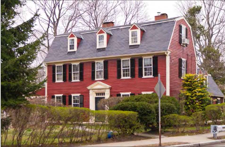
This house in West Newton is a good example of the Georgian Style, with a pedimented central entrance, a paneled wood door, and double-hung windows.
