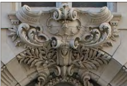
Terra Cotta - Fired-clay, non-structural building components, often with colored glaze, used for decorative, ornate details and wall finishes.
