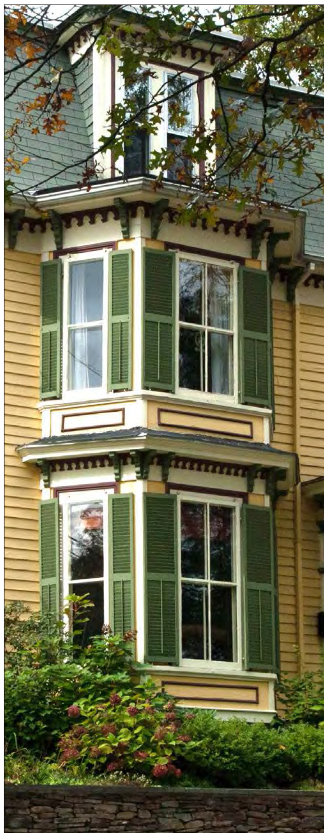
The louvered wood shutters on the projecting bay are appropriately sized for the window openings with the narrower shutters on the side of the bay and wider on the front. Also note the wood exterior storm windows with the vertical and horizontal muntins aligning with each window configuration.
