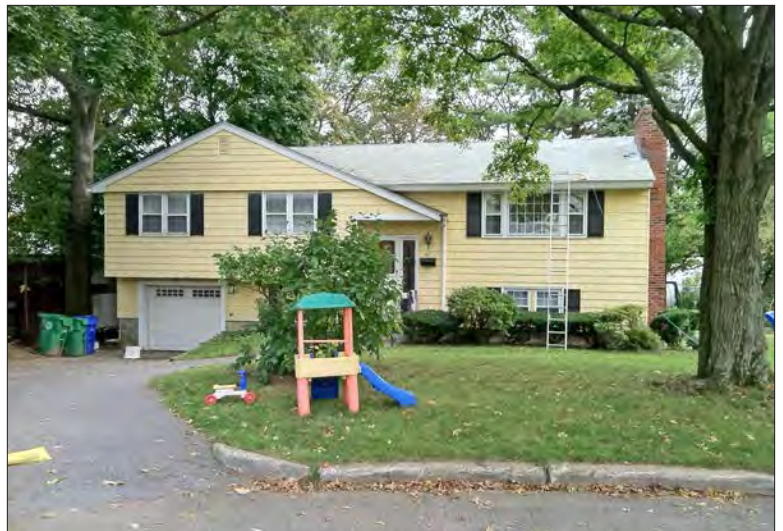
This house in Newtonville is an example of the Split-Level home that became common after World War II, with a low-pitched roof, half-story wing and sunken garage.
