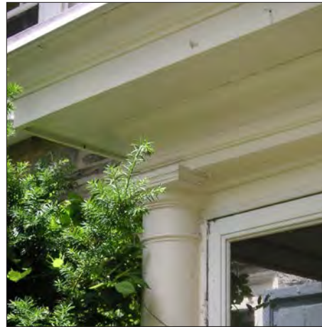
Porch enclosures that are attached to existing decorative porch elements such as this column can cause damage that is both difficult and costly to repair.
