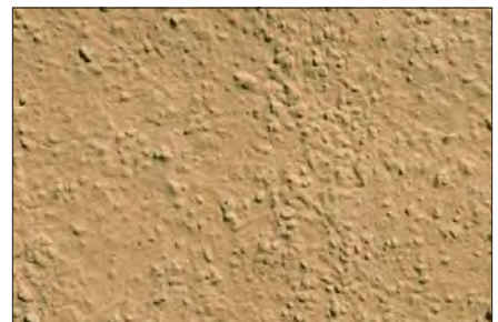
Dash Finish Stucco - Textured finish with pronounced aggregate at the surface.
