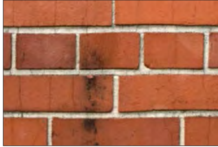
20th Century Brick - A hard, dense, fired-clay, regularly shaped building component; sometimes with a glazed surface; used primarily in walls, piers, foundations, chimneys and exterior pavers.
