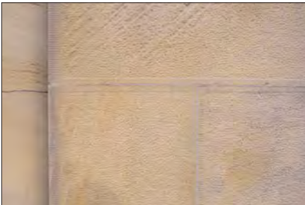
Limestone - A sedimentary rock; used for building walls, window sills and lintels, ornamental stone trim, and sculpture.
