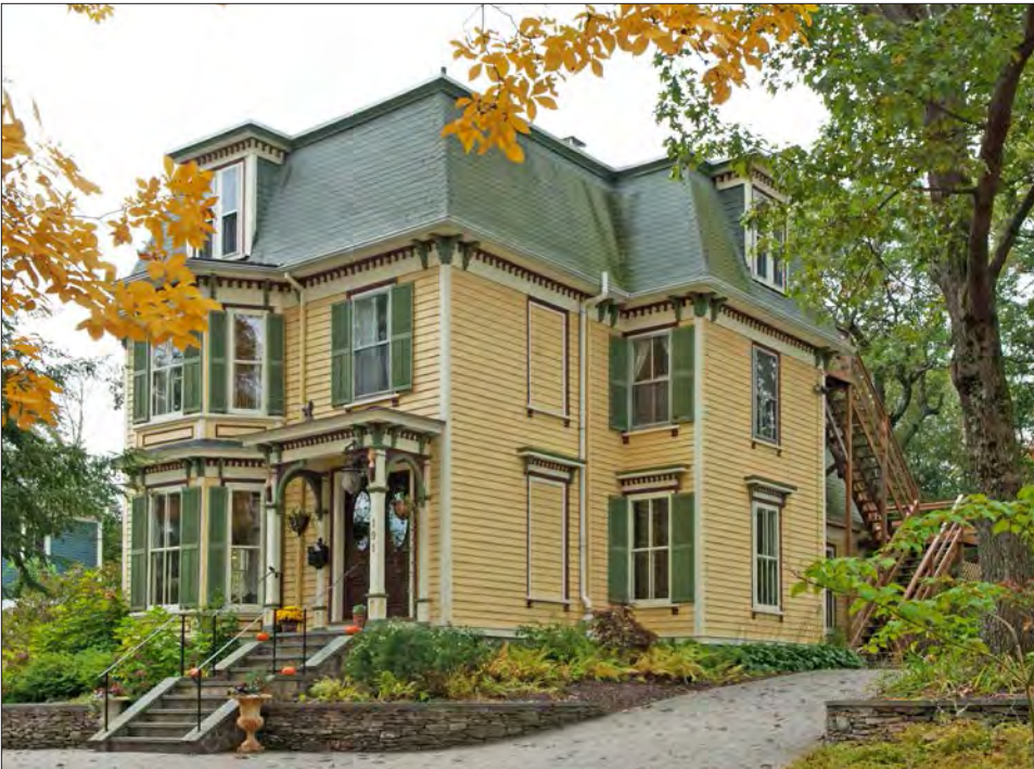
This Second-Empire house in Auburndale features a mansard roof, with heavy bracketed eaves, prominent dormers, elaborate window hood moldings and tall narrow windows.
