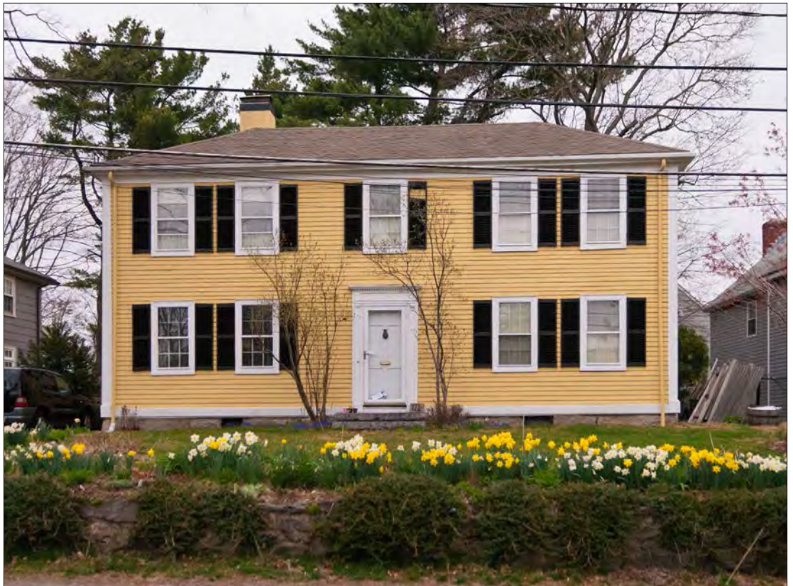
This Federal-Style house in Chestnut Hill demonstrates the symmetrical plan, minimal cornice detailing, and brick chimney common to the style.
