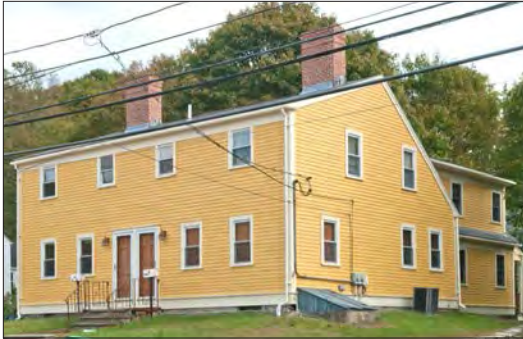
Additions should be deferential to historic buildings, as seen in this example from Newton Upper Falls.
