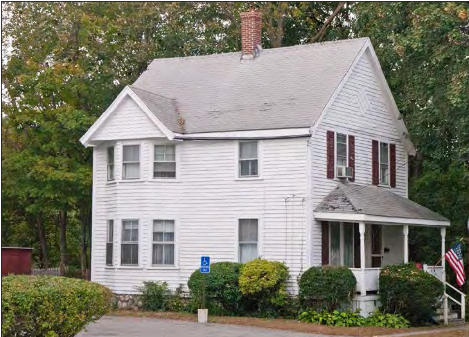
This vernacular Victorian house with Queen Anne detailing in Newton Upper Falls demonstrates the traditional front-gable roof house form, with applied Victorian-period detailing. Note the decorative patterned shingles at the front gable end and over the side elevation bay.
