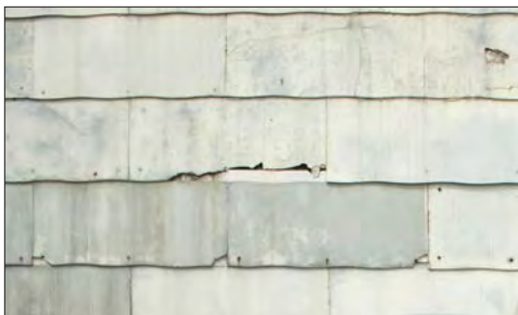
These asbestos shingles are cracked and worn. If replacement is considered, removal should be completed by a trained contractor.
