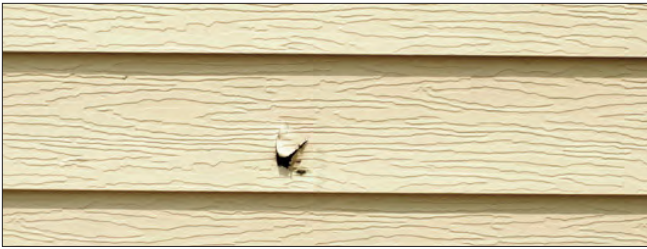
Replacement of this aluminum siding is the best way to repair this puncture. A wood-grained texture is inappropriate.
