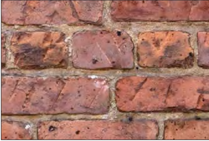
19th Century Brick - A soft, fired-clay, fairly regularly shaped building component; often with color and surface variations; used primarily in walls, piers, foundations, chimneys and exterior pavers.
