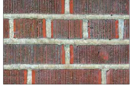
Wire Cut Brick - A dense, fired-clay, regularly shaped building component; with a ridged surface; used primarily in 20th century building walls and chimneys.
