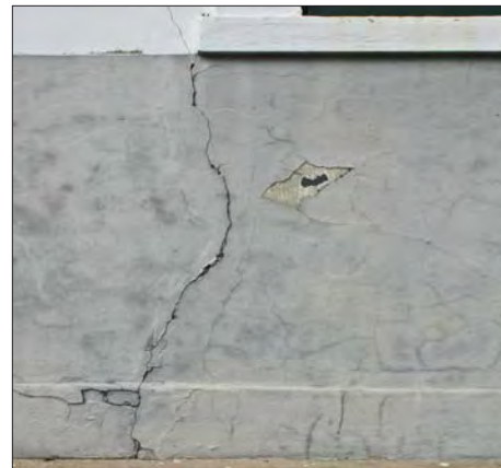
The crack from the window sill might be a sign of building settlement. Review wall for other signs of movement or settlement. Repair crack and apply a lime-based paint for a uniform appearance.
