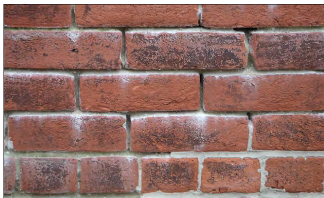
The mortar joints between the bricks has deteriorated, particularly at the vertical joints, increasing the potential for moisture infiltration. The area at the lower right corner of the photograph has been recently repointed and mortar has been smeared over the surface of the brick rather than tooled. To maintain the historic appearance, it is recommended that the replacement mortar match the historic in appearance, color, texture, hardness and joint profile.
