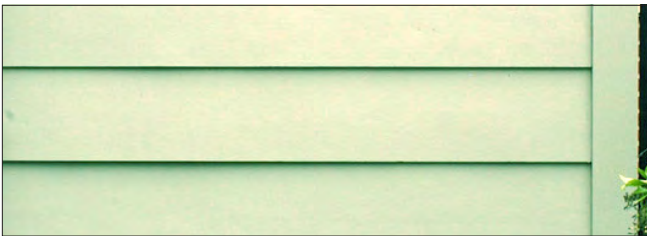
Fiber-cement siding material is an economical alternative for an addition to a historic building. It can be painted to match the existing paint scheme.
