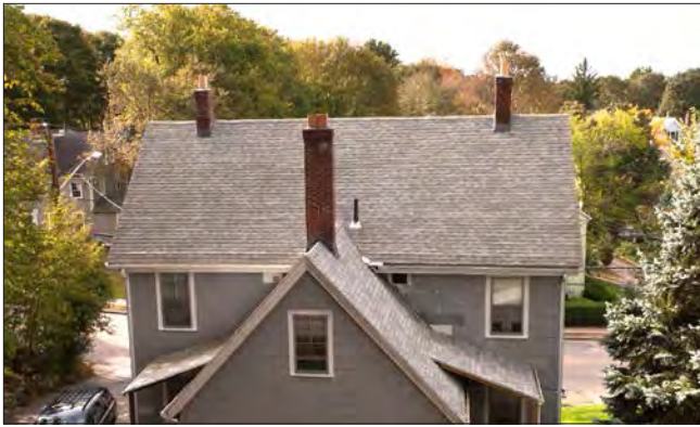
Asphalt shingles are a common 20th century building material, for both roof replacement and new construction.
