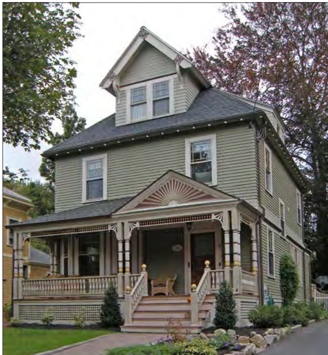
The scale, detailing, and roof forms of historic porches - such as this Queen Anne example in Newtonville - helped define the architectural style of the house and the overall feel of the streetscape. These attributes should be carefully considered when designing new porches in a historic setting.
