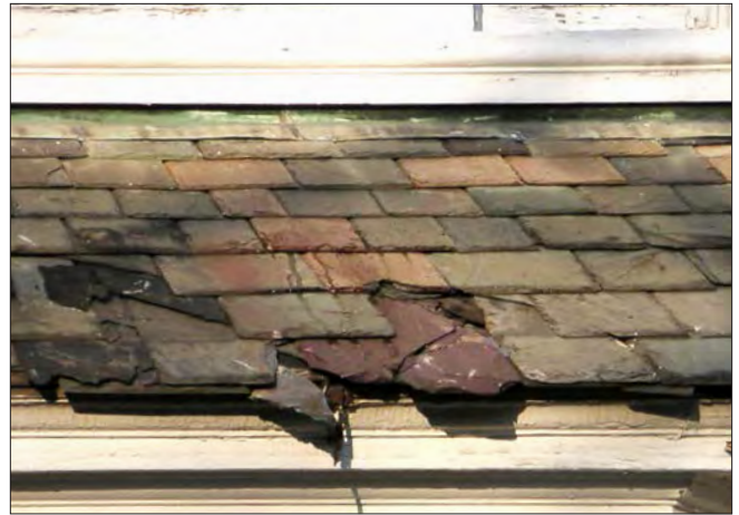
Slates are cracked, dislodged and missing. Some of the surfaces are delaminating. Approximately 25 to 30 percent of the slates on this roof are either missing or damaged. Given the pervasiveness of the problems, considering roof replacement would be appropriate.
