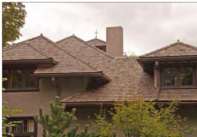
Wood shingle roofs can be applied in a variety of decorative patterns and configurations. This example includes alternating rows of scalloped and square-butt shingles.
