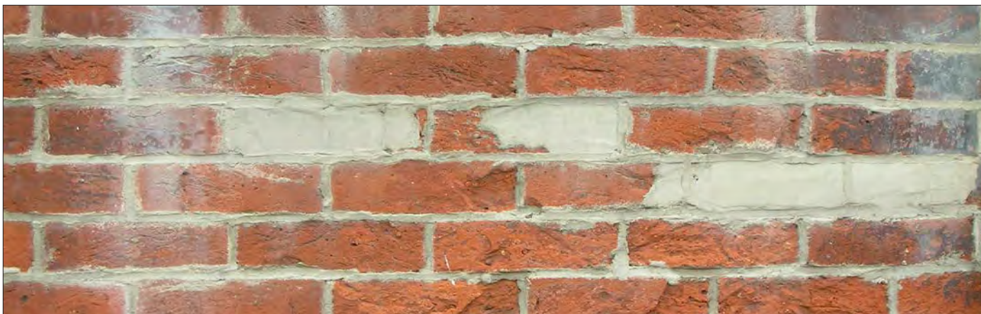
The rough texture and uneven surface suggest that an overly aggressive cleaning method was used. Stucco patches replace bricks and efflorescence, a powdery white substance, can be seen on the surface.
