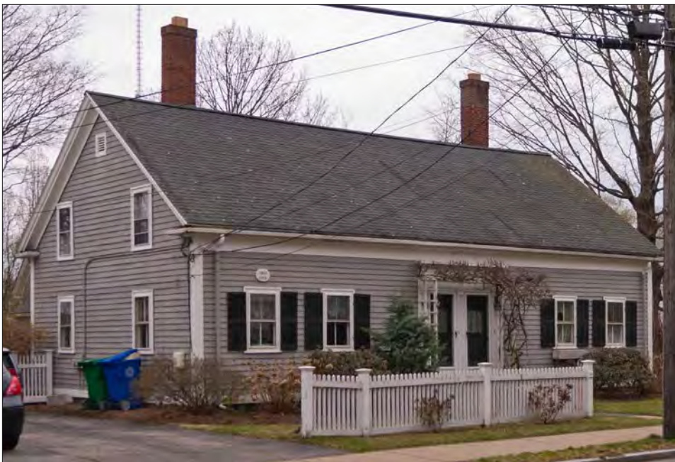
This multi-family residence in Newton Upper Falls demonstrates the simple side-gable roof and symmetrical plan (including paired central entrances) typical of Newton's early-19th century mill-housing type. It also includes simplified Romantic (Greek Revival) details, such as the gable-end returns.
