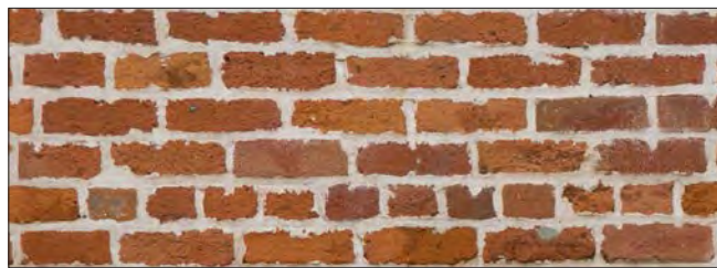
This photograph illustrates an inappropriate repointing of historic brick. A saw was used to cut-out the joints during repointing, extending the vertical joints. In addition, both the vertical and horizontal joints have been widened.
