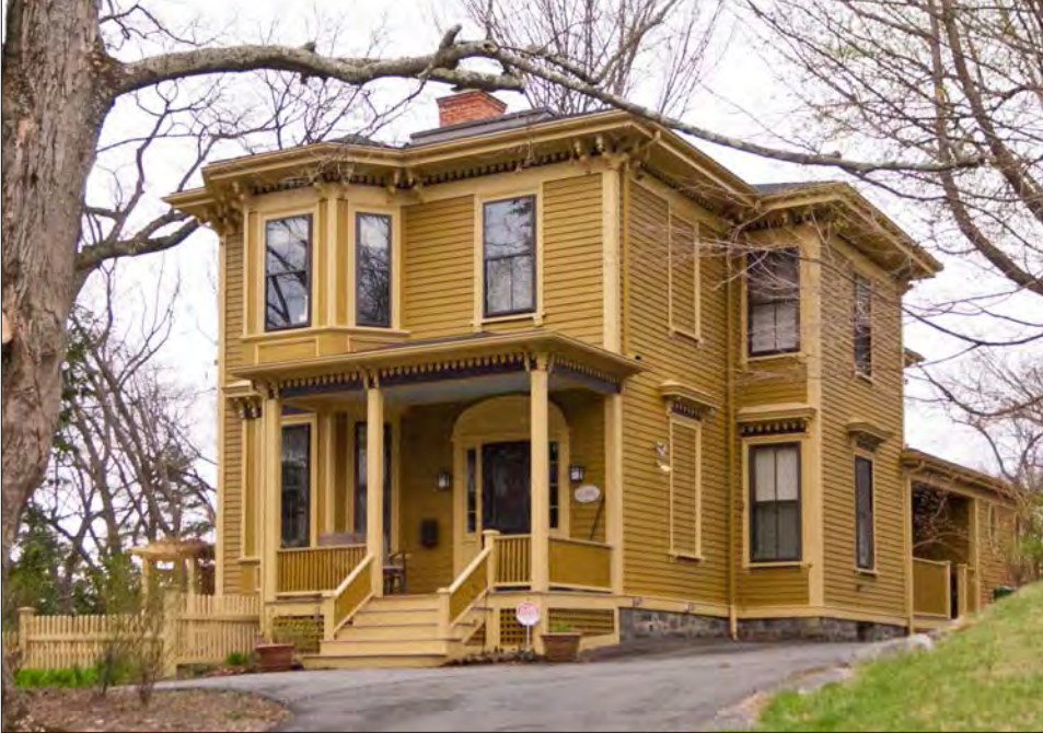
This Victorian-Era house in Auburndale features common Italianate characteristics, including the low-pitched roof with heavy bracketed eaves, tall narrow double-hung windows and elaborate wood window surrounds.
