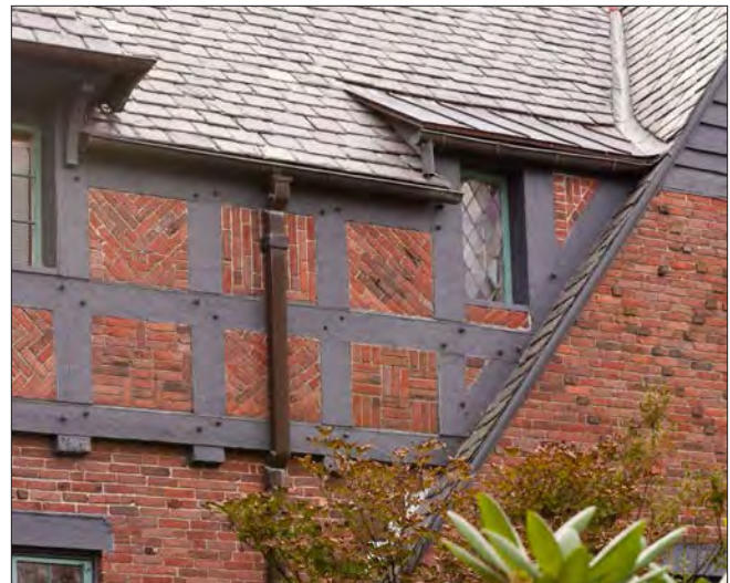
This Tudor Revival house in Chestnut Hill includes a variety of exterior wood elements, including half-timbering, decorative wood brackets, wood lintels and painted wood siding at the gable end.
