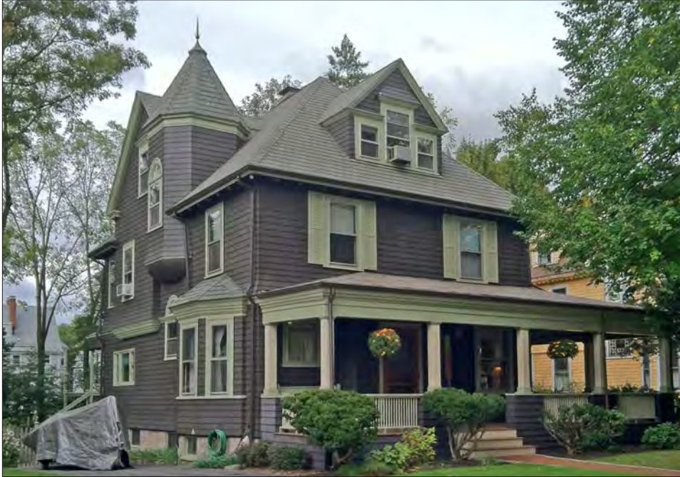
This house, located in Newtonville, demonstrates the steeply pitched, irregular roof, full-width porch that wraps around the side elevation, and prominent turret that are common features of Queen-Anne homes.
