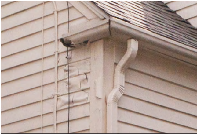
Paint problems at exterior woodwork are sometimes the first indication of an underlying moisture problem. The paint below the end of the gutter is peeling off the siding. Repairing the gutter and verifying that storm water is draining through the downspout is recommended prior to repainting.
