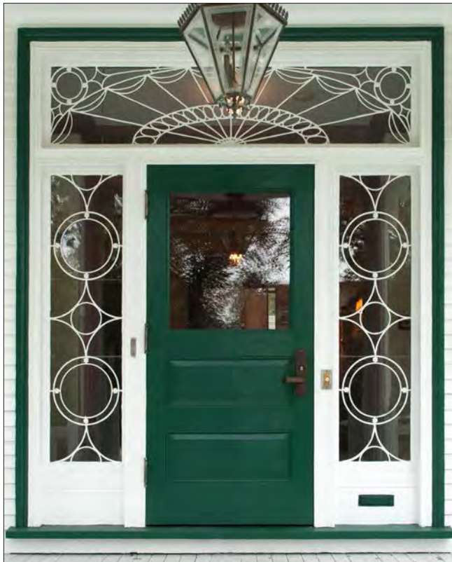
This single-light wood-paneled door has a highly detailed and decorative transom and sidelight.
