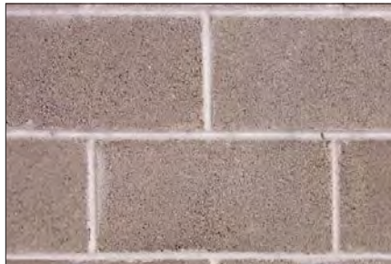
Concrete Block - A structural building material made by mixing water, cement, sand and aggregate, placing the mix in forms and hardening; commonly used for foundations, walls and piers.
