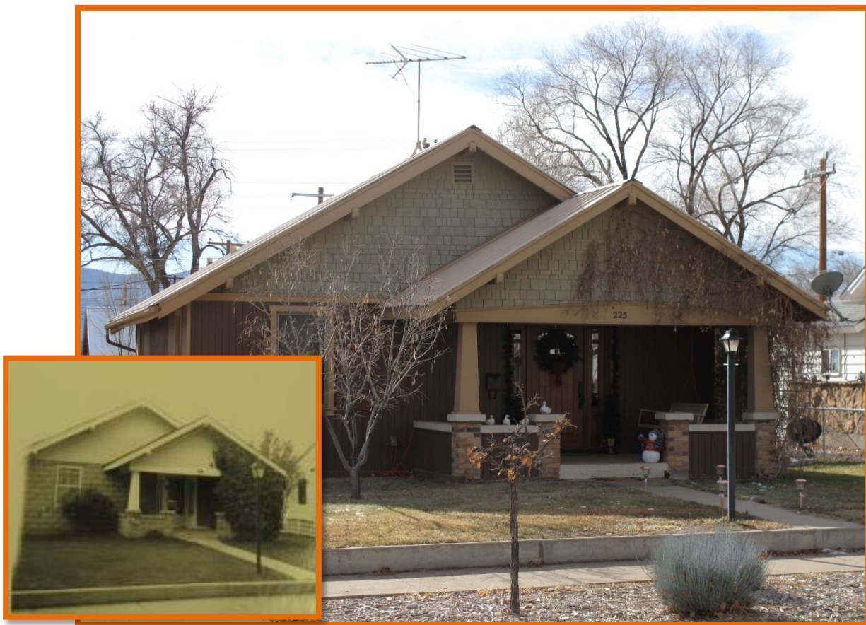
Photograph 12: A historic photo from the Montezuma County Assessor Records shows how this bungalow style house at 225 E Montezuma looked before the concrete block was covered.
