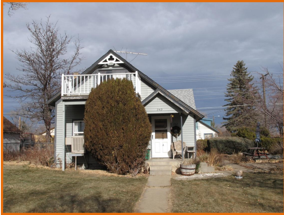
Photograph 5: The oldest building in the survey is the home at 242 East Montezuma, built about 1900.
