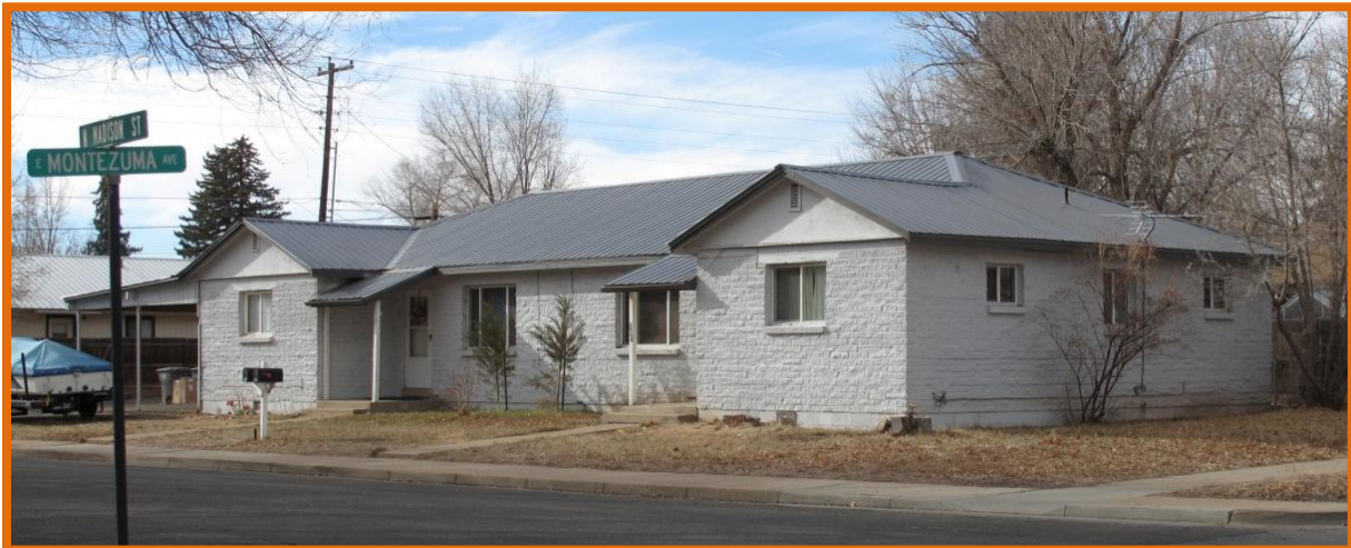
Photographs 10-11: These photos illustrate two versions of the ranch form. The house in the top photo is at 546 E. Montezuma and the house at the bottom is at 137 N. Madison.
