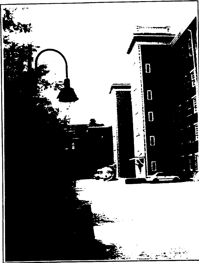
Figures 28, left and 29, below show the relandscaped western portion of the Mill Yard. The surface is packed crushed stone. Oak trees, lamp fixtures, and bollards screen Mill No. 8. The shrub planting, around the sluice gate hoist includes burning bush and helps screen the view of the eastern portion of the Mill Yard. The lower photo shows the Counting House on the right with Mill No. 6 behind it. Except for the NPS orientation sign in front of the Counting House, there is little definition to the eastern portion of the Mill Yard.
