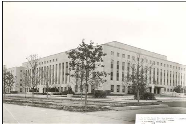
E. Barrett Prettyman Courthouse (formerly U.S. District Courthouse), 1952. National Archives, RG 121-BS, Box 99, Folder E
