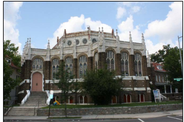
Petworth M.E. Church, Grant Circle and New Hampshire Ave., NW. Photo by EHT Traceries, July 2012.
