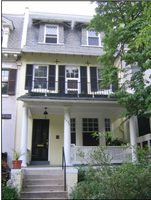
2236 Cathedral Avenue, NW (1909).
