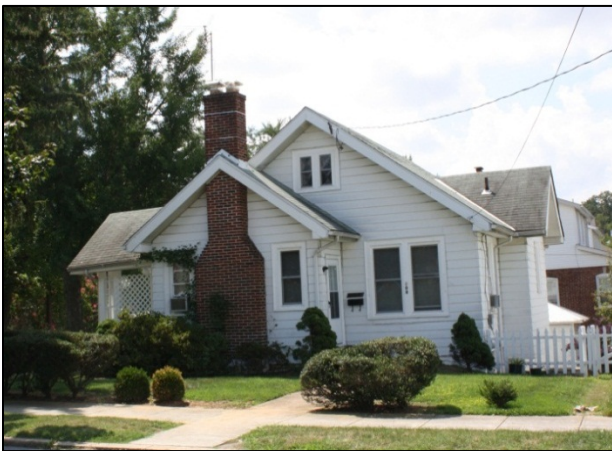
200 Quackenbos Street, NW. Photo by EHT Traceries, July 2012.
