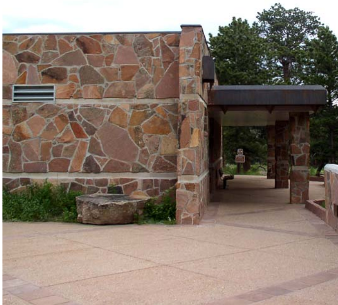
below: Like the visitor center, the comfort station uses random-laid native stone, horizontal lines, and decorative accents. (NPS-ROMO photo)
