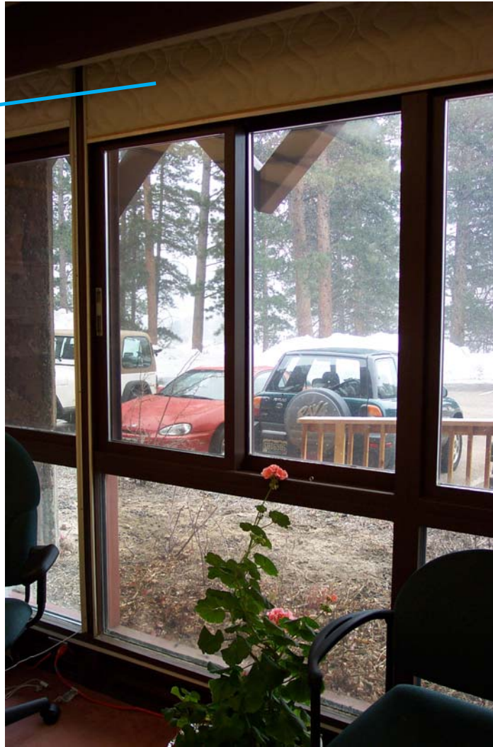
above: Before the rehab, quilted shades provided additional insulation through single-paned windows. (NPS-ROMO photo)
