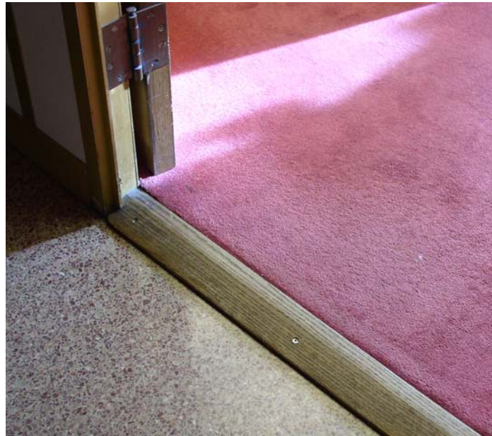
above: Carpeted offices meet terrazzo hallways in most of the office space. Carpets may be replaced but should be low pile and harmonious with the terrazzo. (NPS-ROMO photo)
