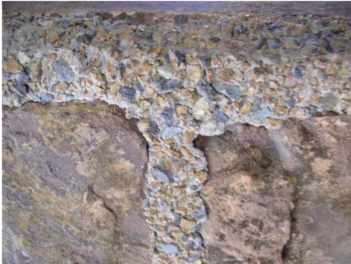
above: The crushed stone in the mortar is an important feature of the masonry on the building (NPS-ROMO photo)
