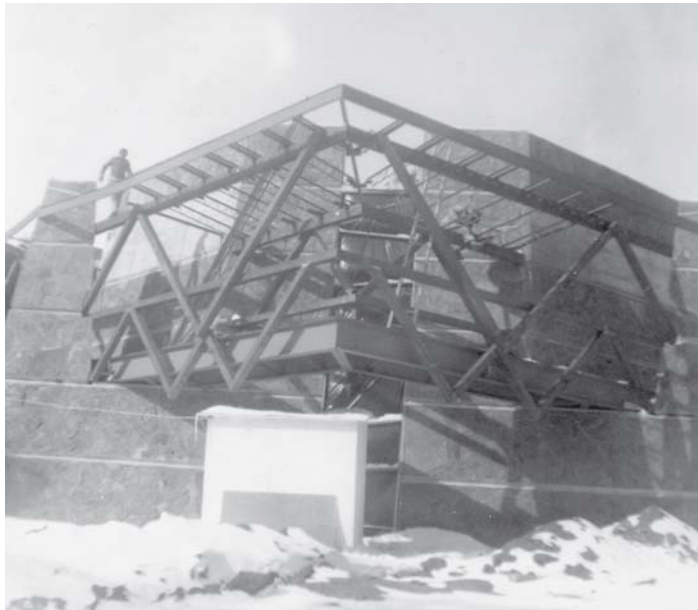
above: Steel tubes form the structure of the auditorium and cantilevered balcony, March 1966. (NPS-RMNP photo)
