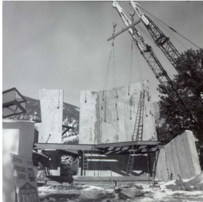
above: Cranes set the auditorium panel. The largest masonry panel weighted 65,000 lbs.
