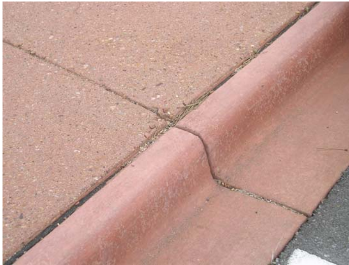
above: The new walkways are exposed aggregate; the curbs are smooth finish.
