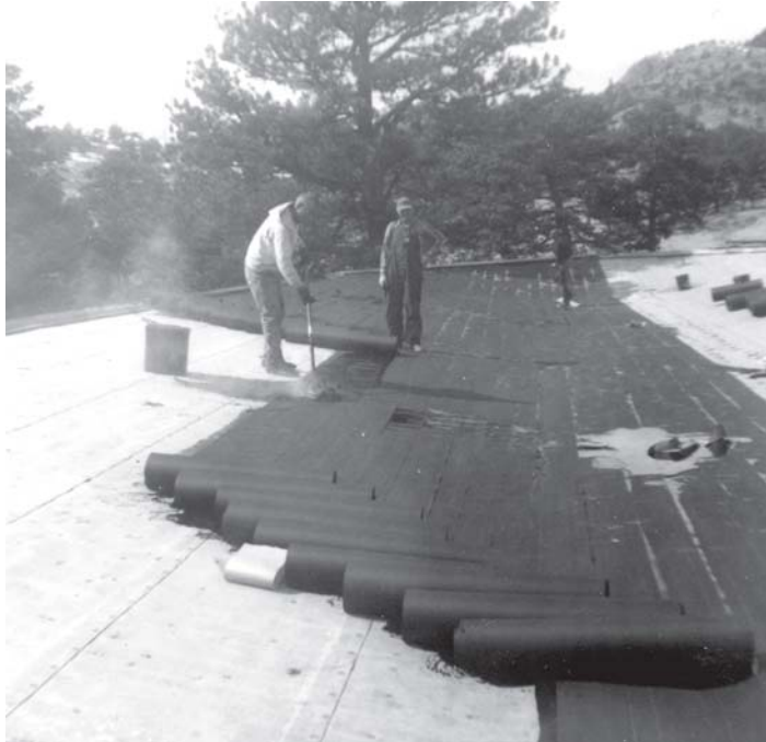
above: Installing the original rolled roof in March 1966. (NPS-ROMO photo)
