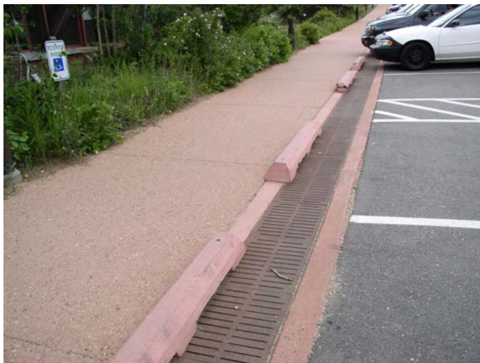
below: The at-grade drain and lack of curb make the handicap parking readily accessible. (NPS-ROMO photos)
