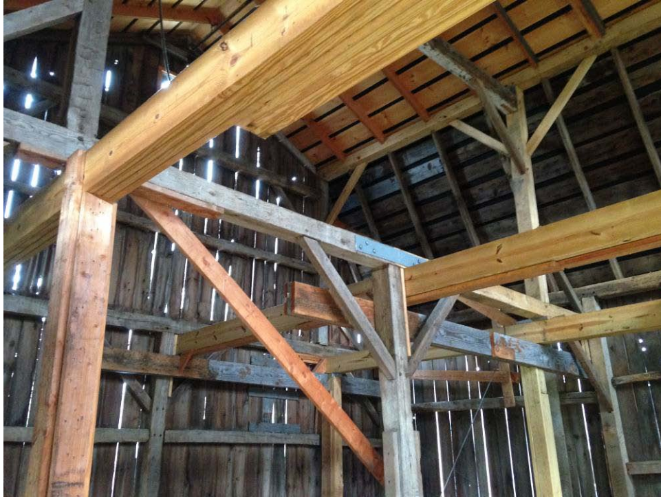
Temporary Shoring for Roof
