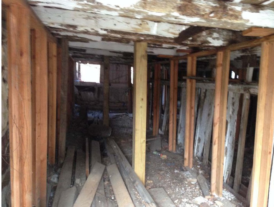
Temporary Shoring at Main Level
