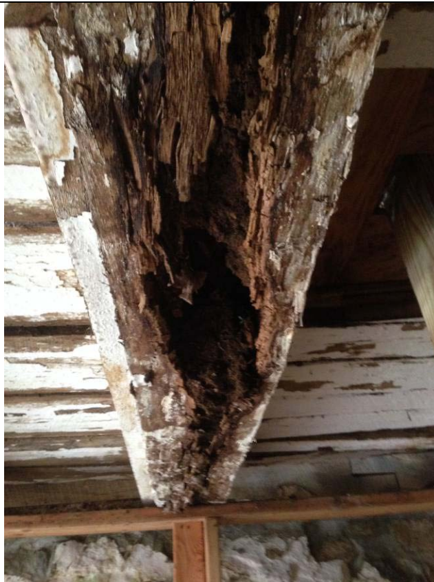
Severely Rotted Main Level Floor Fanning
