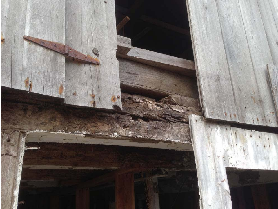
Severely Rotted Main Level Framing
