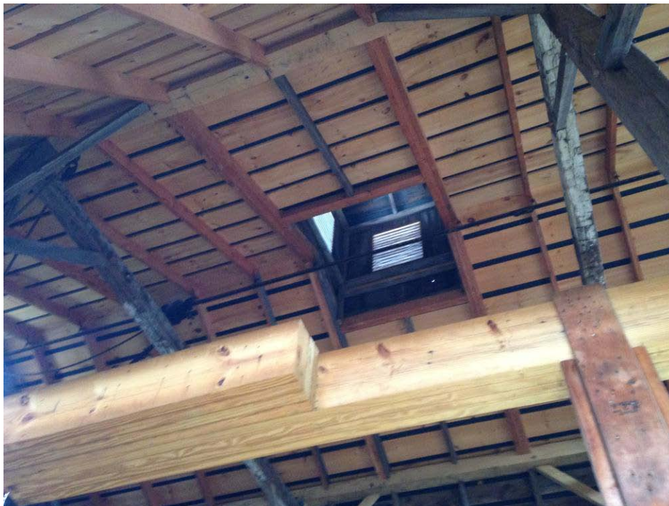
Previously Repaired Roof Framing
