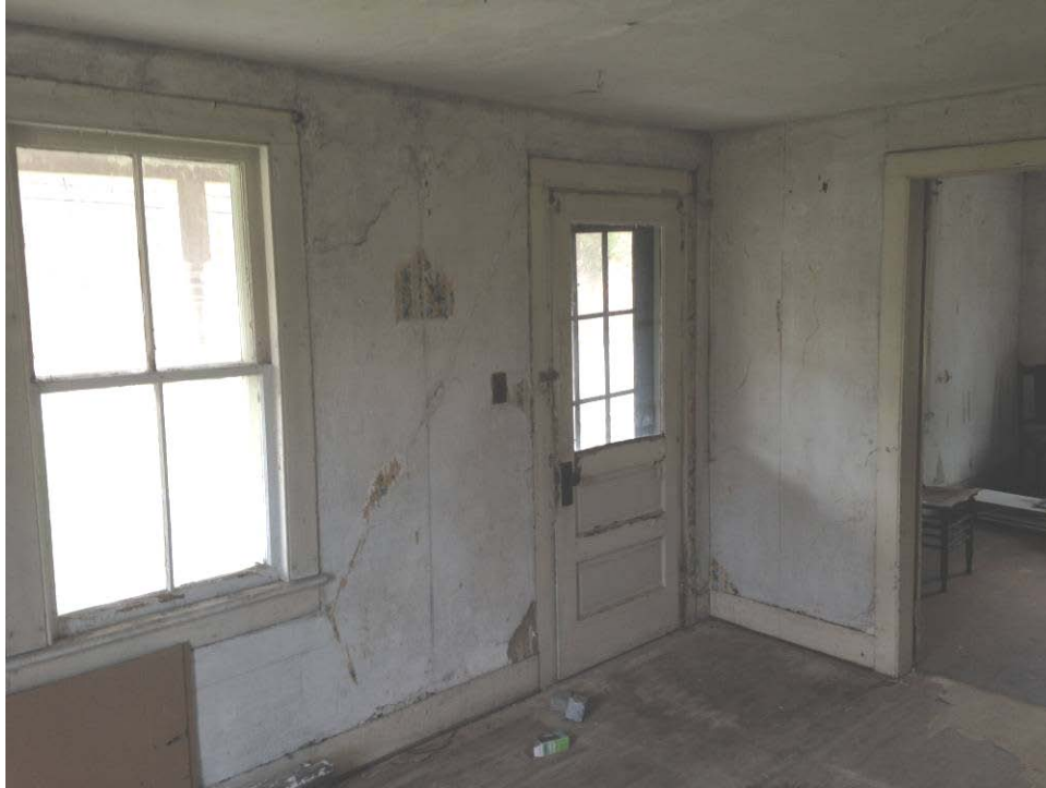
Cracked Wall Plaster
