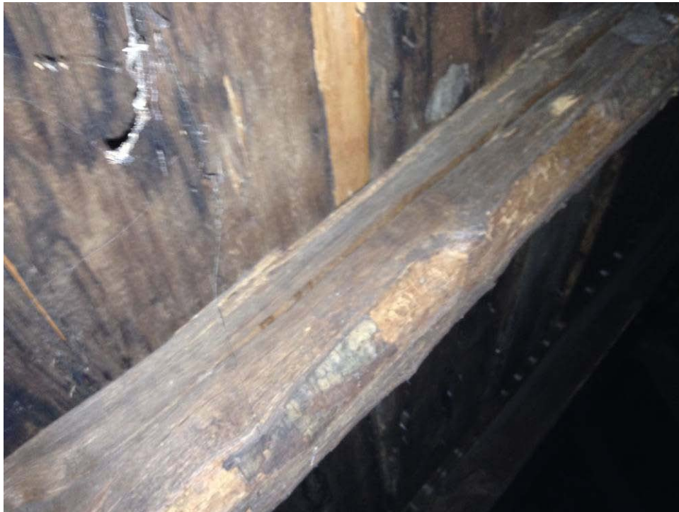
Cracked Roof Rafter
