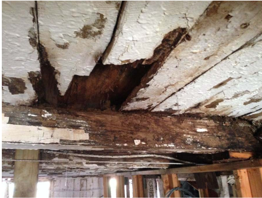
Severely Rotted Main Level Floor Fanning
