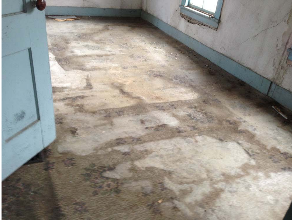
Defective Vinyl Floor Covering
