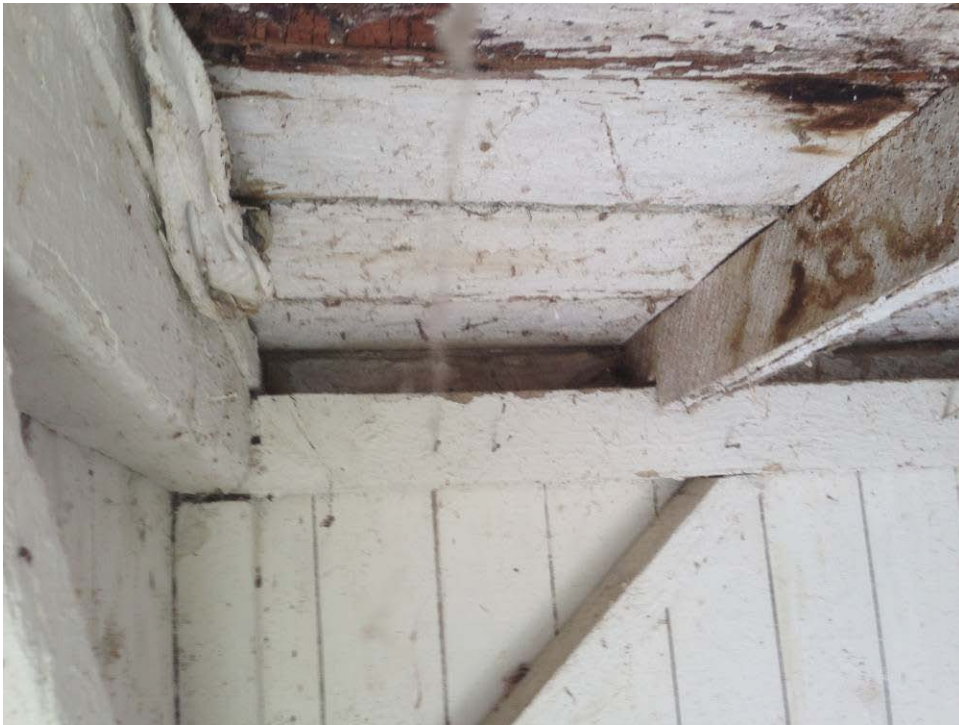
Rotted Roof Framing
