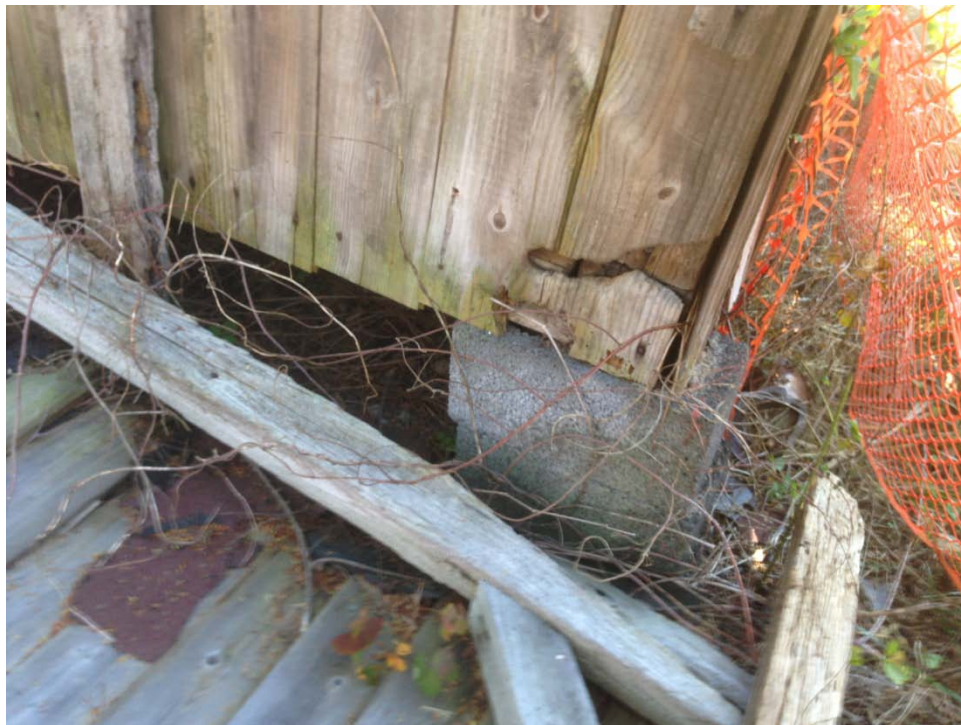
Typical Base Detail with CMU Block
