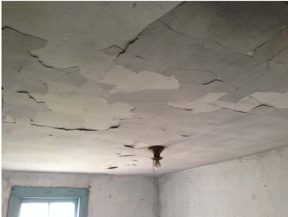
Cracked Plaster Ceiling
