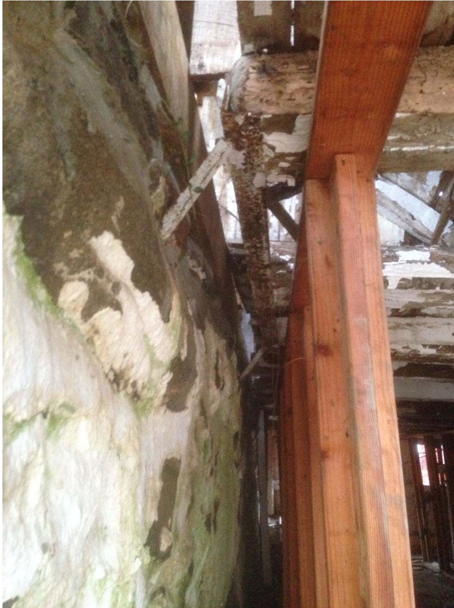
View of Floor Framing Disengaged From Foundation
