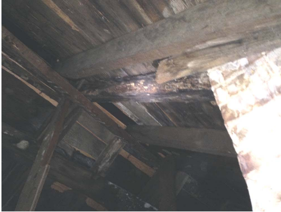
Defective Roof Framing Around Chimney
