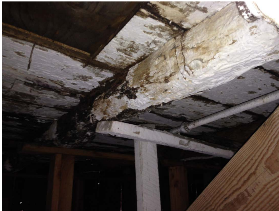
Severely Rotted Main Level Framing
