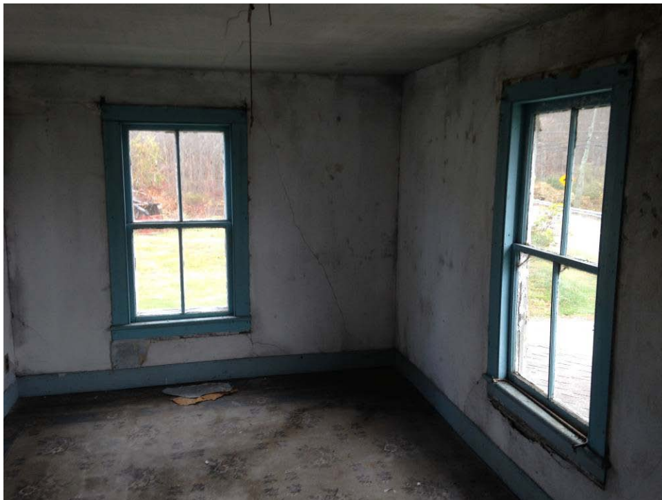
Cracked Wall Plaster
