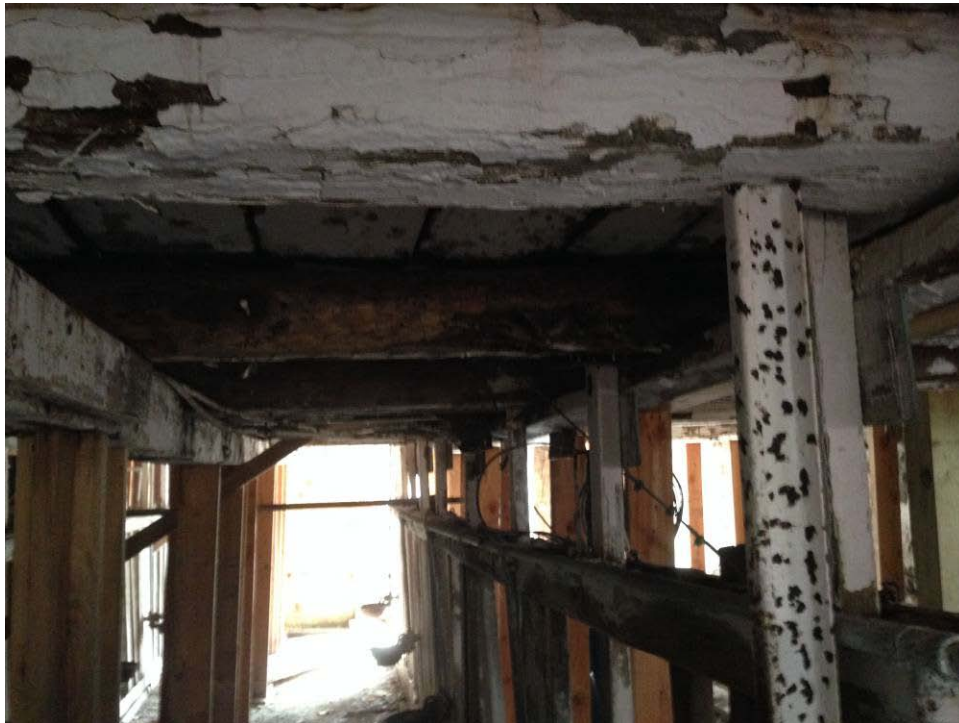
Severely Rotted Main Level Framing
