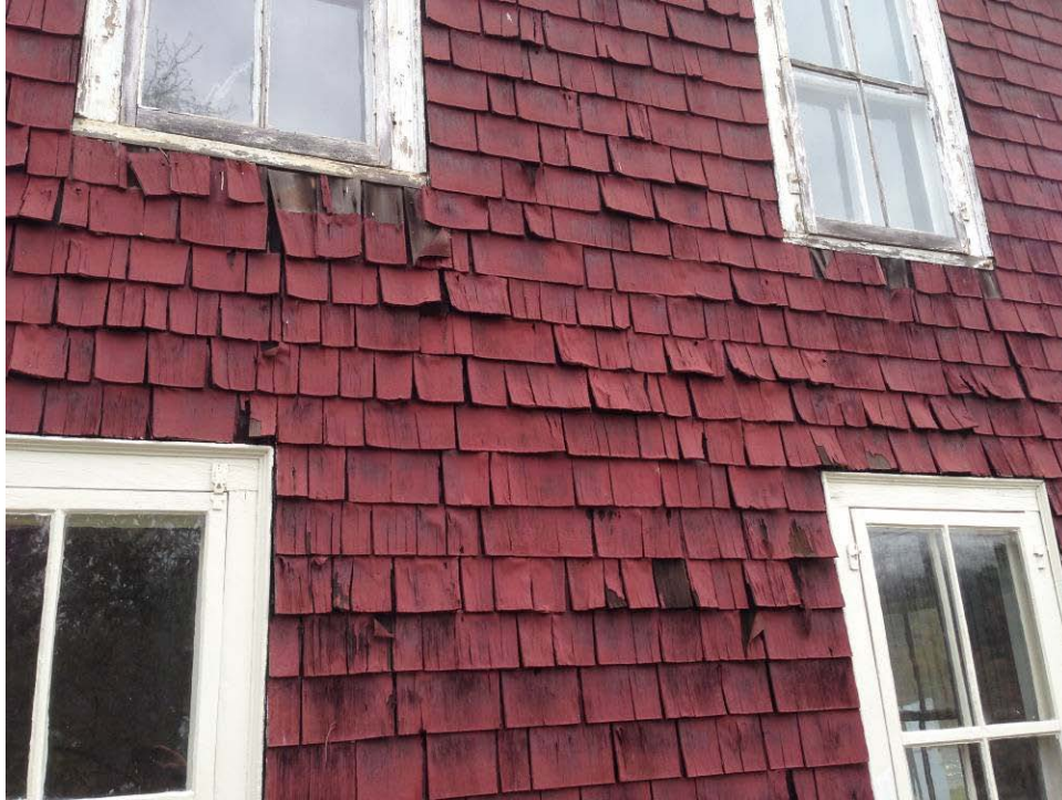
Defective Siding and Deteriorated Window Frames
