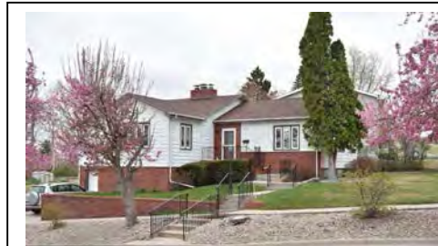
Figure 15. 1902 West Boulevard, April 2015.
