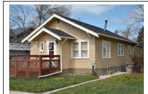
Figure 10. 824 Clark Street, April 2015.
