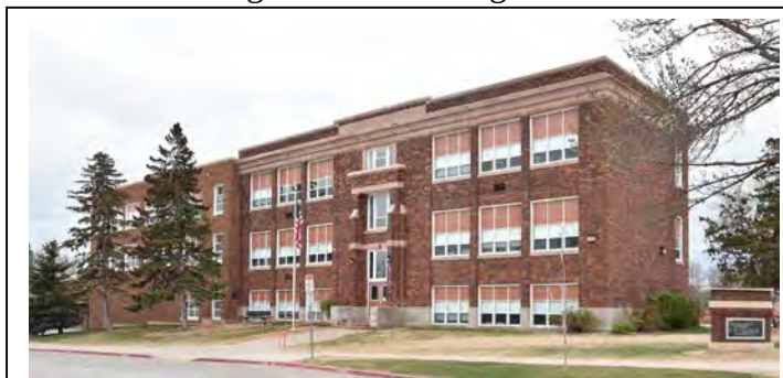
Figure 16. 827 Franklin Street, Woodrow Wilson School, April 2015.
