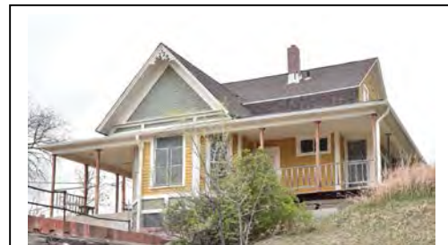
Figure 28. 702 Clark Street, April 2015.
