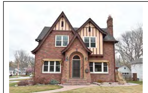
Figure 31. 1404 West Boulevard, April 2015.
