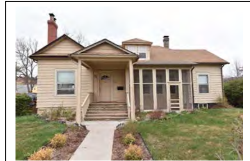
Figure 8. 705 West Boulevard, April 2015.
