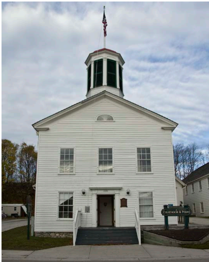
Photo 13. Mackinac County Courthouse, 7374 Market Street, looking north. November 2010.
