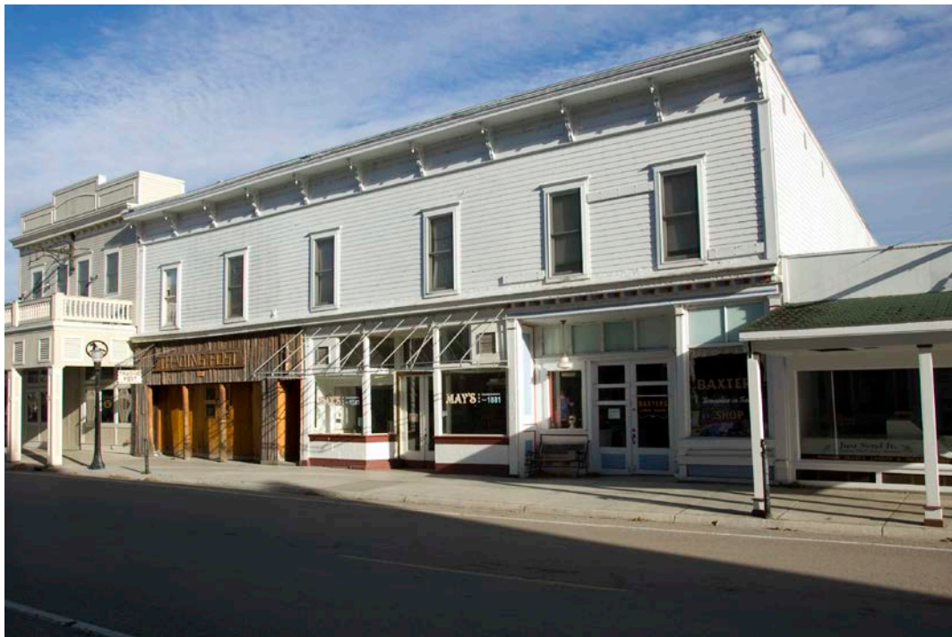
Photo 14. 7347-55 Huron Street, looking southeast. November 2010.
