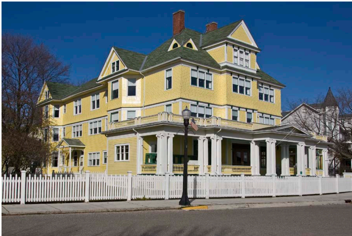
Photo 19. Windermere Hotel, 7498 Huron Street, looking north. November 2010.
