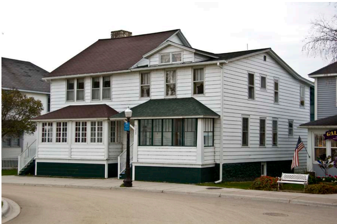
Photo 10. Louis Buisson House, 7573-77 Market Street, looking east. October 2010.
