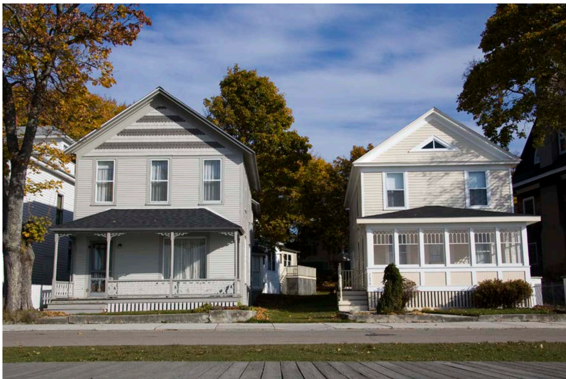
Photo 9. 7664 (left) and 7656 Huron Street, looking north. October 2010.
