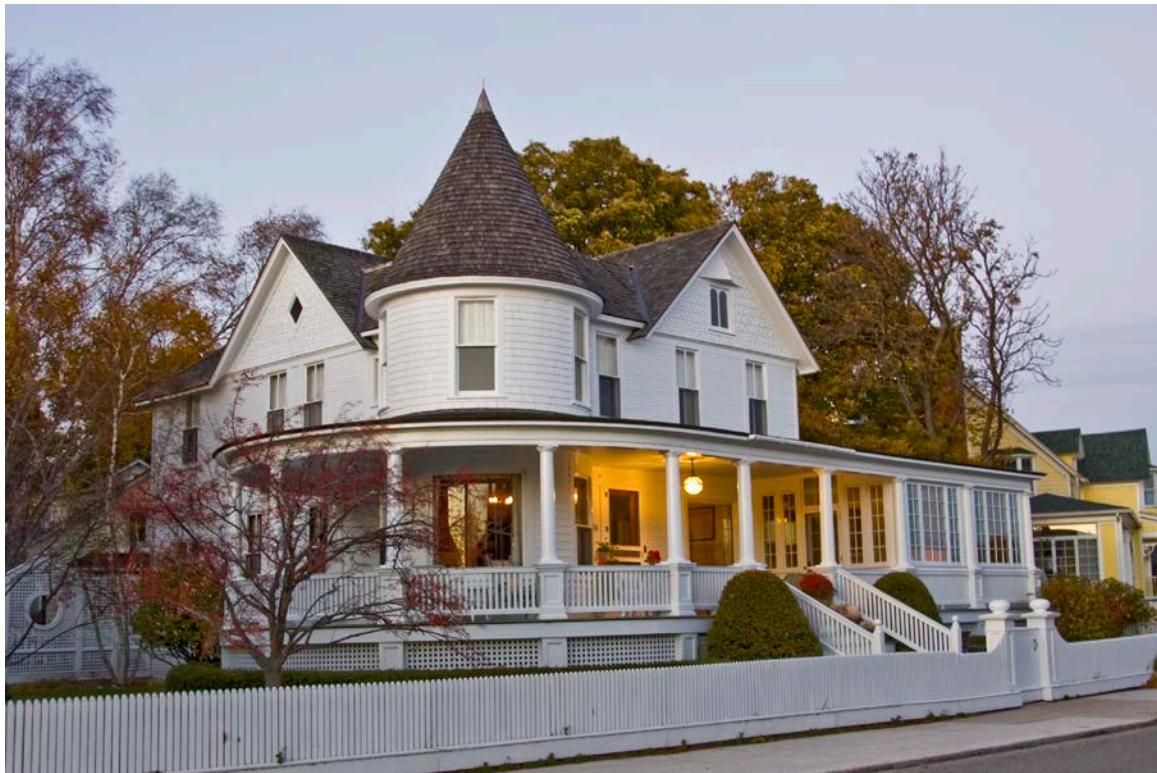
Photo 13. 7566 Huron Street, looking northeast. October 2010.
