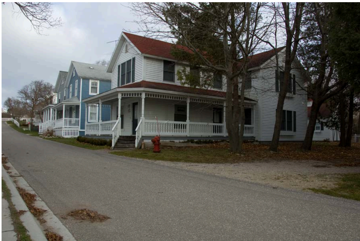
Photo 4. Mahoney Street, looking northeast. November 2010.
