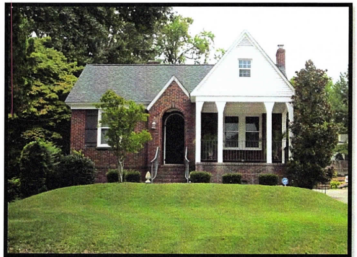
921 Heard Avenue is an example of an American Small House.
