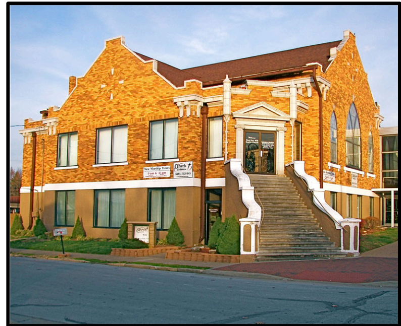
Cast stone is used on this building in details on the entry stair, surrounding entry doors, wall caps, and other wall accents.
