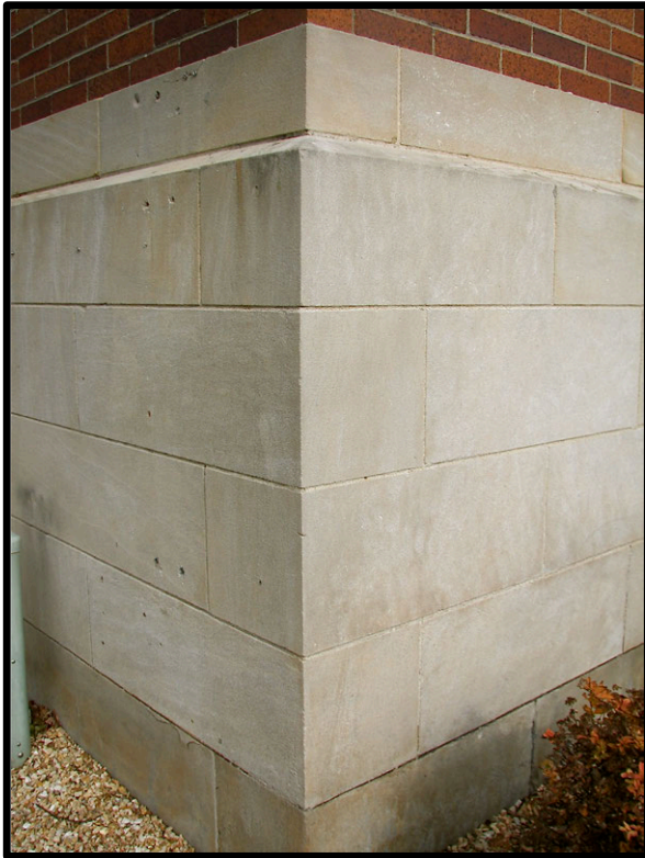
Cast stone masonry foundation on historic County Courthouse building and represents an important architectural characteristic.
