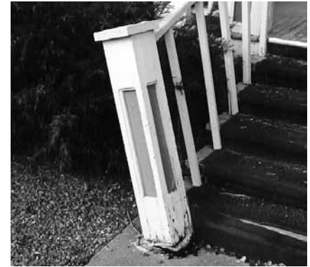
Before: A deteriorated railing should be repaired, not replaced, when feasible.
