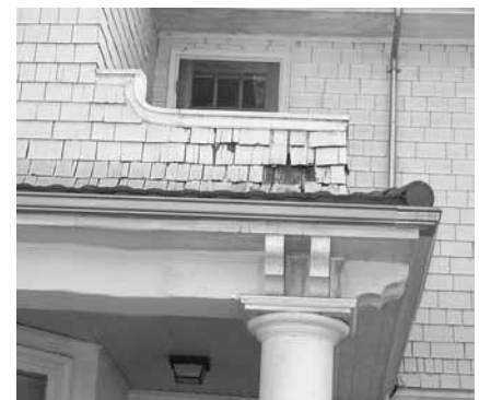
Do not remove damaged materials that can be repaired. In this case, loose shingles may be re-secured while missing ones may be replaced.
