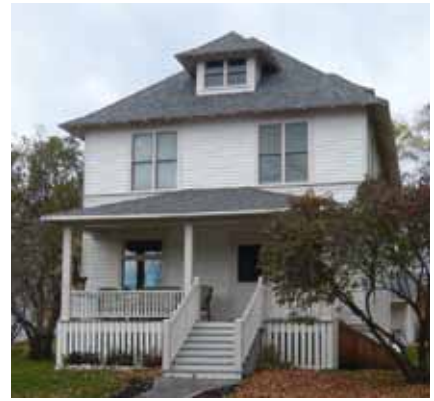
Maintain the existing location, shape, details and posts of an original porch.
