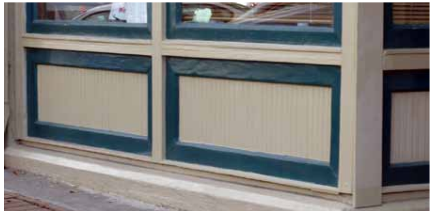
A kickplate, located below the display window, adds interesting detail to the streetscape and should be preserved.
