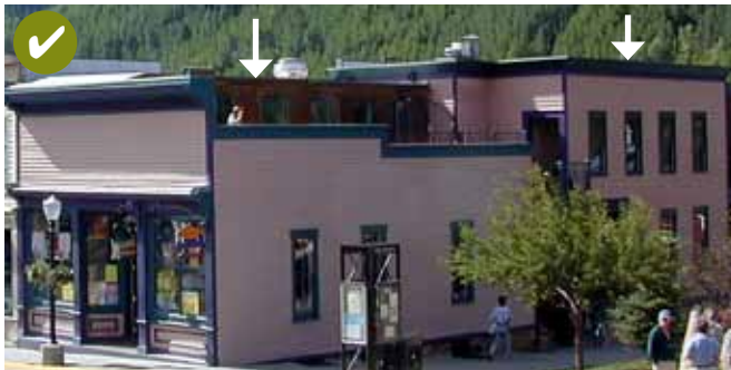
This two-story rear and rooftop addition is compatible with, yet remains subordinate to, the original one-story structure.
