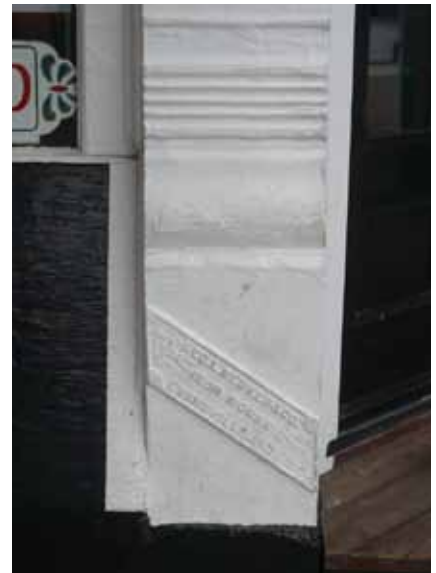
The signature of a Mesker Brothers cast iron post is a noteworthy feature of this Downtown foundation.
