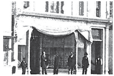
This traditional awning on the historic Opera House is operable to help regulate internal climatic conditions.
