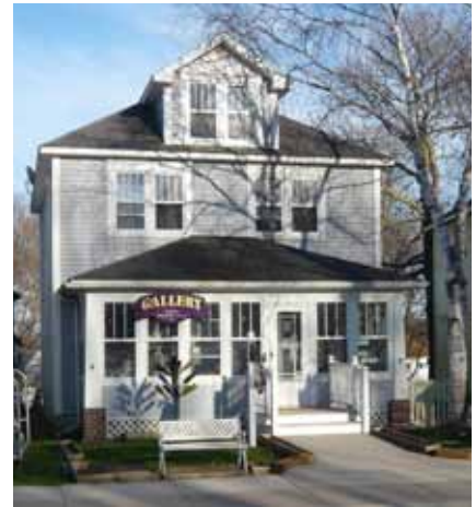
Many examples of adaptive reuse occur throughout downtown.
