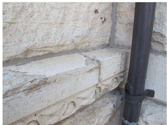
Deteriorating stone
