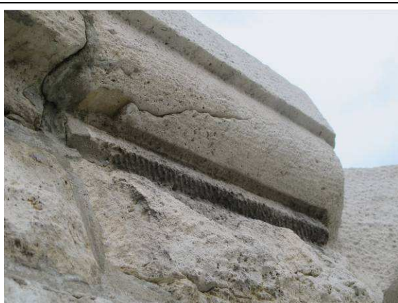
Spalling limestone
