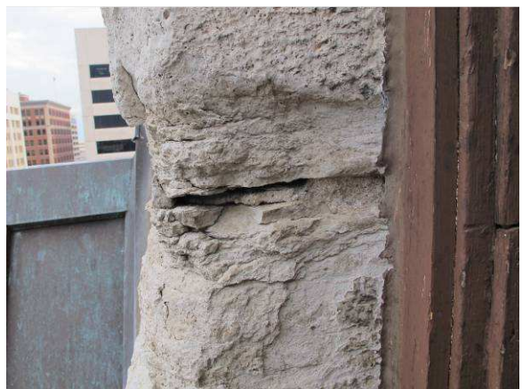
Delaminating limestone
