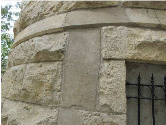
Parging on limestone
