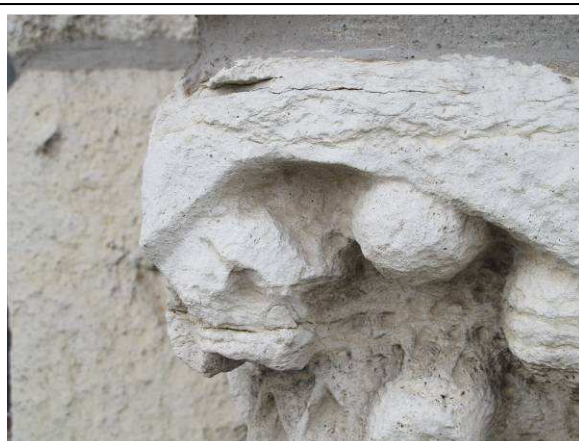
Loss of detail in carving
