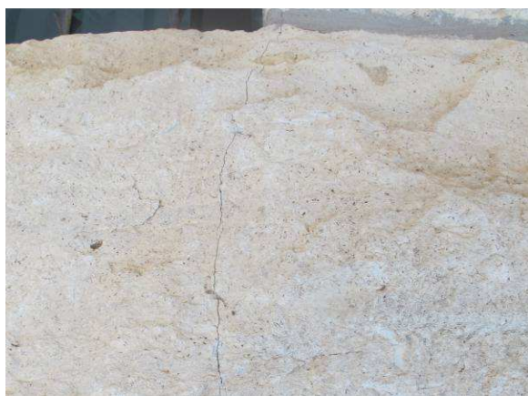
Crack in limestone
