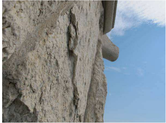
Spalling stone
