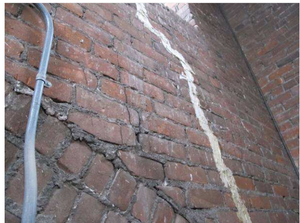
Close up of repaired crack
