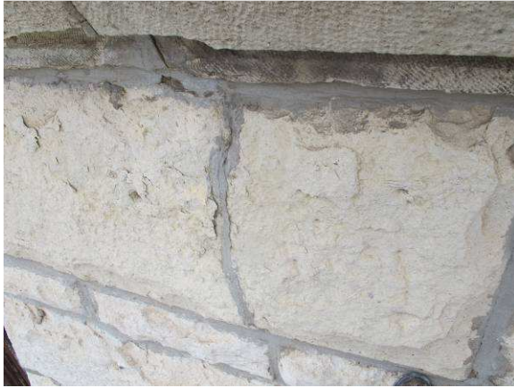
Separating mortar joints
