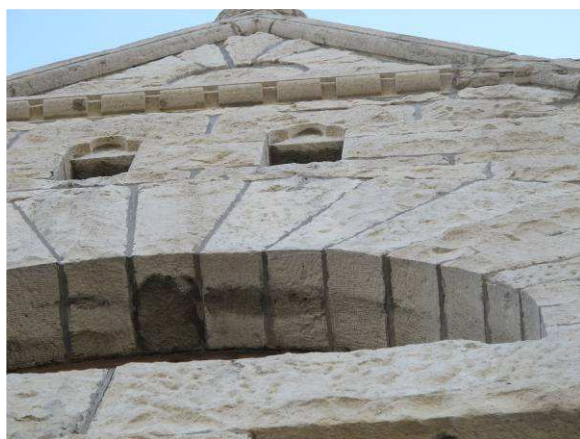
Upper wall above main entry
