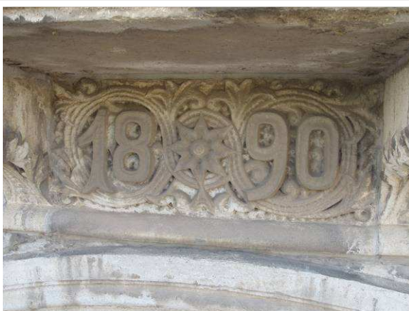
Discolored carved date of construction
