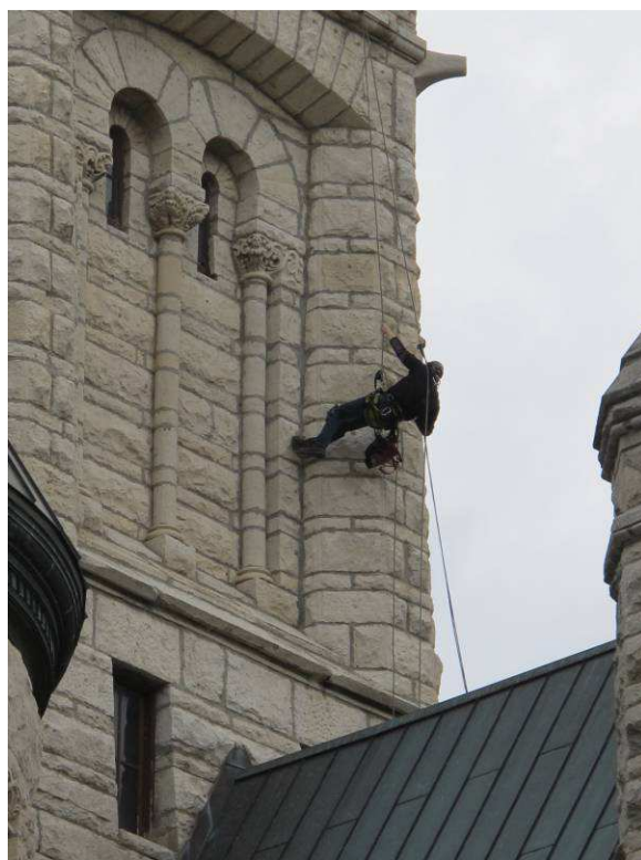
First drop on west face almost complete
