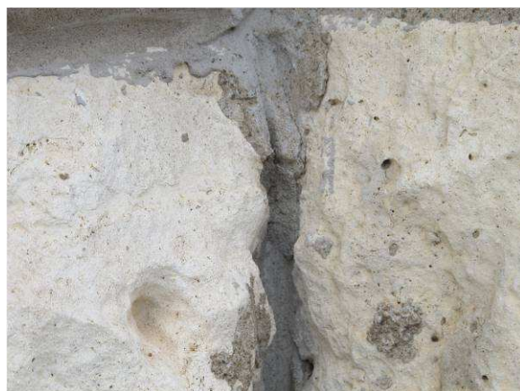
Missing mortar
