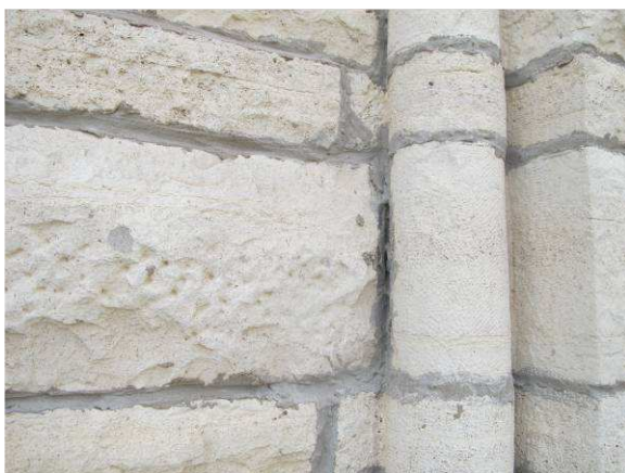
Missing mortar
