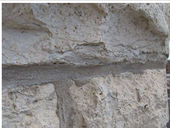
Deteriorating limestone
