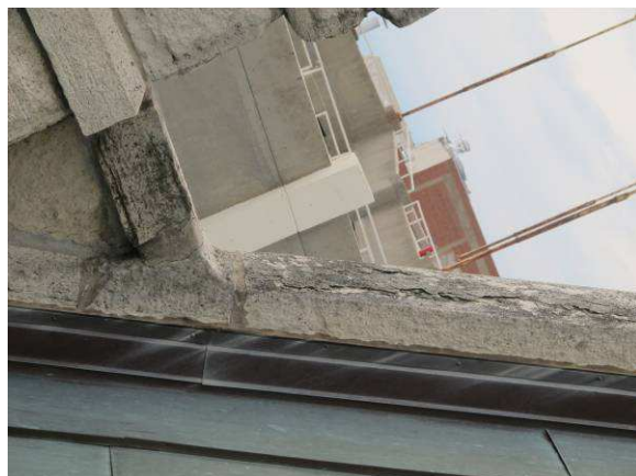
North side of east roof peak
