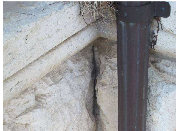
Missing mortar
