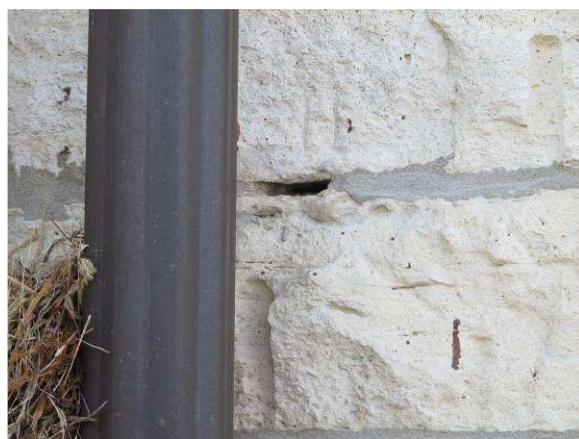
Missing mortar
