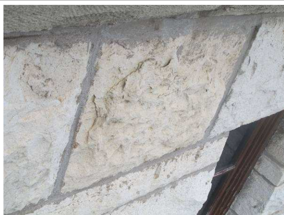
Spalling stone
