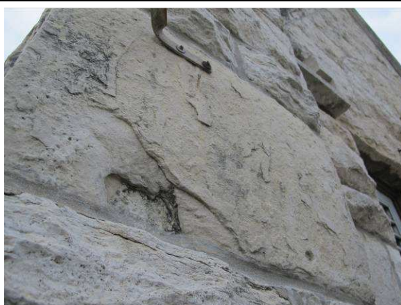
Deteriorating stone
