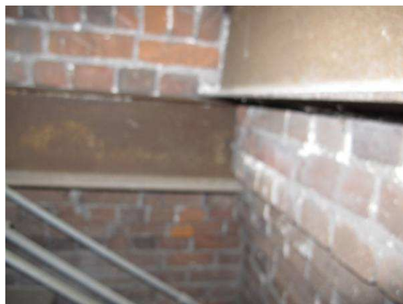
Metal I beams inset in brick
