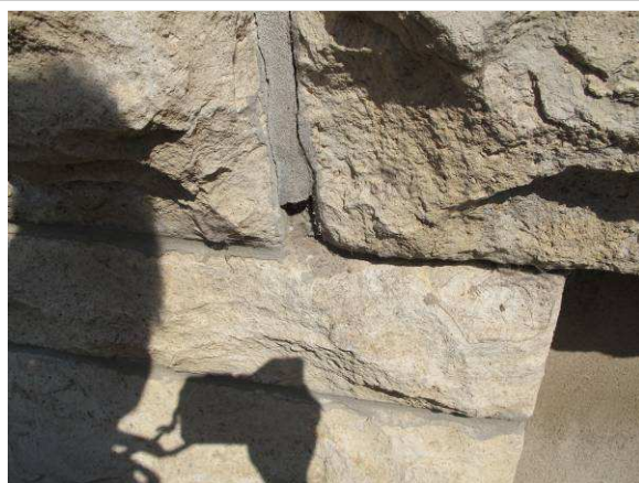
Missing mortar
