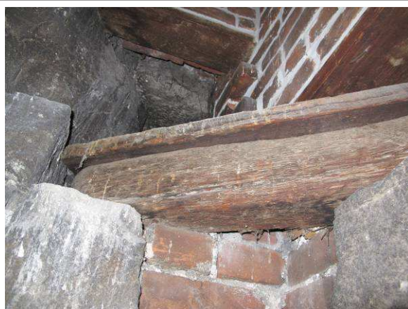
Wood beam at corner
