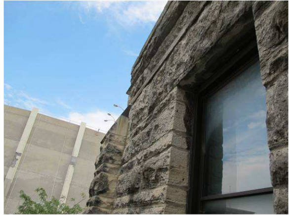
Deposition on limestone
