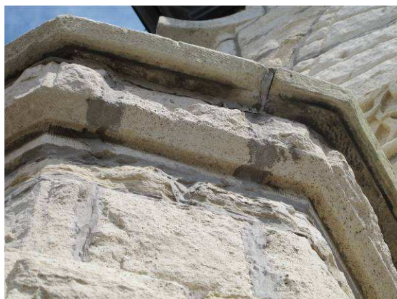
Separating mortar joint
