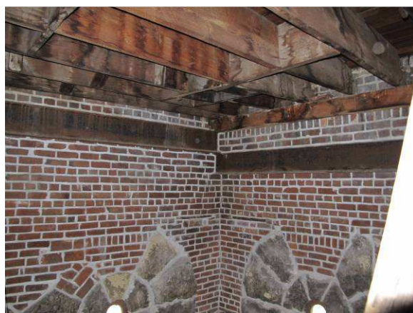
Stone, brick, metal beams, wood beams & joists
