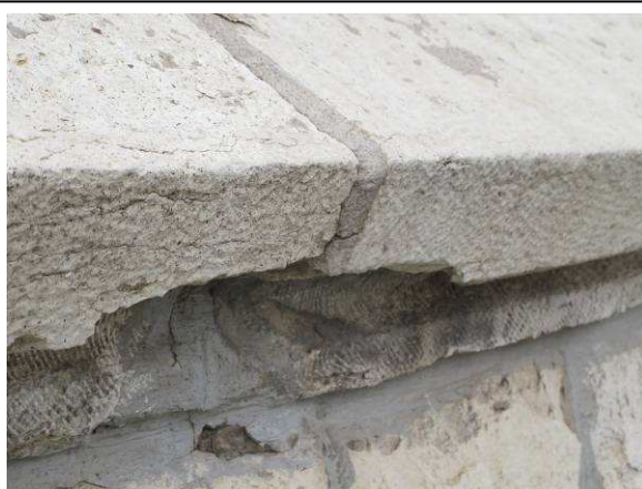
Spalled limestone
