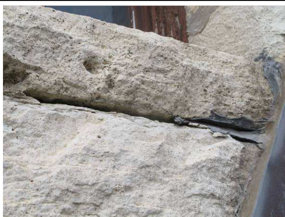
Missing mortar
