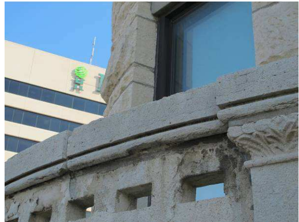
Damaged limestone
