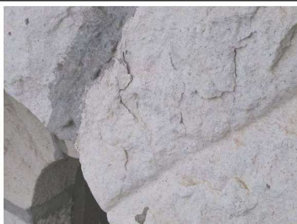
Spalling limestone
