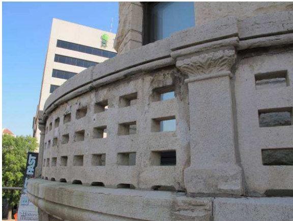
Damaged limestone
