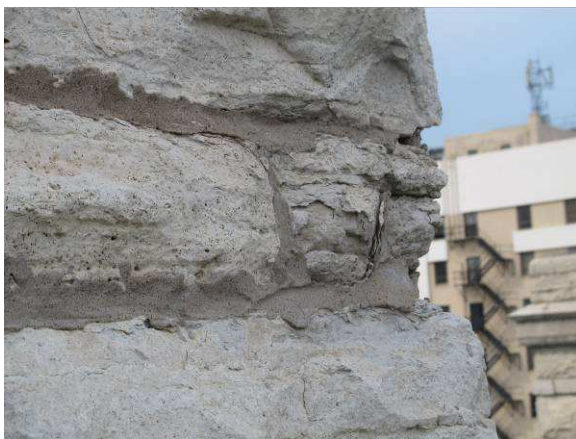
Spalling stone
