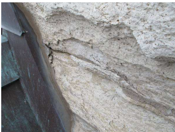
Delaminating limestone
