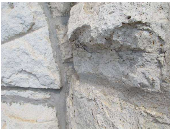
Spalling stone
