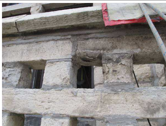
Deteriorating balcony
