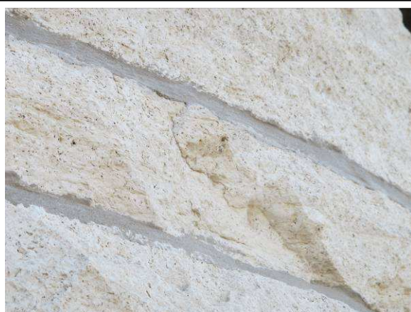
Spalling limestone
