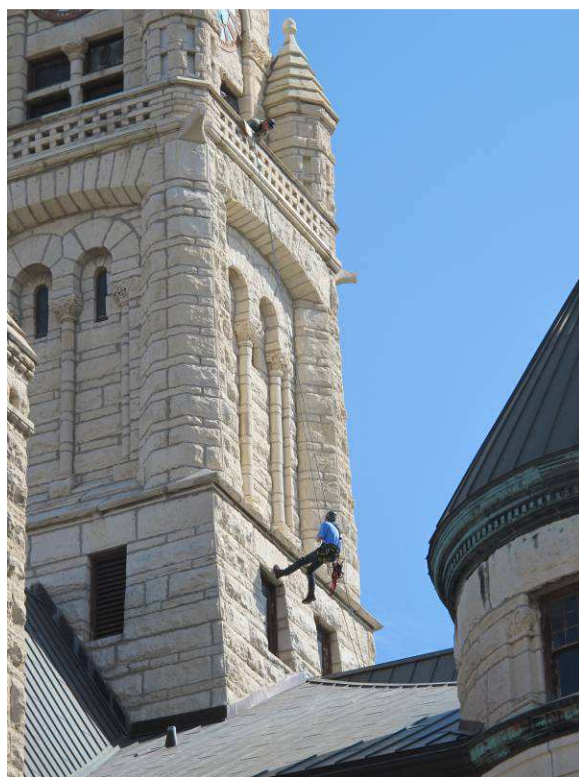
First drop on south face almost complete
