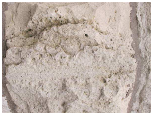
Deteriorating limestone
