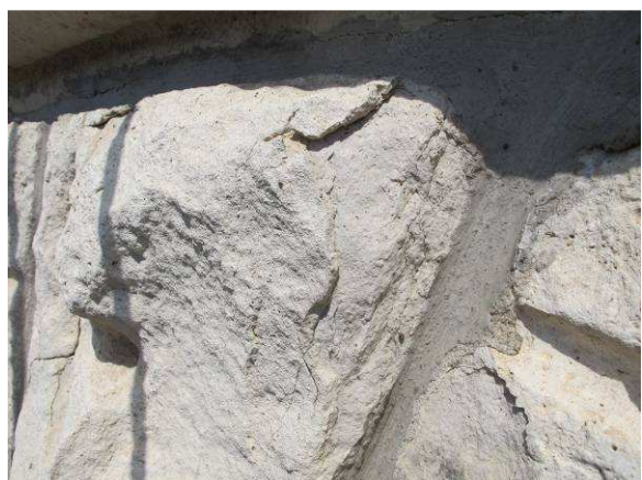
Deteriorating stone
