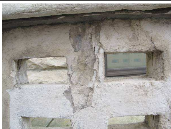
Deteriorating stone
