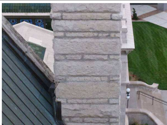
Backside of chimney at south end of bldg
