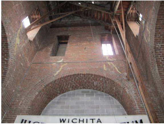
Repaired cracks above arch
