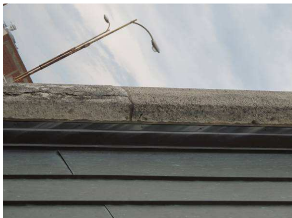
North side of east roof peak
