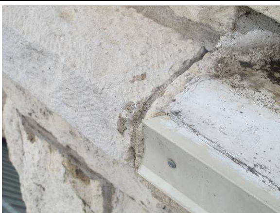
Missing mortar
