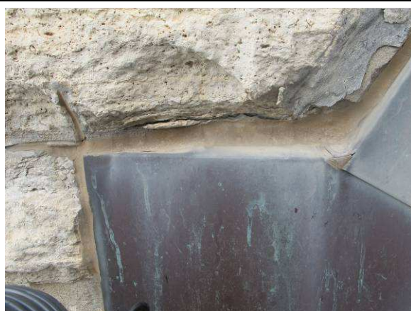
Failed sealant
