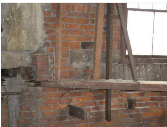
Uncoursed brick and stone
