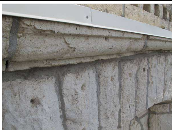
Delaminating stone
