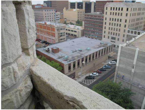
Damaged balcony rail
