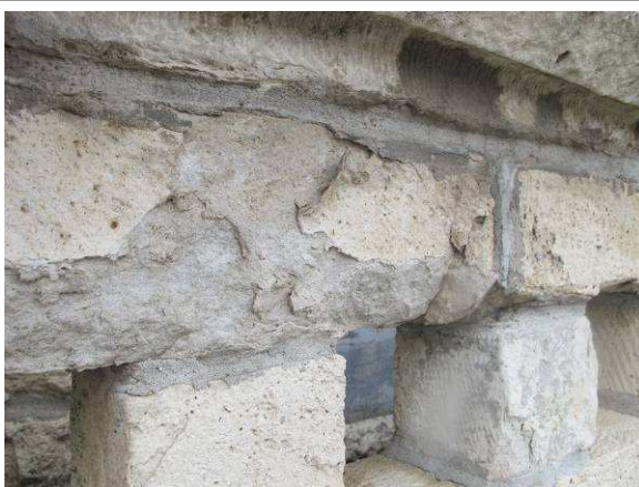
Deteriorated limestone
