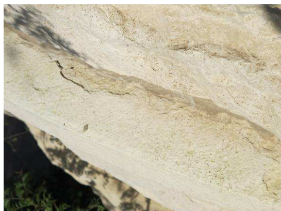
Spalled stone
