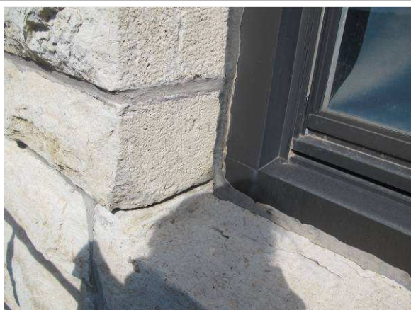
Missing mortar
