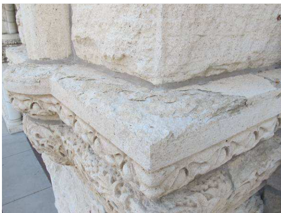
Deteriorating stone
