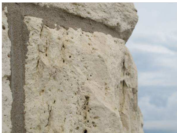
Spalling limestone
