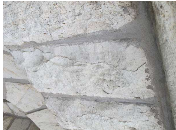
Spalling limestone
