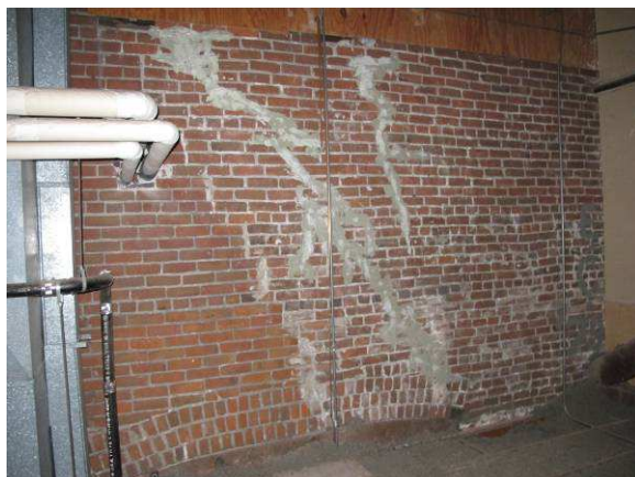
Brick repairs at north end roof
