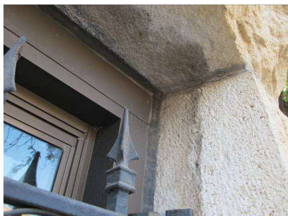
Failing sealant
