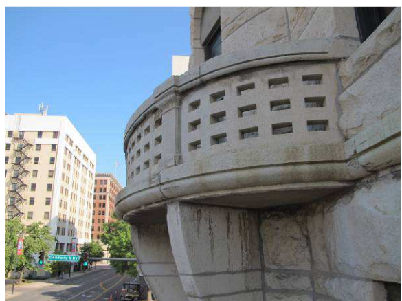
Deteriorating mortar
