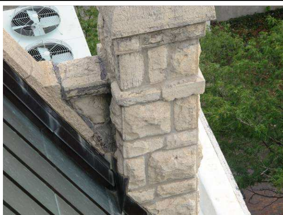
Failed mortar
