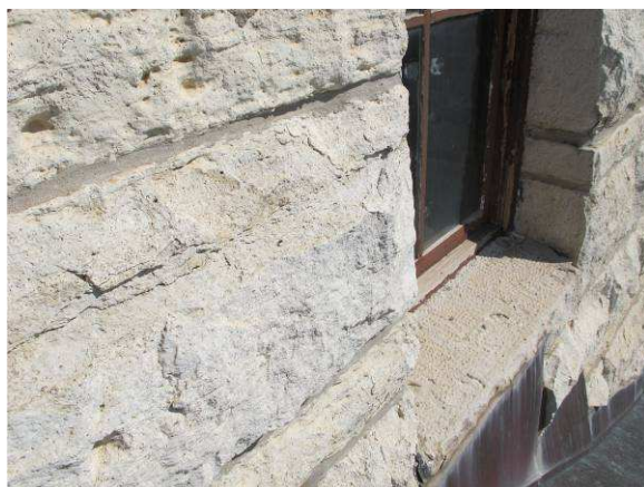
Deteriorating limestone
