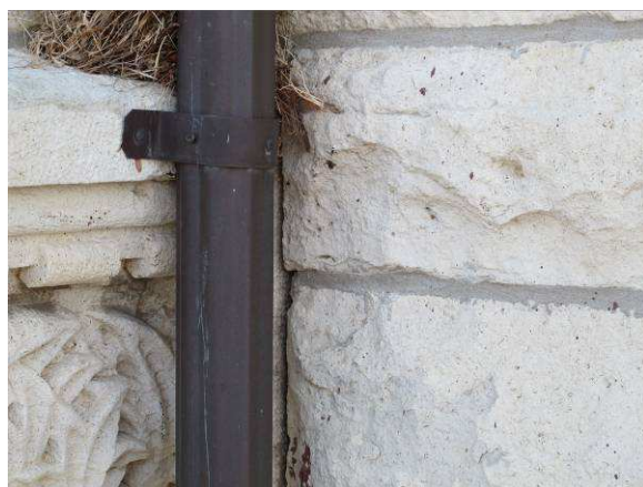
Missing mortar
