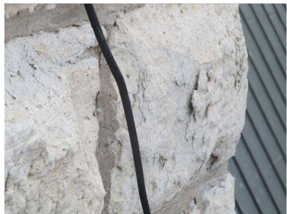
Spalling stone
