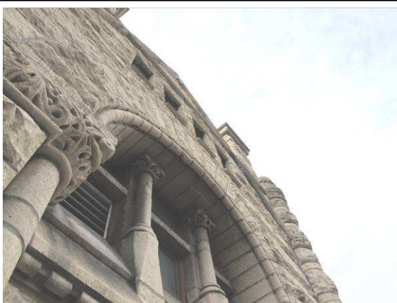
Underside of arch
