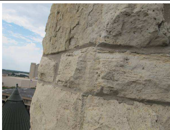
Deteriorating stone
