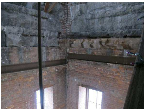
Metal and wood beams
