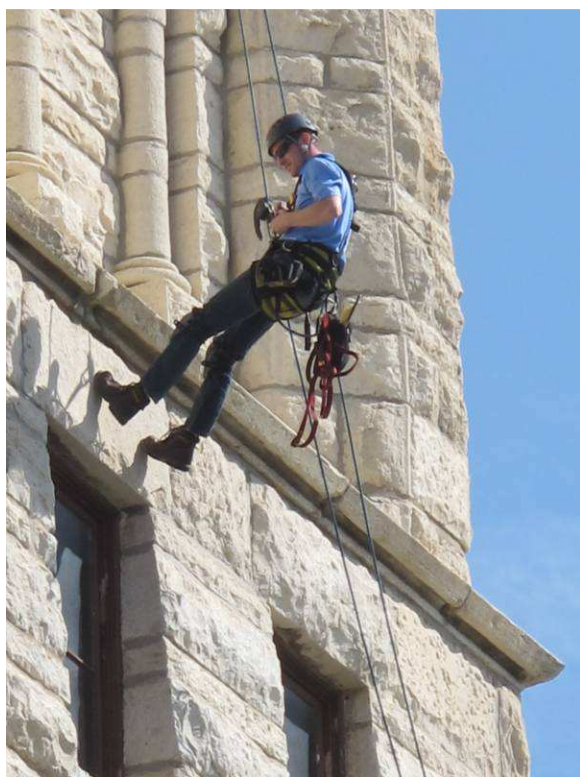
Assessment ongoing on south face
