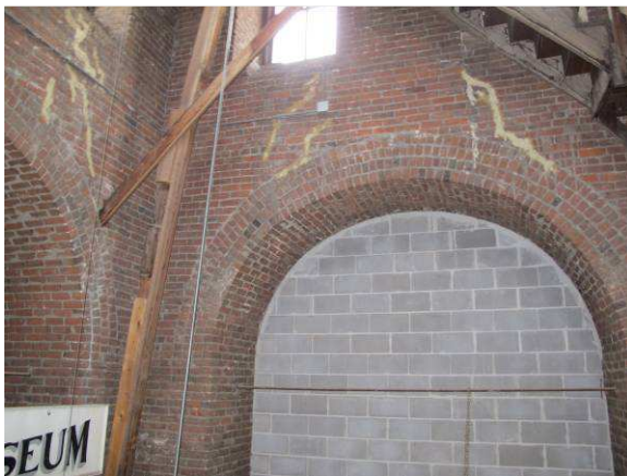
Repaired cracks above arch
