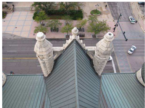
View of back of perimeter stone
