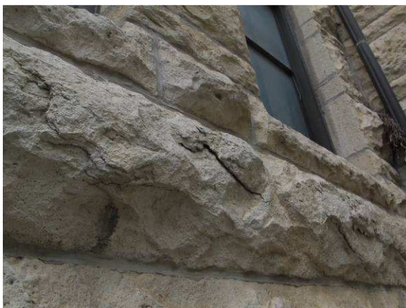
Spalling stone
