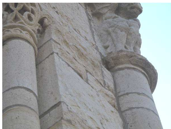
Deteriorating limestone
