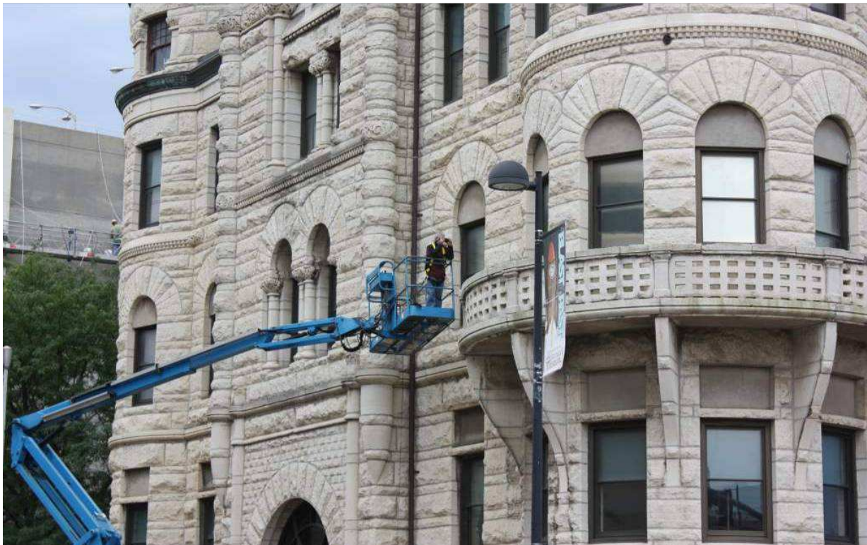
Assessing the northwest corner balcony from the 60' articulating lift
