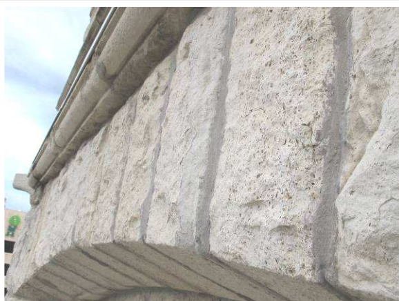
Loss of detail above arch
