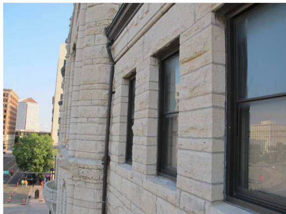
West side of the building
