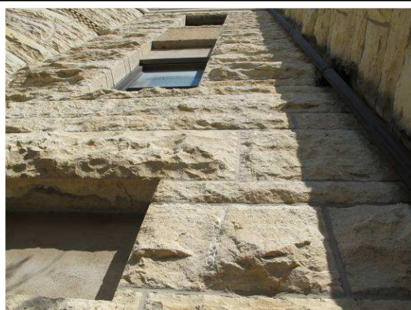
Mix of infilled and glazed windows
