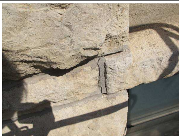
Separated mortar
