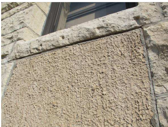
Cement board infill at windows
