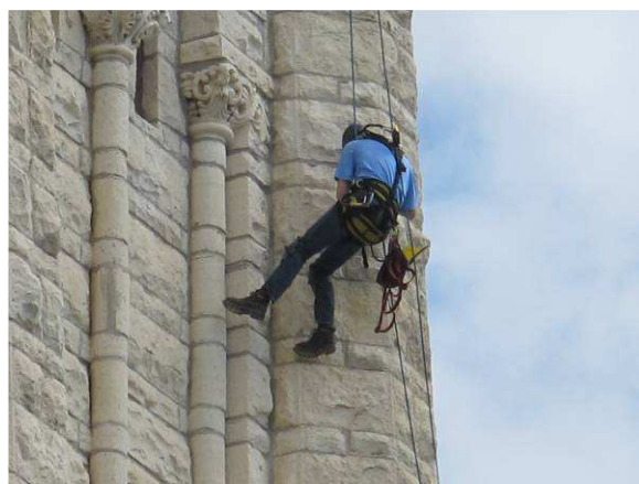
Close up showing rappelling system
