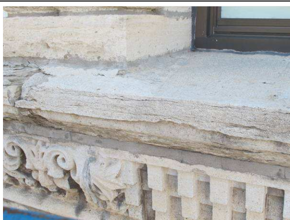
Damaged stone
