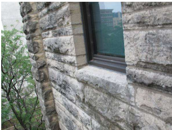
Deposition on limestone
