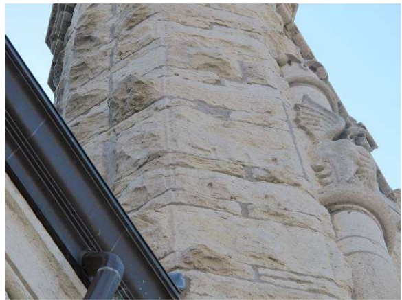
Deteriorating stone
