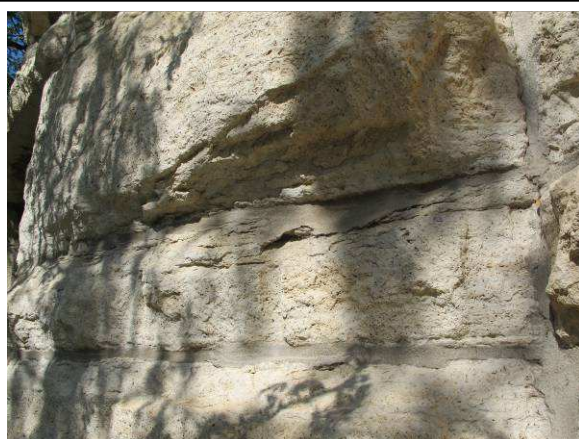
Deteriorating limestone
