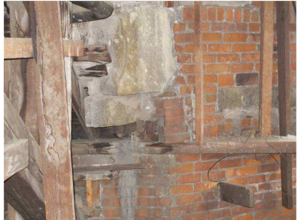
Uncoursed mix of brick and limestone
