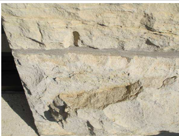
Spalled stone
