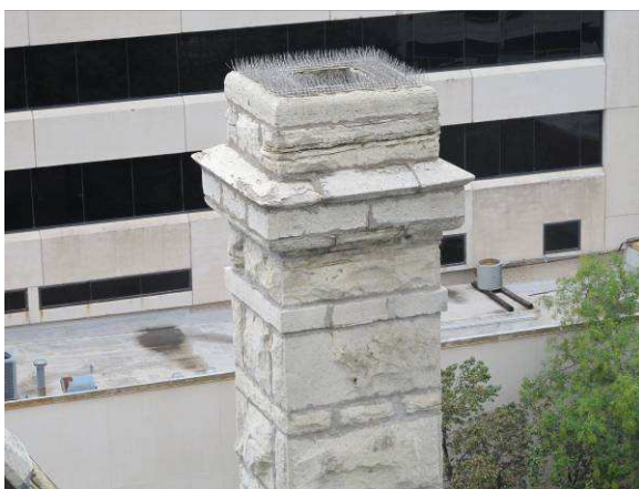
Chimney at NE corner
