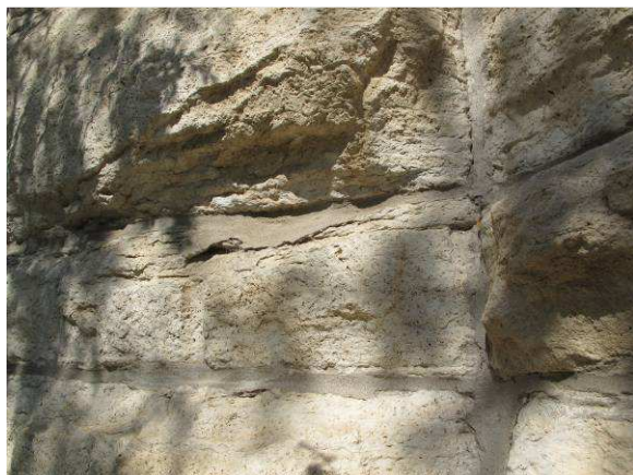
Deteriorating limestone
