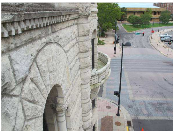
North side of bldg looking west
