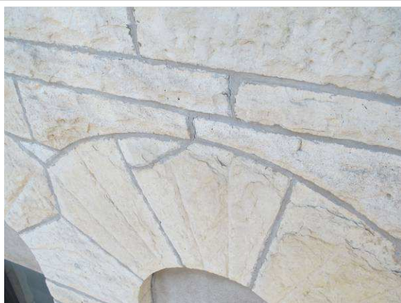
Repaired cracked stone
