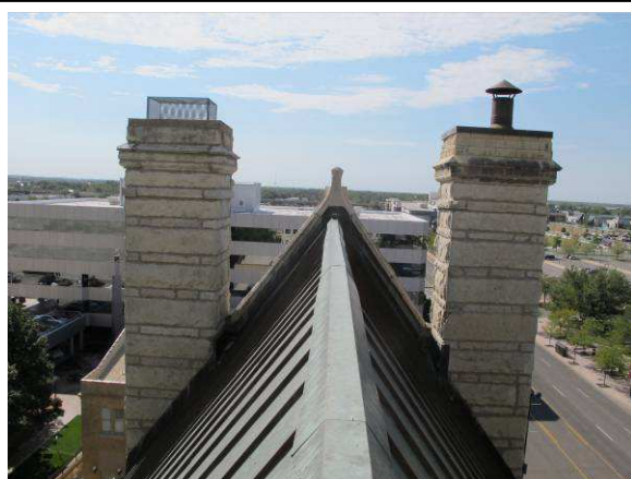
Back of south side chimneys
