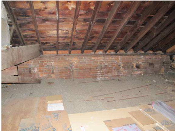
Interior brick wythes and seated ceiling rafters
