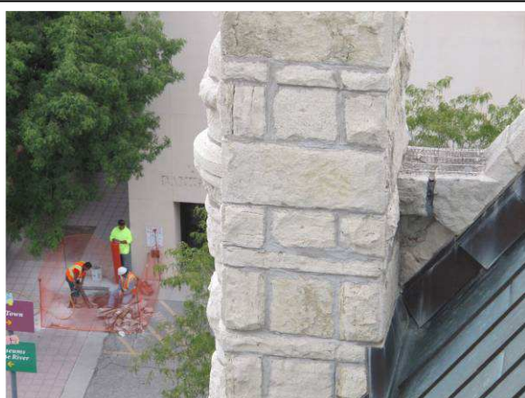
Chimney at NW corner
