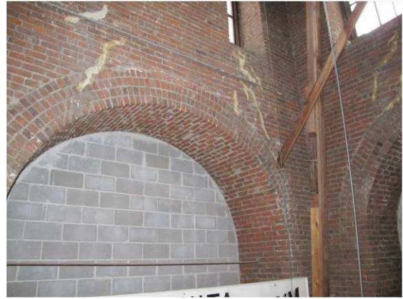
Repaired cracks above arch
