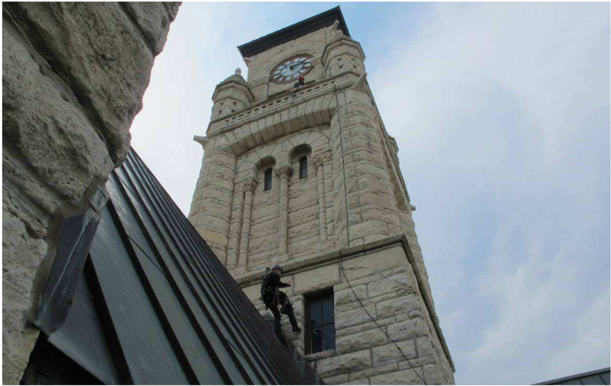
Completing the assessment on the east face of the tower
