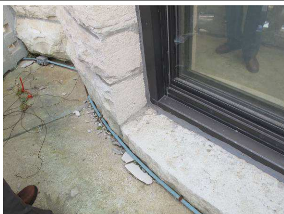
Deteriorated stone
