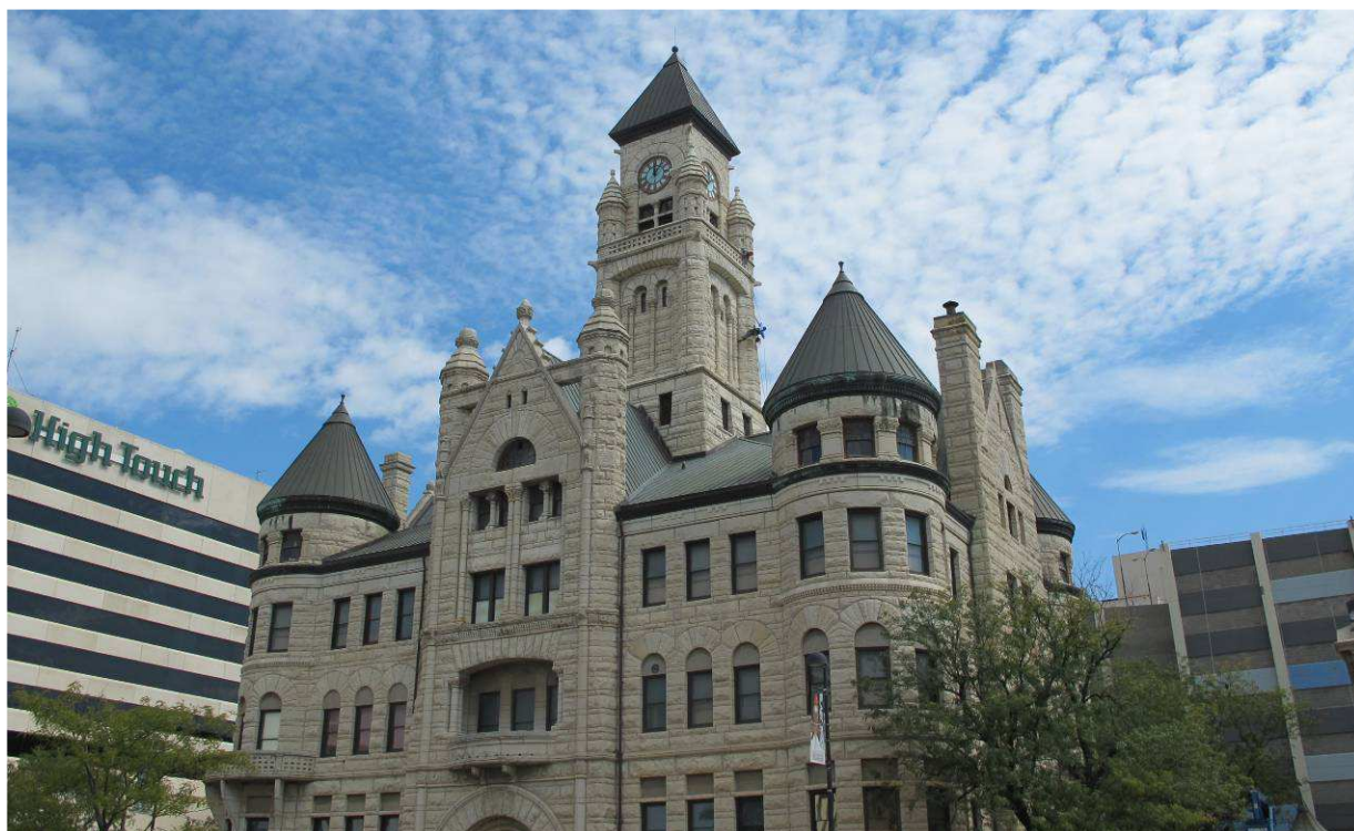
2 nd drop assessment underway on south face of clock tower
