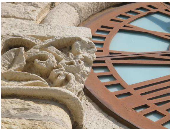
Loss of carving detail in stone
