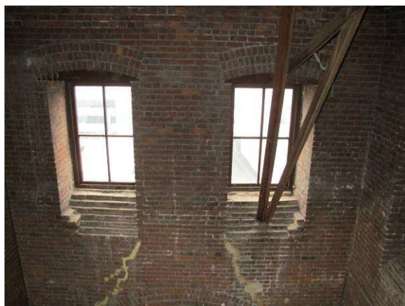
Repaired cracks from above
