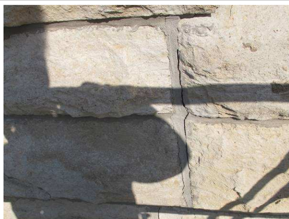
Separated mortar
