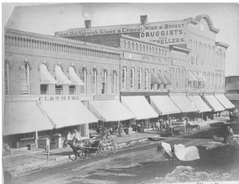
Figure 11. The three-story Phoenix Blocks ( upper right ) "rose from the ashes" of the 1871 fire that destroyed three buildings on the northeast corner of Main and 2nd streets. This block of Main Street was the first to be lined with all masonry buildings, all of which are extant, although variously altered. Source: Cedar Falls Historical Society/UNI Historical Cedar Falls website
