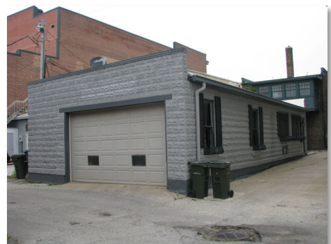
Figure 35. Concrete block storage building (Map #44), built to be Gram Plumbing Shop in 1912, quite possibly made use of Weart-Frisby’s locally produced rough-faced cement blocks. Photo by Jennifer A. Price, October 2014
