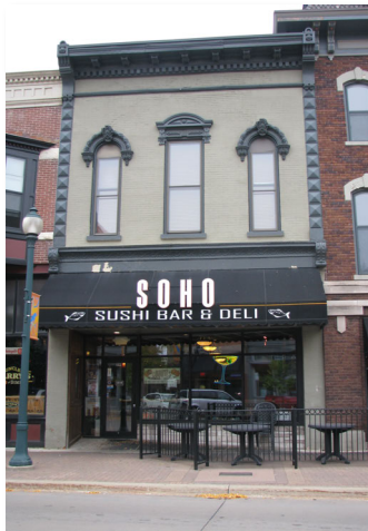
Figure 36. The cast iron storefront components on the upper floor of the Townsend & Knapp Bank Block, built 1870, include its window hoods and prominent bracketed cornice. Photo by Jennifer A. Price, October 2014
