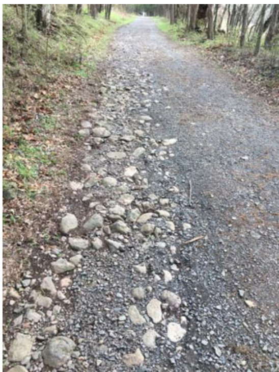
Rock Road looking south from Bladen's farm lane intersection.
