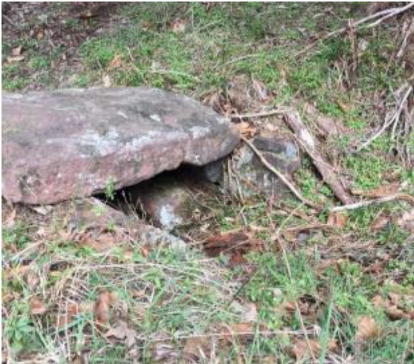
Red sandstone culvert at the base of Bladen's farm lane.
