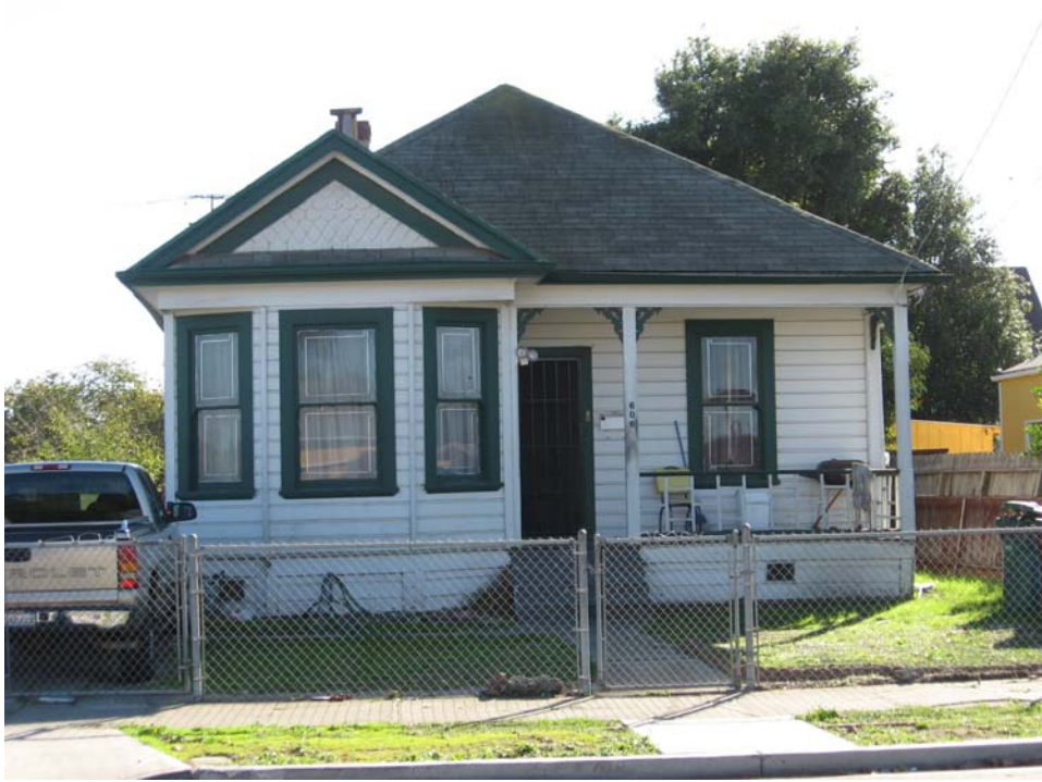
606 Maine Avenue (1905) is an example of a property that appears to be individually eligible for the California Register. It retains nearly all of its original materials and decorative details, such as the scrolled porch brackets, and is an excellent example of a modest Queen Anne style cottage (Page & Turnbull).
