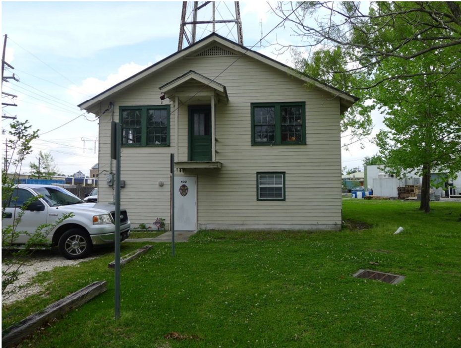
South West Facade
