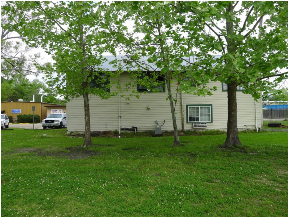
South East Facade
