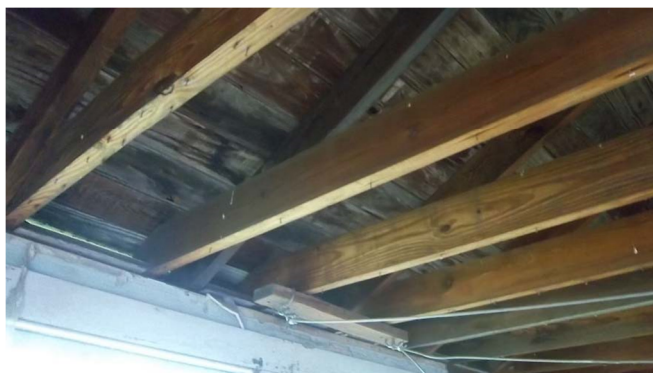
Wood rafters and plank wood roof deck
