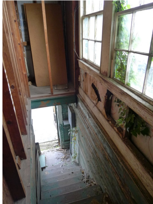
The exterior door to the second floor is boarded up and beyond repair
