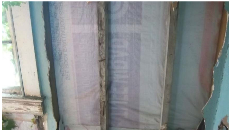
House wrap between studs and rigid foam board
