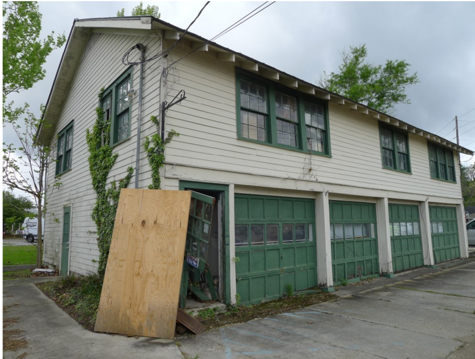
North West Facade
