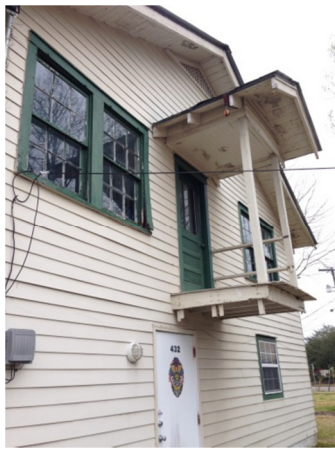
Cantilevered porch to former exterior stair
