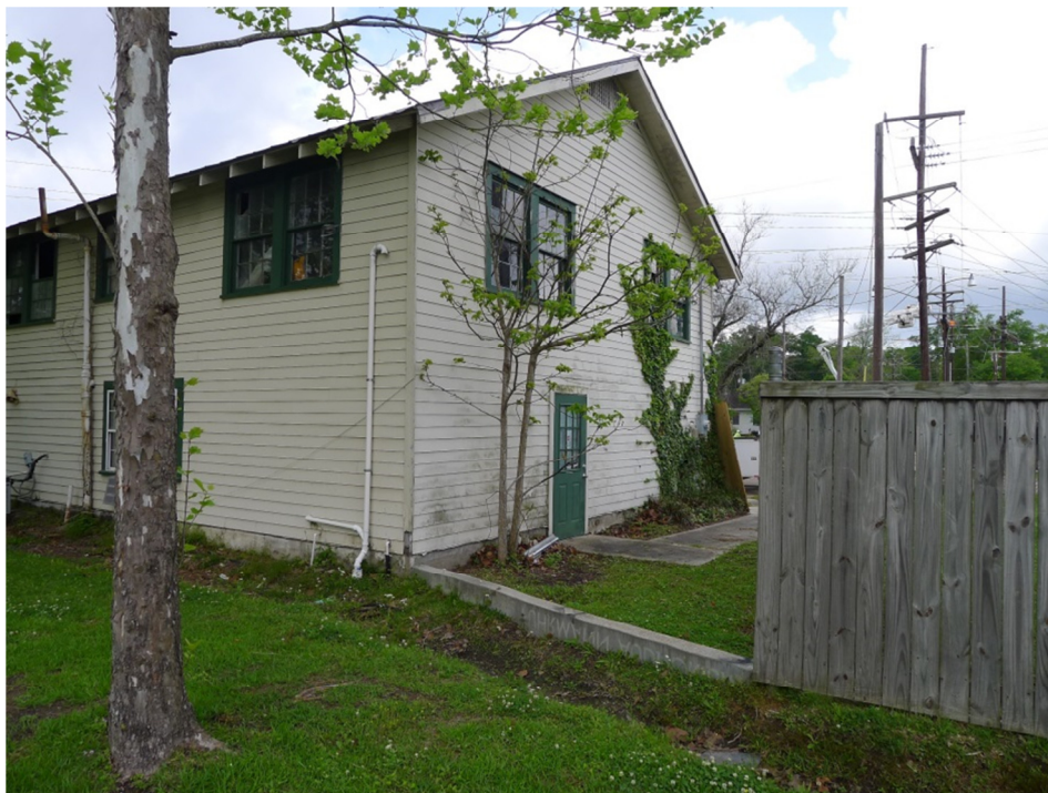
North East Facade
