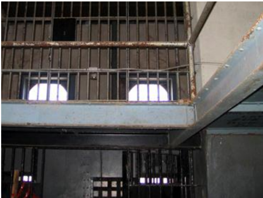
Photo: Steel and masonry interior structure framing the open, central gallows tower, which could include a lift, “Llano County Red Top Jail of 1895, Llano, Texas, Preservation Master Plan”
