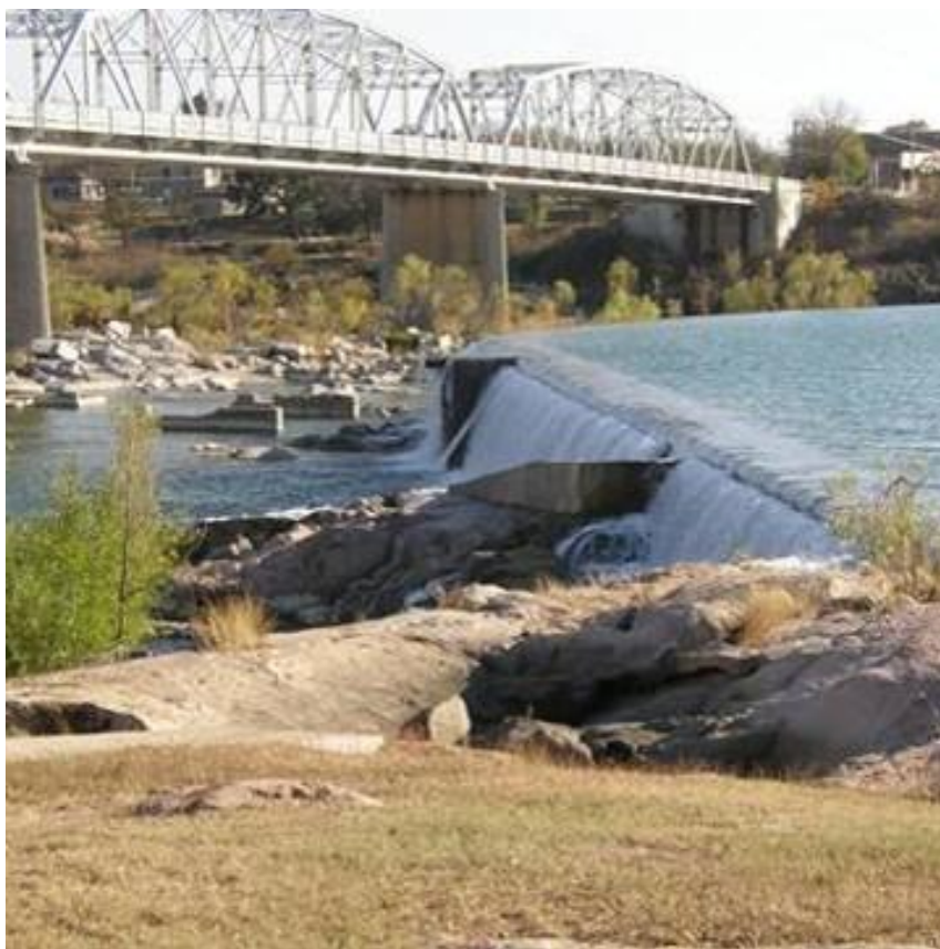
1935 Roy Inks Bridge and Dam, photo courtesy www.texasescapes.com
