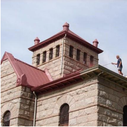
Red Top roof repairs June 2009
