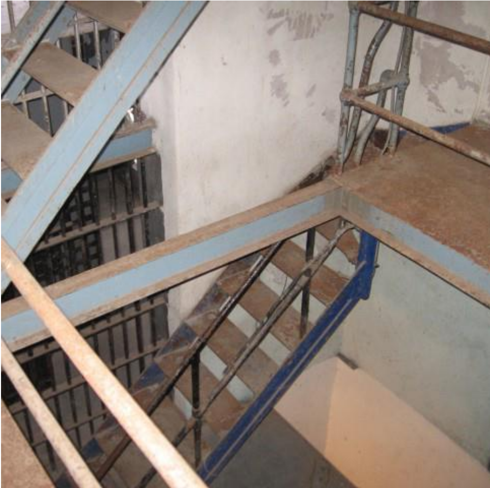
Photo: Central shaft of gallows tower and stairwell, "Llano County Red Top Jail of 1895, Llano, Texas, Preservation Master Plan"
