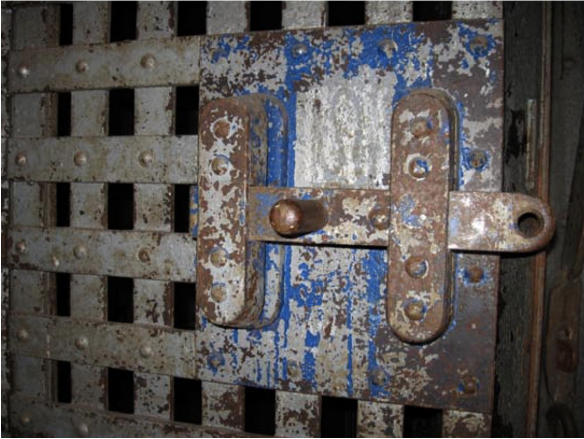
Photo: Cell locking system, “Llano County Red Top Jail of 1895, Llano, Texas, Preservation Master Plan”
