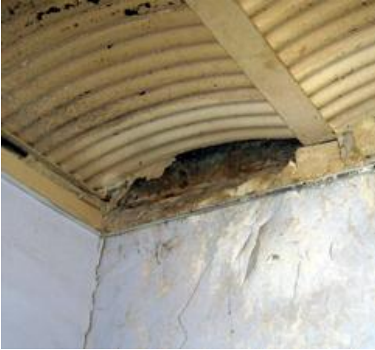
Photo: Corrugated metal vaulted ceiling and I-beams, "Llano County Red Top Jail of 1895, Llano Texas, Preservation Master Plan"
