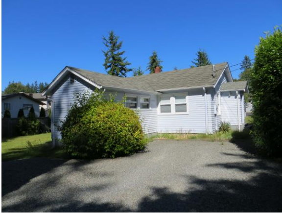
oblique view of east and north facades 2015
