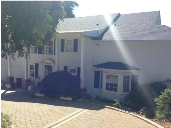
oblique view of north facade 2015
