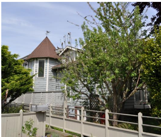
west facade and turret detail 2015
