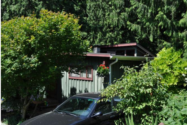
oblique view of south-east corner 2015
