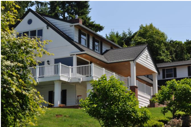
oblique view of north and west facades 2015
