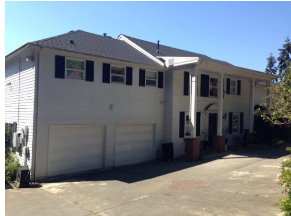
oblique view of north facade 2015
