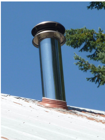
Main Hall Chimney
