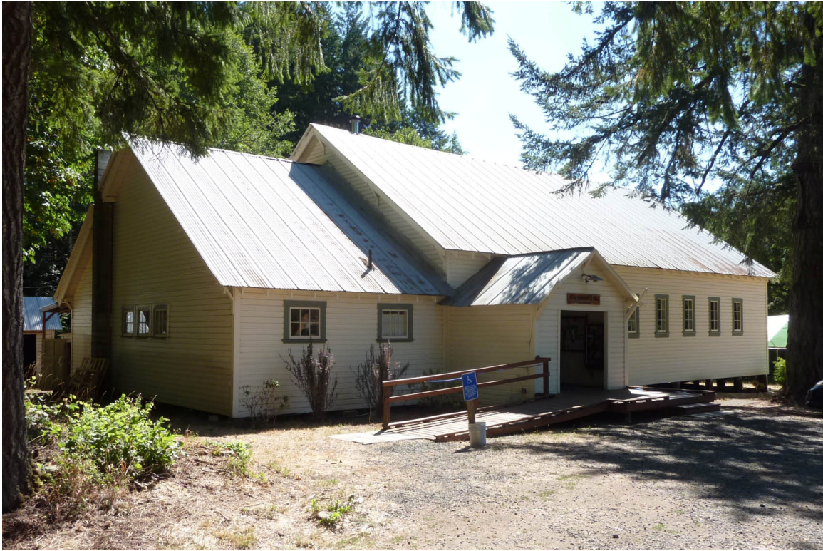
North and West (Front) Elevations
