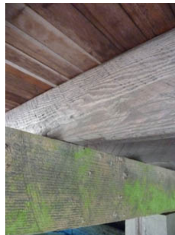
Flooring, Joist, Beam
