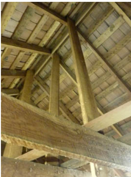
Attic Framing at Addition
