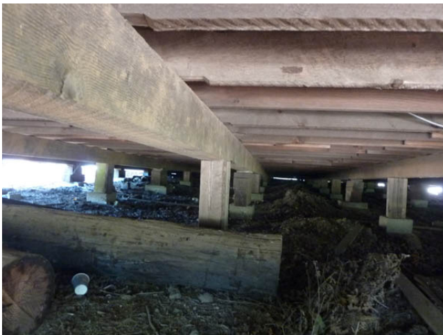
Main Floor Framing; Joists Interior Beam and Posts
