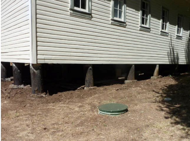
Main Floor South and East Posts, Septic in Foreground
