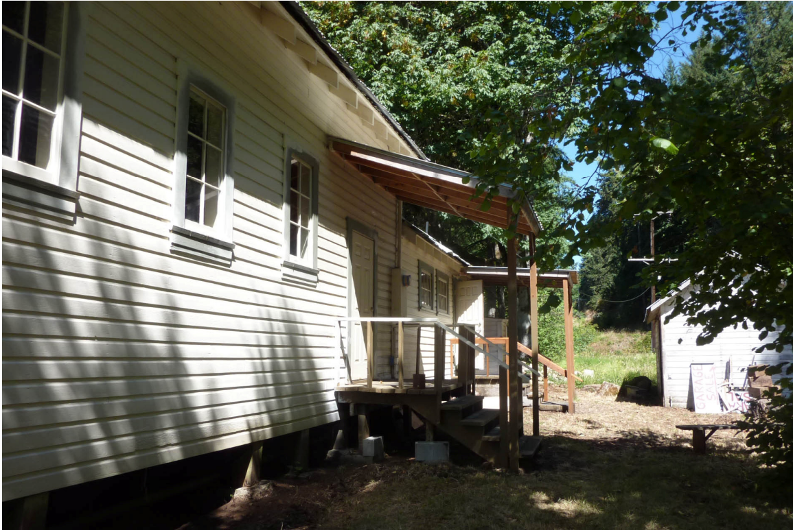
North End of East (Rear) Elevation, Woodshed on Right
