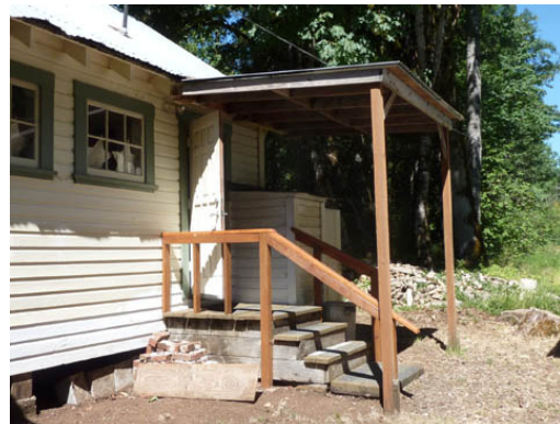
Porch and Roof at North
